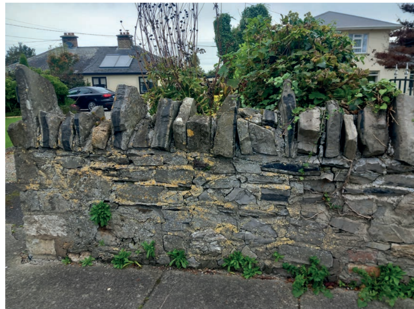
Figure 7.14: Rubble limestone wall with fieldstone cappings on Knockmeenagh Road.
