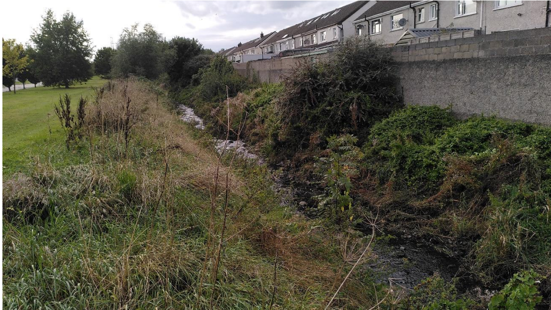
Figure 4-5: Downstream section of Whitestown Stream.
