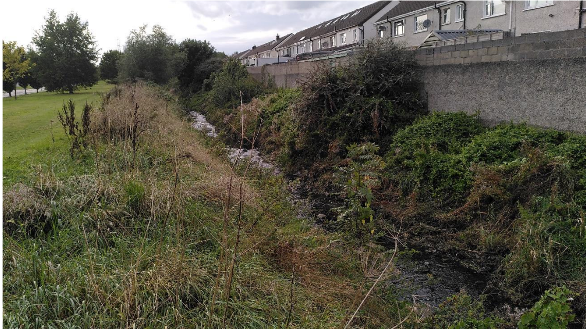
Figure 3-3: Downstream section of Whitestown Stream.
