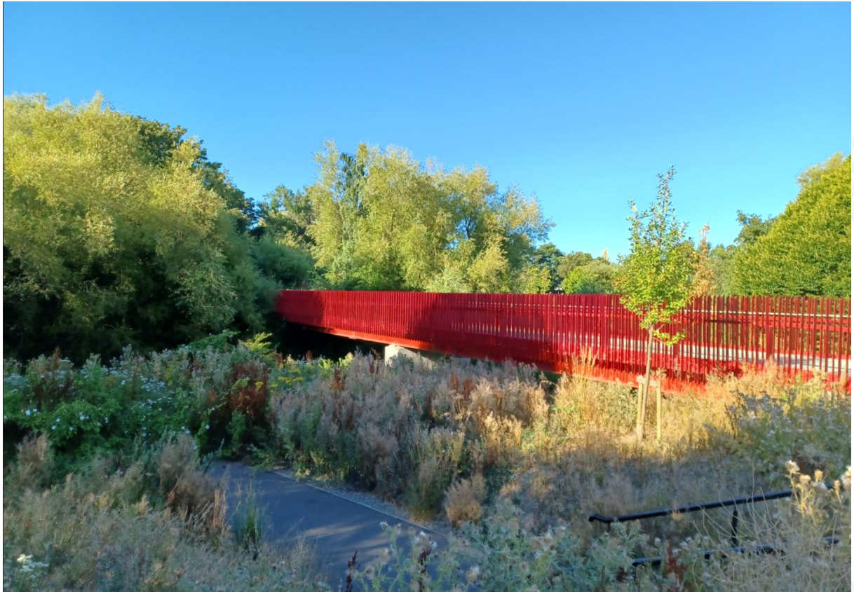
Figure 2-5: Proposed Bridge Design Precedent - Steel Through-Truss Arrangement Supported on Concrete Abutments (Source: Arup)
