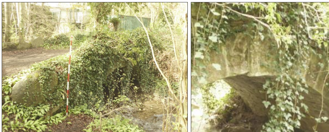
Plate 10 Downstream side of the bridge Plate 11 Detail of the quarry-faced keystones
