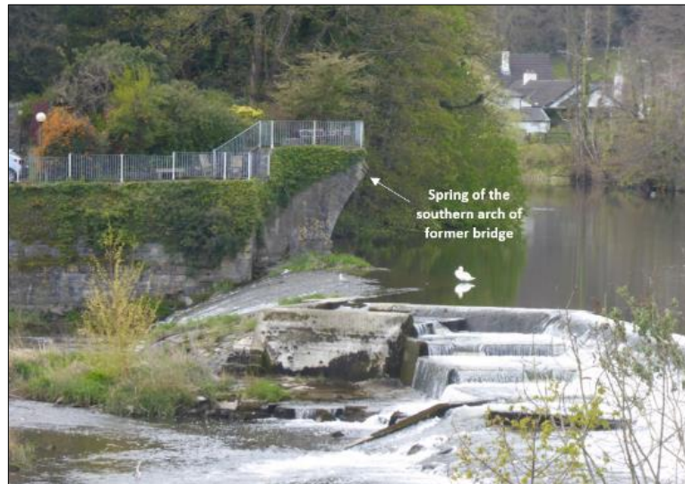
Plate 4 View of the remnants of the former bridge
