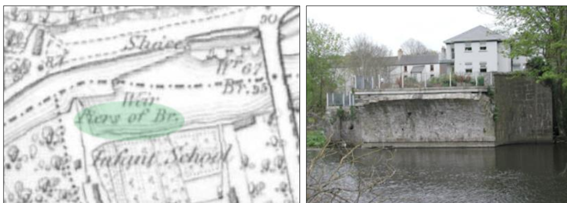
Figure 10 First edition OS Map 1836-37 and a view of the surviving spring arch of the 'Coldblow Bridge'.
