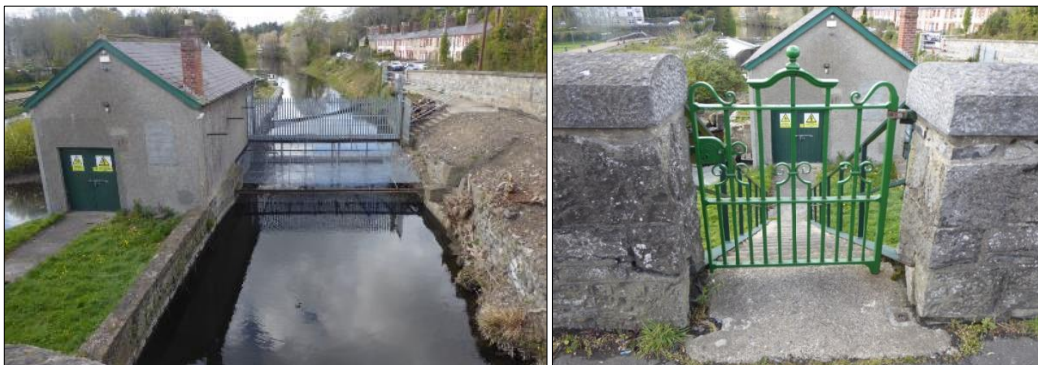
Plate 5 Turbine House and mill race Plate 6 Stairs leading to the turbine house
