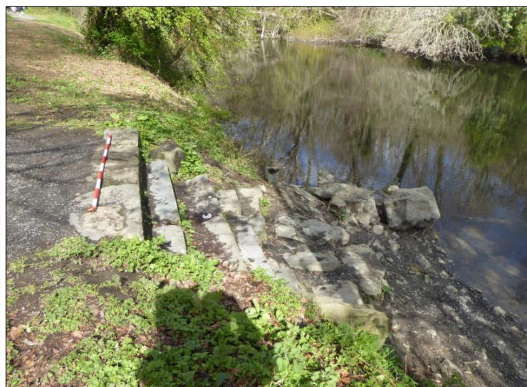
Plate 12 Steps to the river (CH5)
