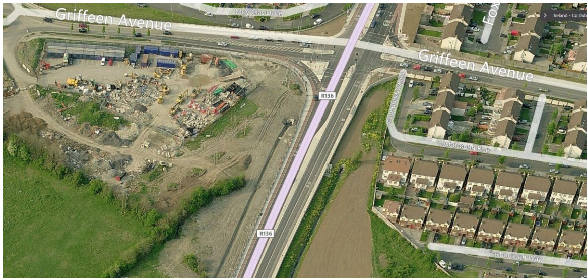
Figure 2-4: Existing Outfalls either side of the Outer Ring Road
