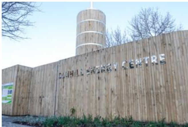
Figure 24: Bunhill Energy Centre in Islington, London 24
