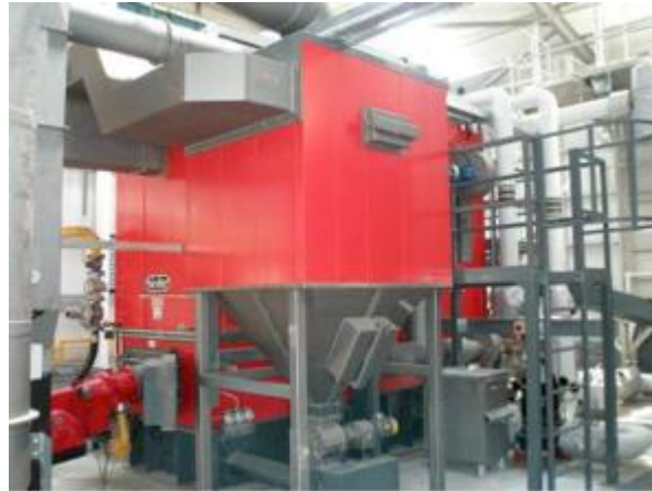
Figure 16: Example Biomass boiler: Binder biomass boiler (from the 500 kW-10 MW range) 16 .
