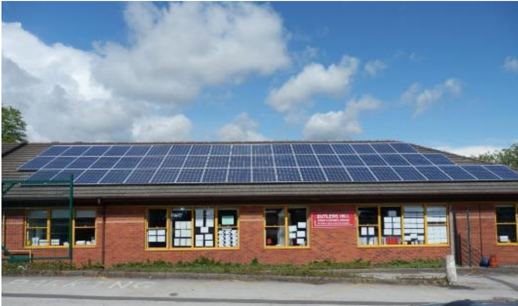
Figure 68: 45 kW solar PV panels installed at Butlers Hill Infant & Nursery school, Nottingham in 2014 38
