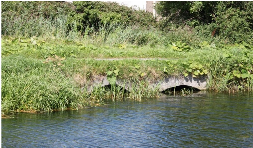
Photo 15: 12th Lock Millrace Cut Stone Arches
