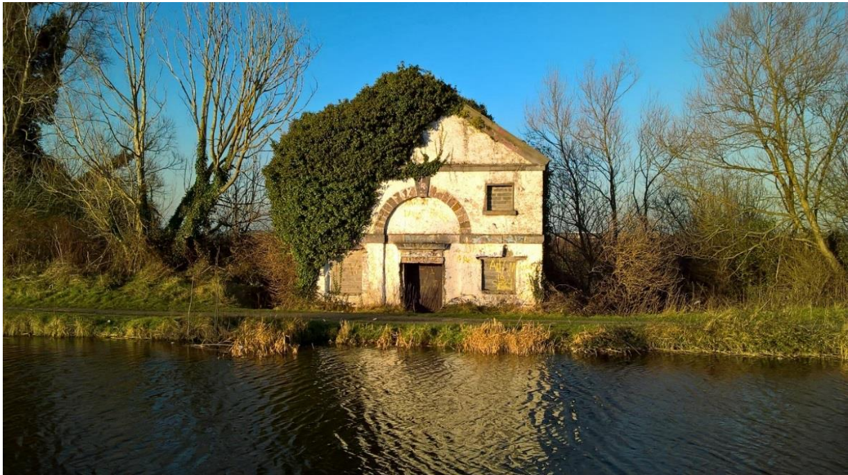
Photo 10: Omer's Lock House at 11 th Lock
