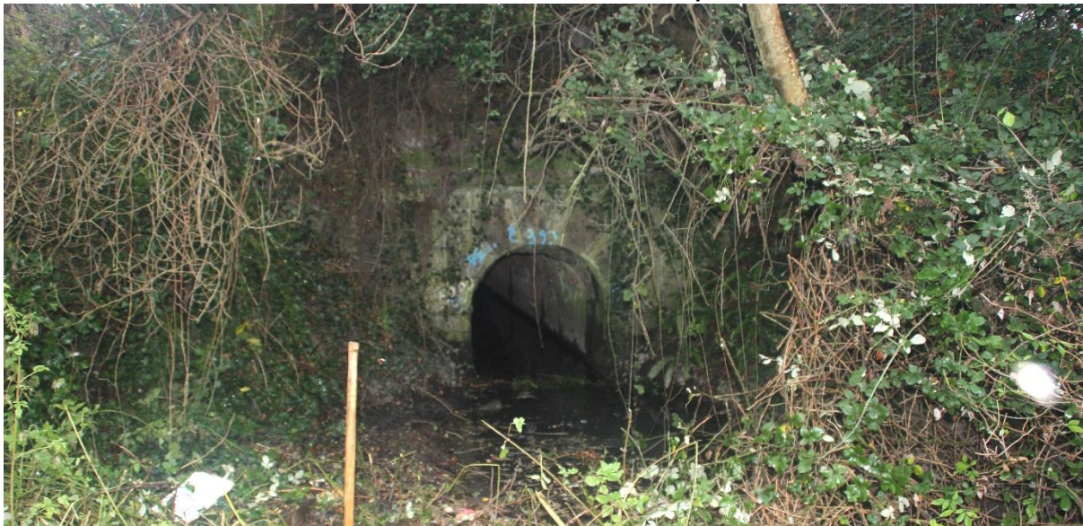
Photo 12: Kilmahuddrick Stream Aqueduct
