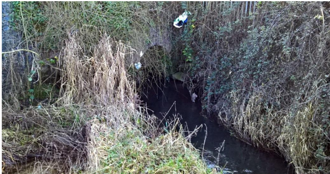
Photo 11: Griffeen River Double Arched Aqueduct
