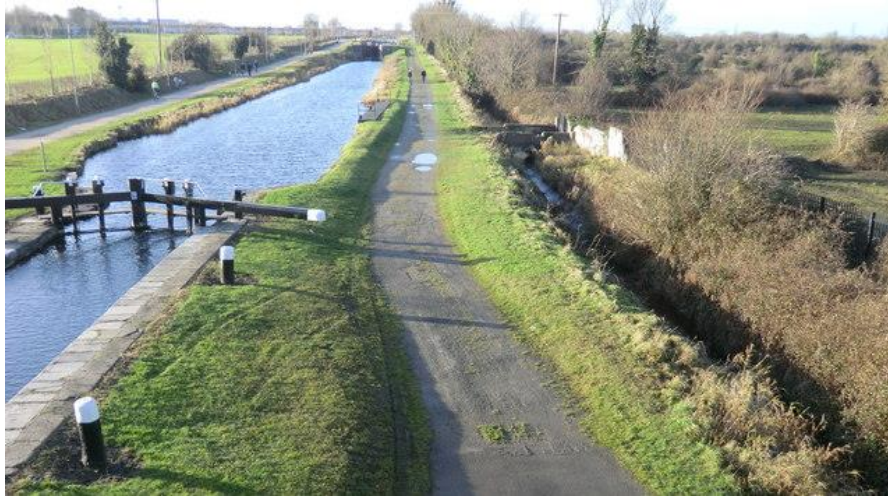
Photo 16: Cappagh Overflow and Bridge adjacent to 10 th Lock
