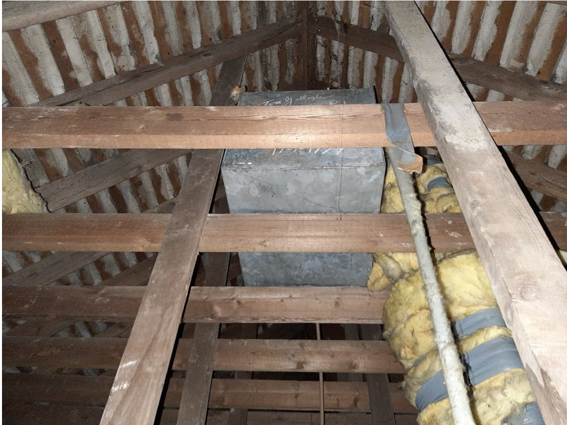
Figure 17 - Roof and galvanised steel water tank (for further details refer to Appendix 2)
