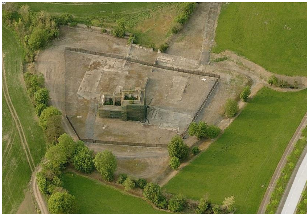
Fig.1. An aerial view of the proposed development site from the south. (Source: Image from the website “bingmaps.com” on 7/11/2016)
