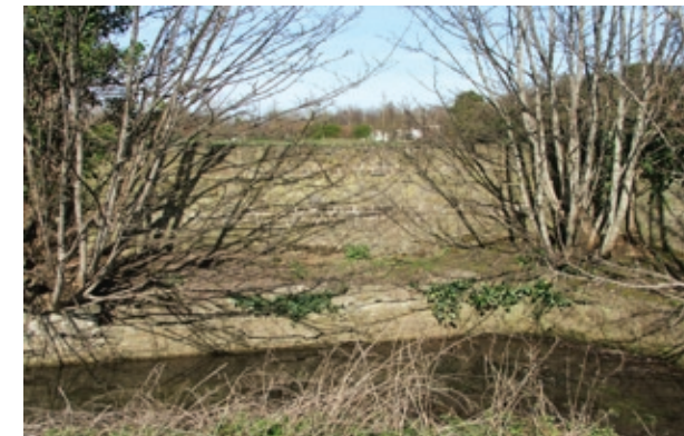
4. Stone Wall Boundary to North of Site
