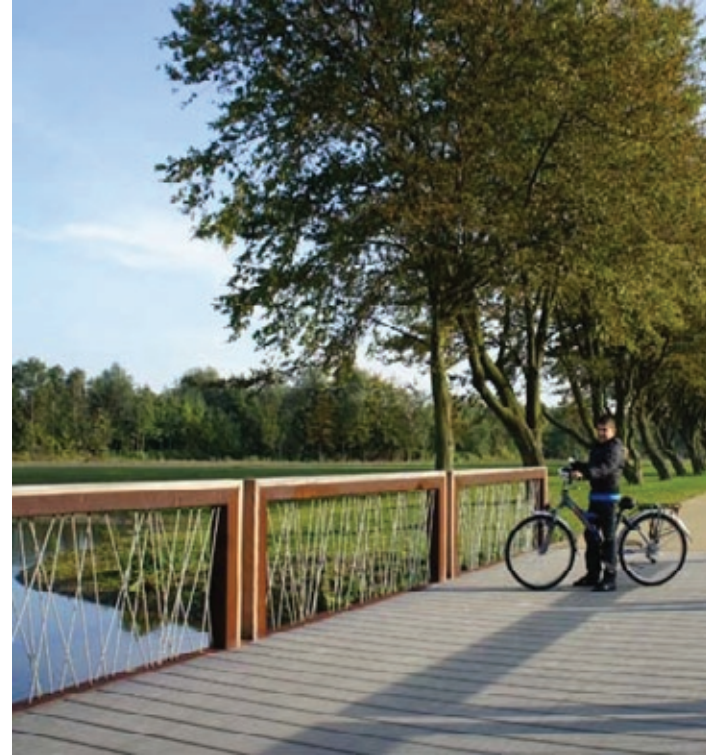
Corten Steel Bridge
