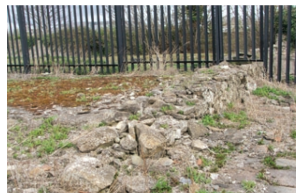
7. Foundations of former Buildings (1900-1910)
