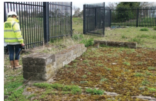
5. Foundations of former Building (1800-1910)
