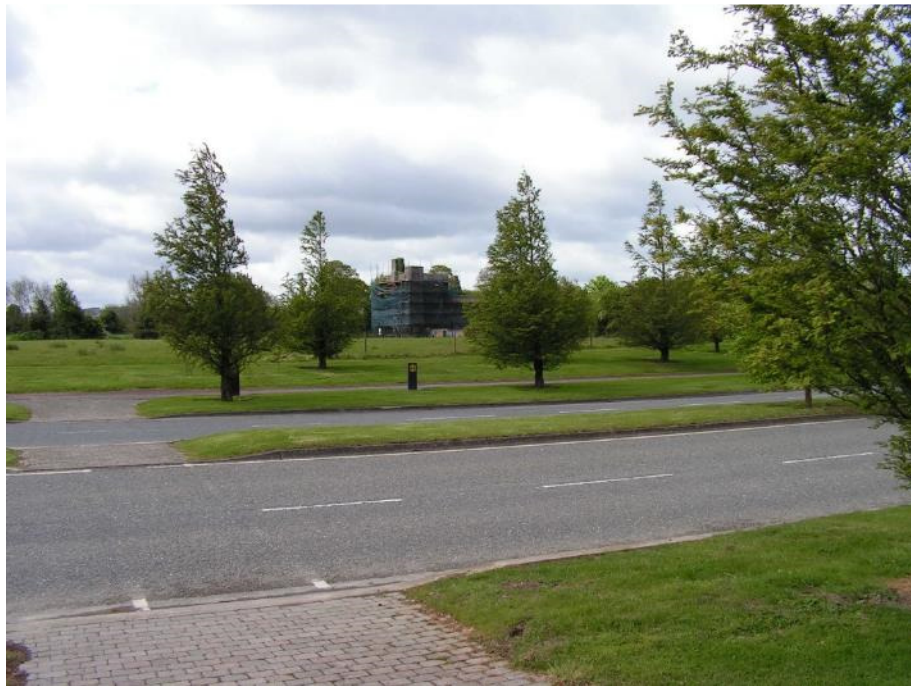
View of the castle from the north (May 2015)
