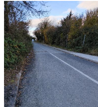
Existing Old Nangoor Road
