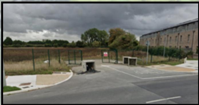
Spur into lands already built as part of Celbridge Link Road
