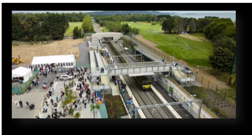
Image above: Aerial photograph of the completed and operational Woodbrook Dart Station. (Source: Google Images.)
