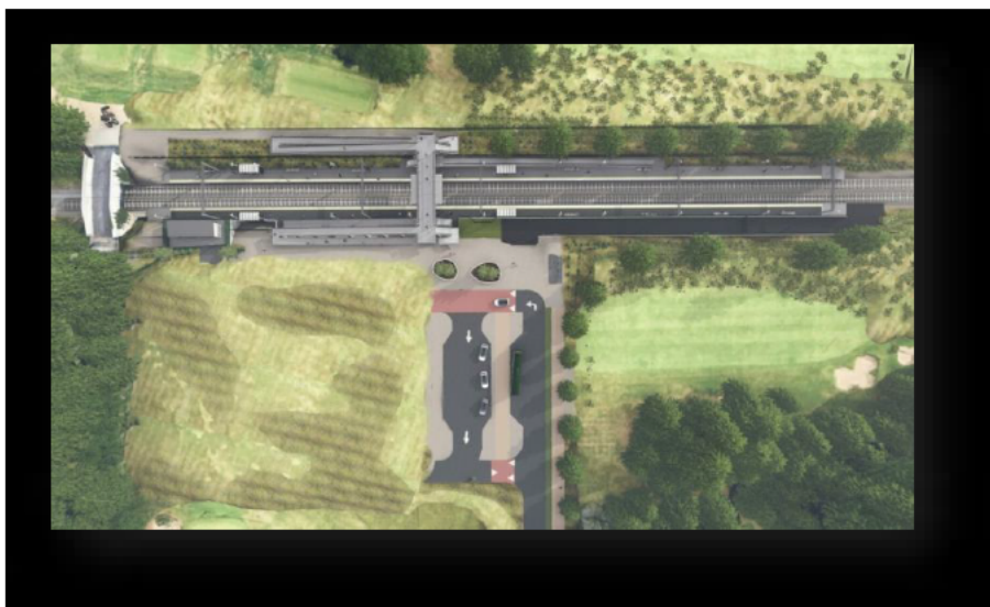
Image above: Plan view of the now built and operational Woodbrook Dart Station. (Source: Irish Rail.)
