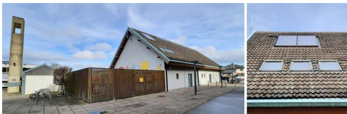
Fig. 2.13: Image Left - View of the Ballyroan Community & Youth Centre, with screened external children's play area and the boiler house with chimney stack, taken from the southwest looking northeast. Image Right - Detail of the solar panels and roof lights to the south facing pitched roof.
