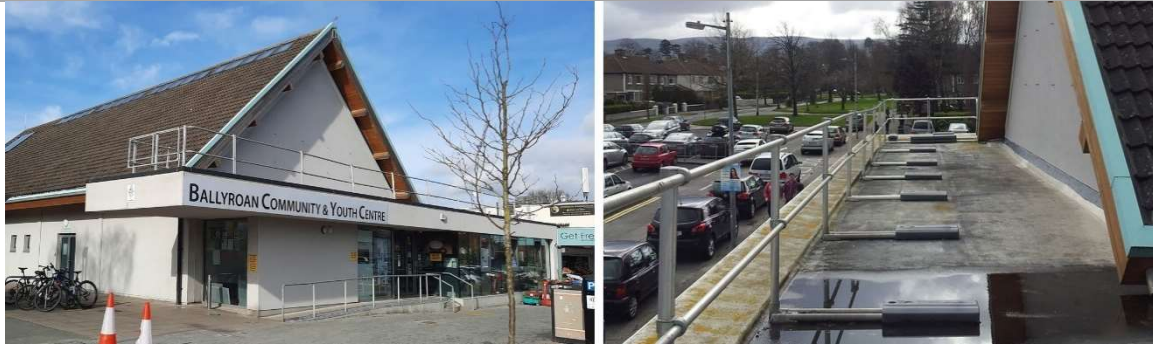
Fig. 2.14: View of Ballyroan Community Youth Centre front elevation, with safe access guarding to single storey flat roof (left). Close up image of the ballasted guardrail system (right)
