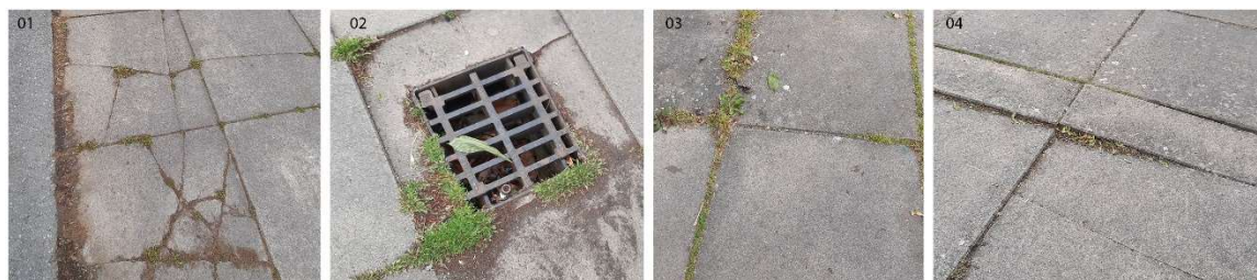
Fig. 2.18: Site photographs taken in May 2025, indicating selection of cracked, subsided and lifted pavers
