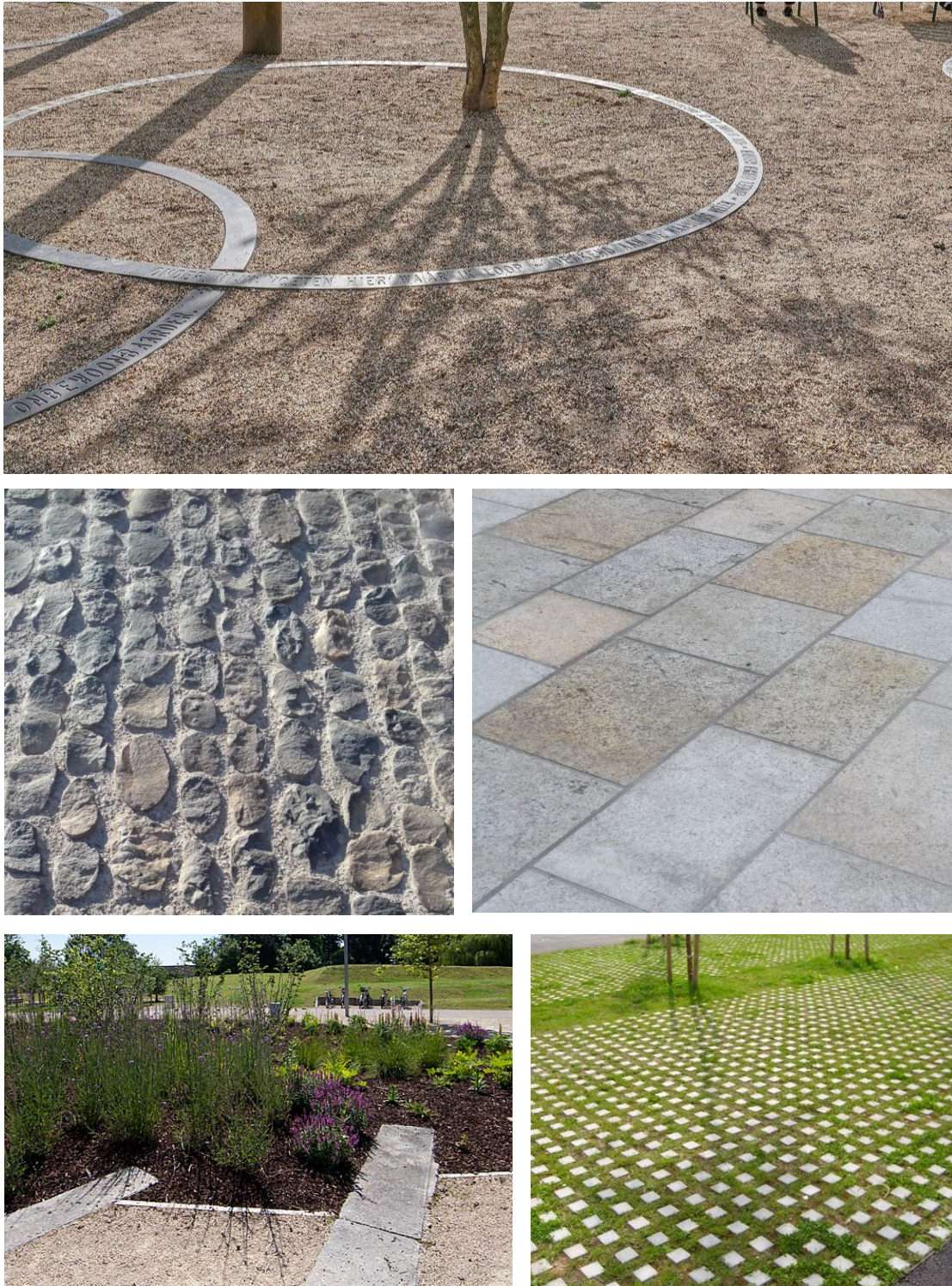
Fig 19: Typical Materials Proposed, clockwise from top left: Self-Binding Gravel; Natural Stone Paving; Reinforced Grass; Occasional use of natural stone elements within gravel; Reuse of existing cobble from site
