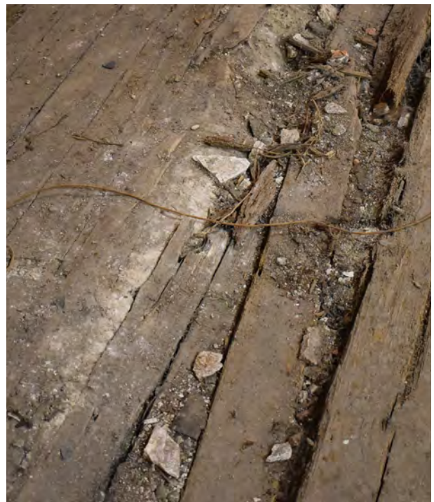
Damage to floorboards in north-west corner of Room 1 above likely service route to nearby radiators.
