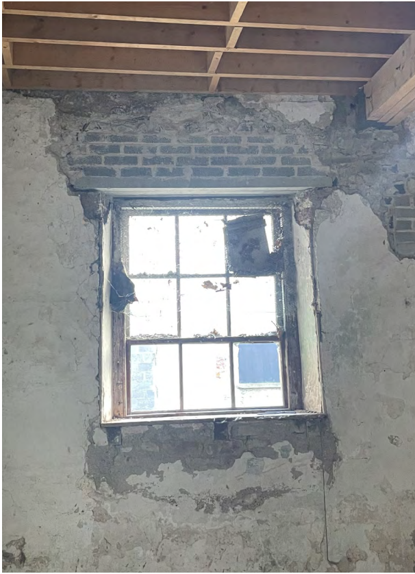
6 over 3 timber sash window in room 2.7. Records from 2018 works report this window to be fitted with a hinge allowing the sash to pivot open.
