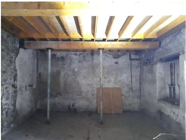
Fig 4.2.4 Back propping to Mezzanine Beam noted photo HHC
