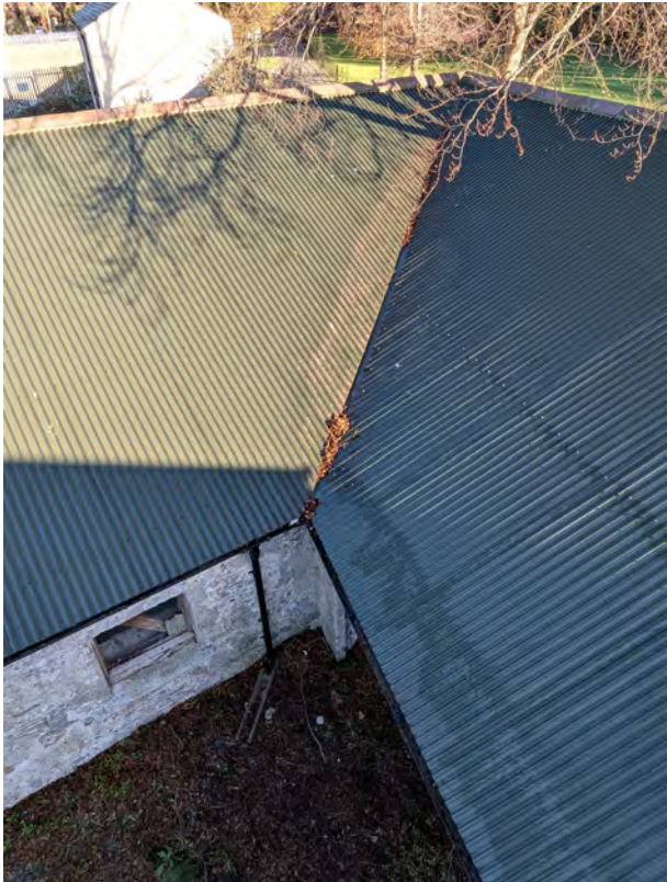
Due to the presence of an adjacent mature tree, Building 3 is prone to a build-up of heavy leaf fall within the valley gutter and at the drainage channel at the base of the downpipe.
