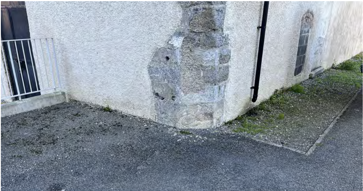
Cracks visible in plasterwork to North-West corner where edge of gully meets corner of wall.
