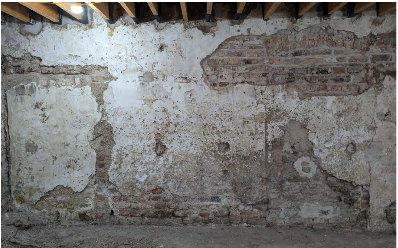
Previous openings in wall between 2.2 and 2.3 partially visible, infilled with brickwork and finished with lime plaster.
