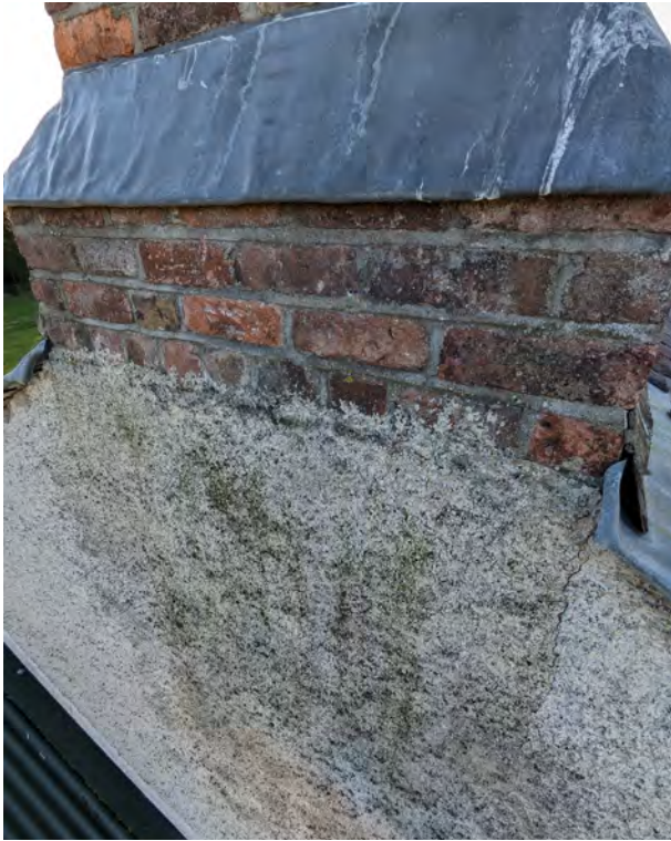
Plasterwork of the northern gable wall discoloured due to damp staining beneath the chimney stack.
