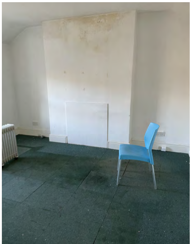
Discolouration to top of chimney breast, first floor, north room.
