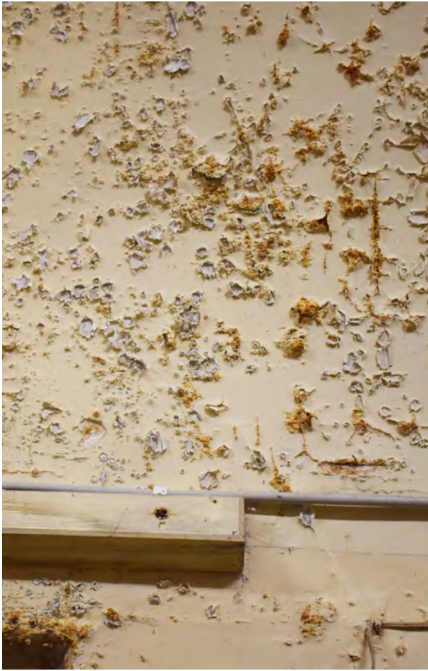
Extensive damage to paintwork throughout, including peeling and growth to walls indicating dampness internally.
