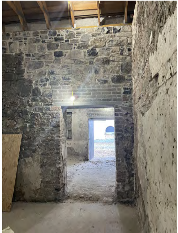
Recently installed concrete lintol, concrete blockwork and stonework to opening between 2.1 and 2.3.
