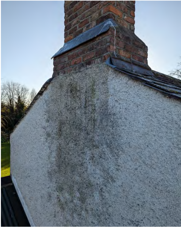
Damp staining to north facing gable.
