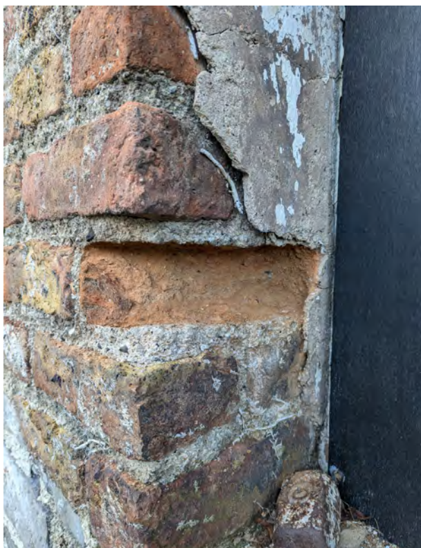
Damage to brickwork and loose plaster to window reveal.
