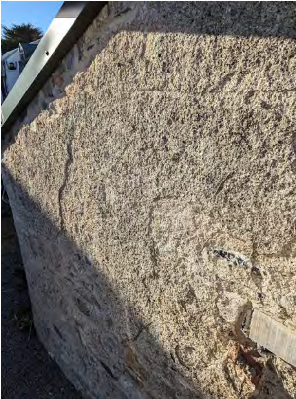
Lime render partially remains on the east facing gable, but shows signs of spalling and crumbles to touch.
