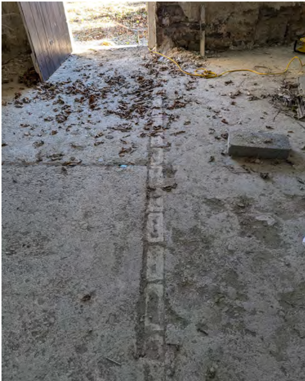
Concrete floor with brick channel detail (Room 2.1)
