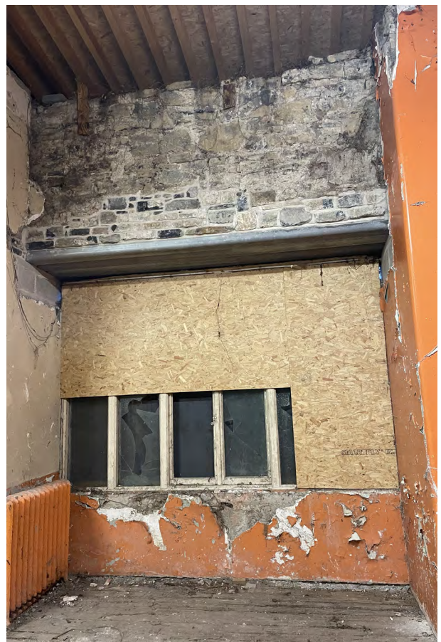
Ope 10: Timber framed window partially concealed with plywood. Damage to glazing. A concrete lintol has been recently installed.
