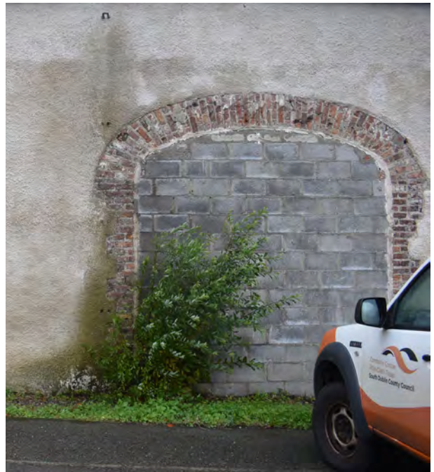
Ope 1, blockwork infill to brick carriageway arch.
