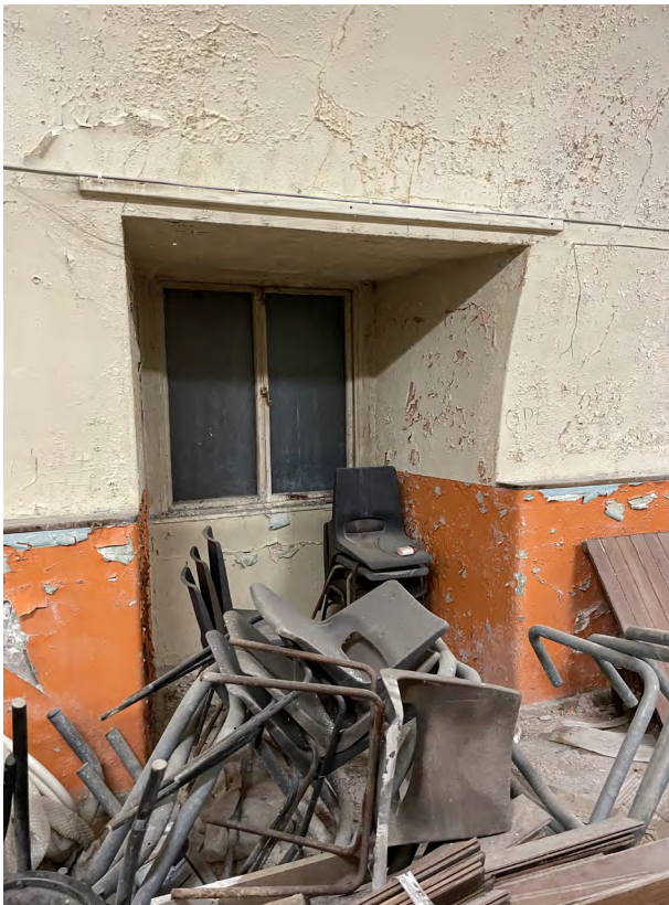
Ope 8: Timber framed window, opaque glass.
