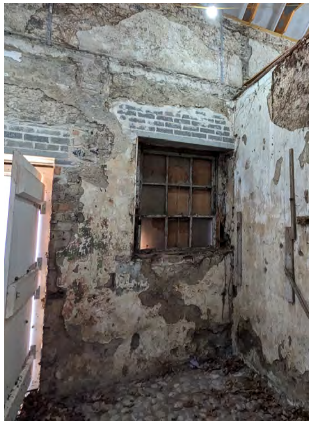
6 over 3 timber sliding sash window in room 2.6. Concrete lintol and blockwork over. Glass panes broken or missing.
