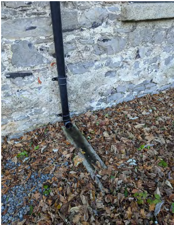
Downpipe at east facade (courtyard 1) discharging into concrete channel, directed away from base of wall.
