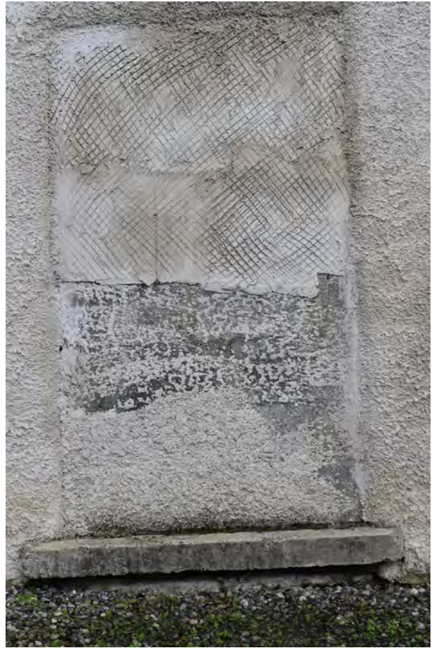
Ope 12, blockwork infil, partially rendered. Concrete cill.
