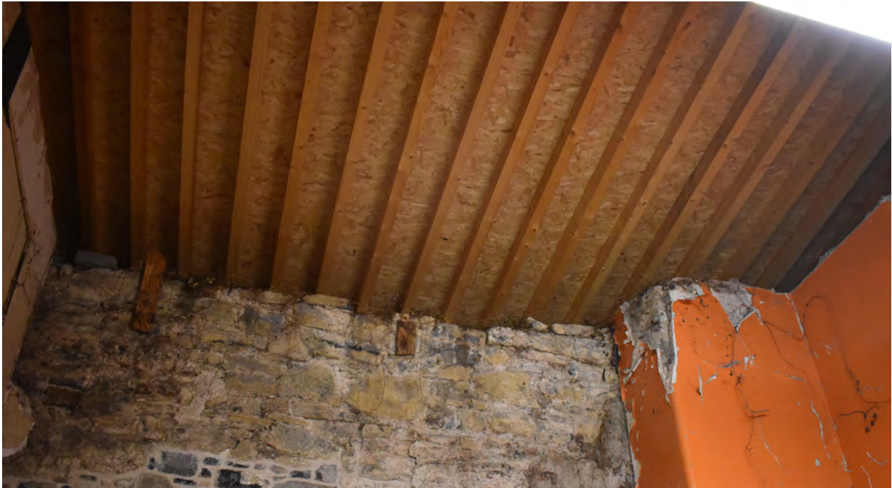
Modern timber roof structure and roof deck visible.
