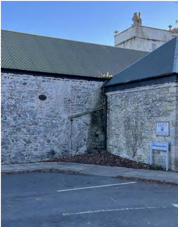
Downpipe to north-west corner discharging from valley gutter. Vegetation growth within gutter and staining to adjacent wall indicating saturation due to overflowing discharge. Leaf build up at base of downpipe.
