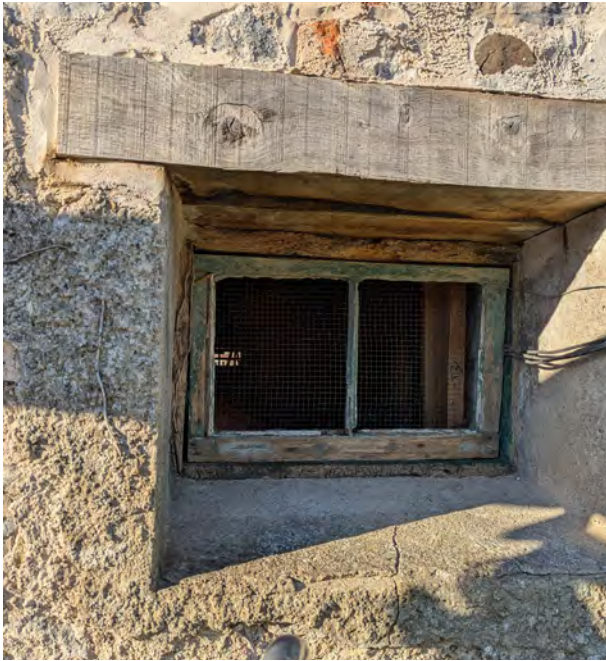
Rectangular window opening at high level within east facing gable wall, containing timber window frame with central mullion.
