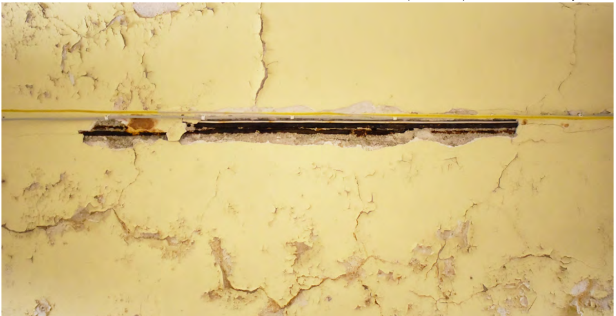
Metal bars, rusted, exposed at top of vaulted ceiling arch.
