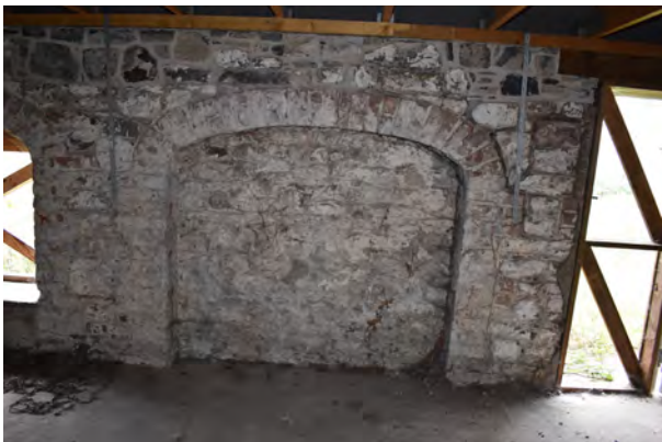
Blind archway filled with stonework.
