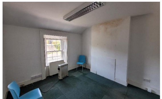
Fig 4.7.2. 1 st flr – staining at chimney
