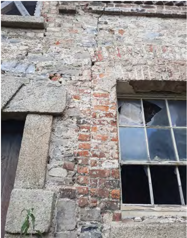
Crack in east facade between door and window at the north end of the facade. Damage to brick cornice.
