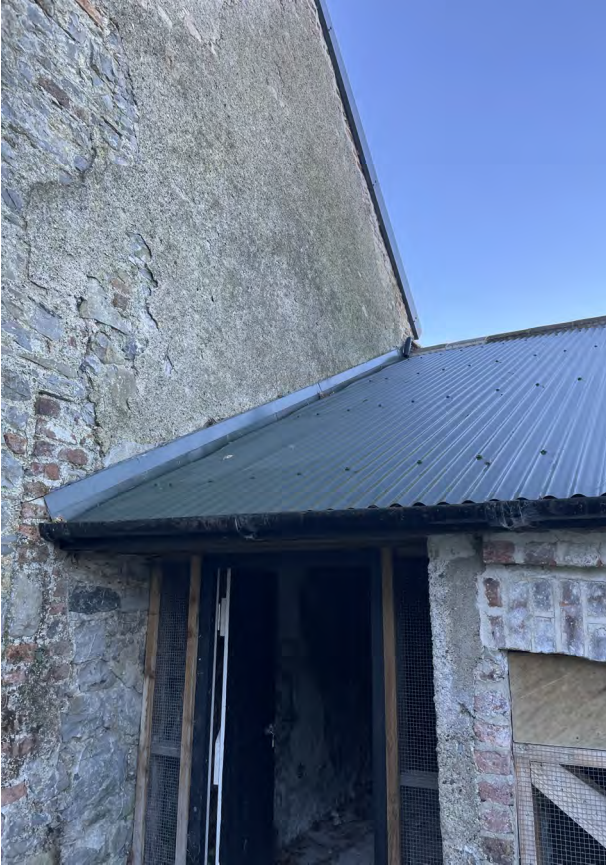
Roof abutment at junction with Building 2, pressed metal flashings.
