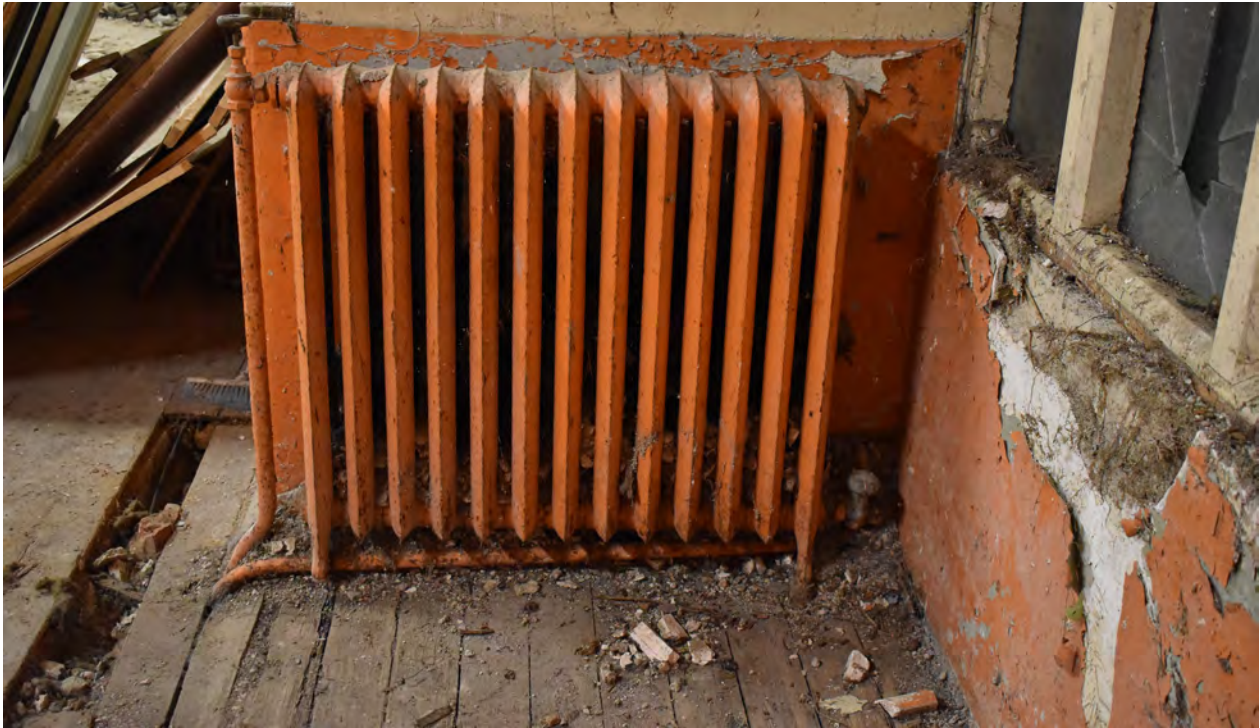
Cast iron radiators and associated pipework run along the perimeter of the external walls.
