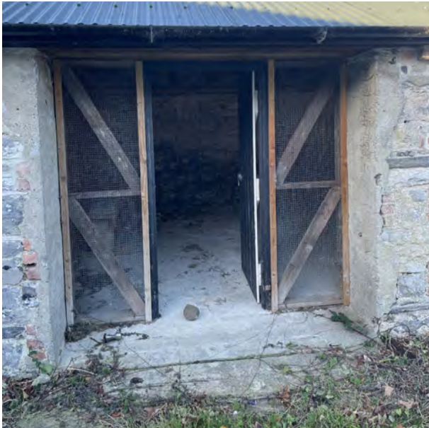
Archway completely demolished and fitted with a braced and ledged door within a mesh surround and a timber lintel. Pre-cast concrete has been installed on the approach to the doorway to create a sloping threshold.
