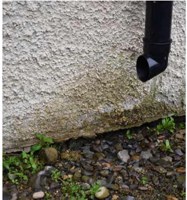
Downpipe outlet directed towards wall, causing staining to base of wall.
