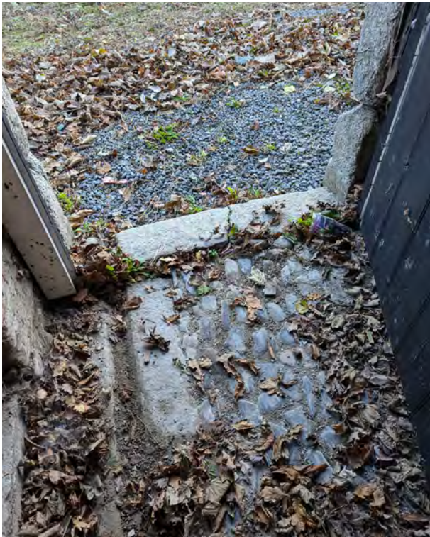
Floor surface to 2.6 consisting of cobbled surface edged with cut stone drainage channel leading to entrance. Crack in stone entrance threshold visible.
