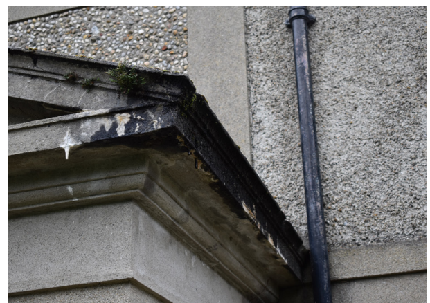
Figure 58 - Stone work to western entrance porch. The edges of the stone-work are damaged, with vegetation growth and damp staining visible
