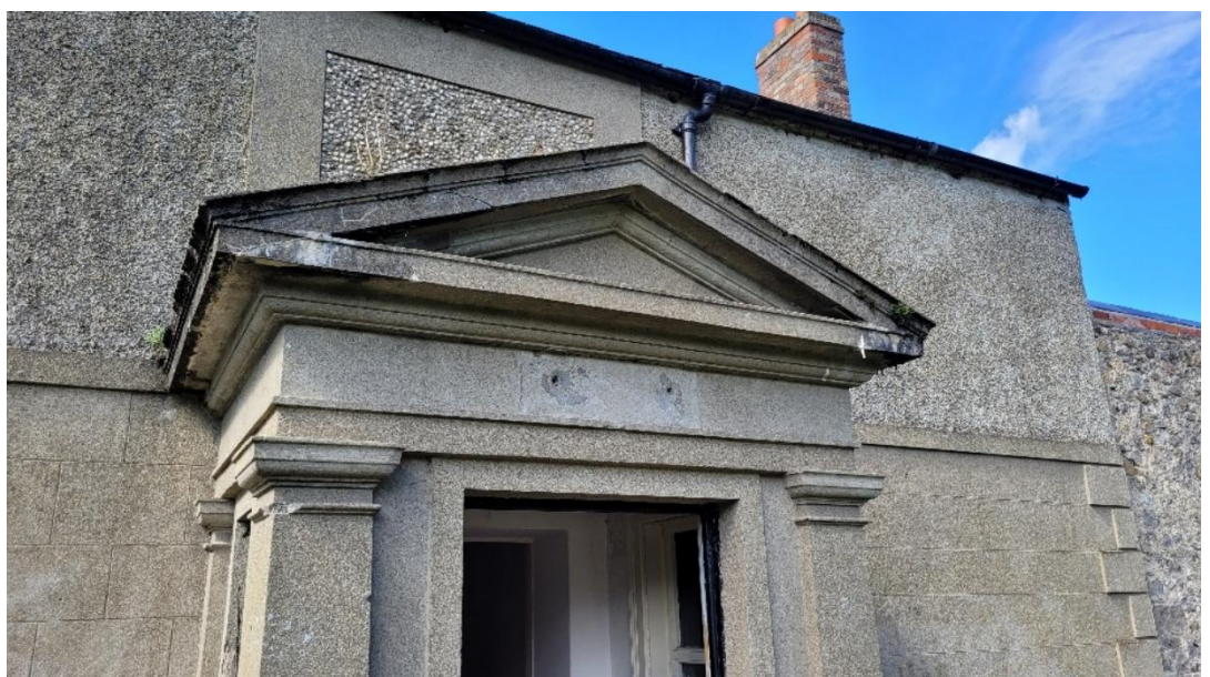
Fig 4.7.3. East Elevation detail – note cracked lime leaching render
