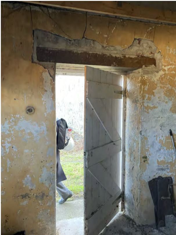
Interior view Building 5 (B), east wall, entrance door. Damage to plaster-work where lintel has previously been replaced.
