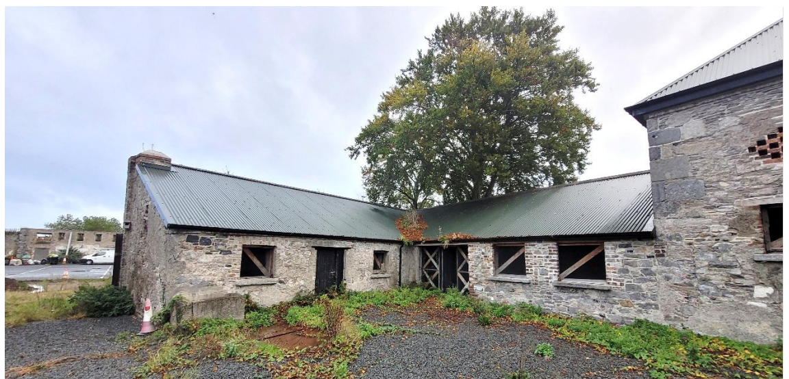
Fig 4.4.2 Elevation onto courtyard 02, note debris in valley and gutters.
