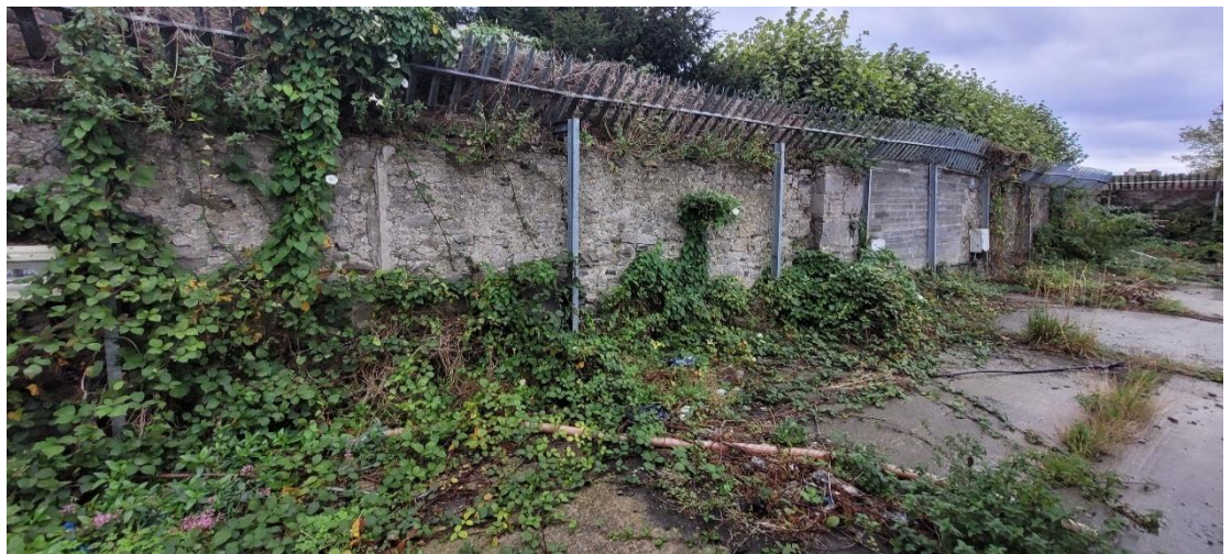
Fig 5.5.3 View of east face of west wall, note blockwork sections and vegetation growth.
