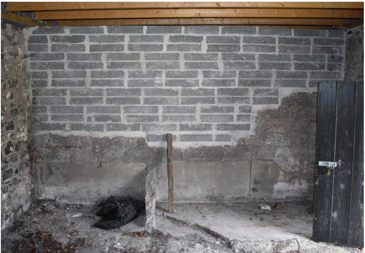
Dividing wall between west and north ranges. Remains of cattle stalls visible at base of the wall which has been built up to the base of the timber roof structure using concrete blocks.
