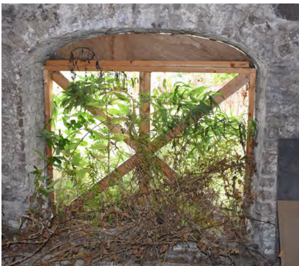
Vegetation growth in archway to northern end of west range.
