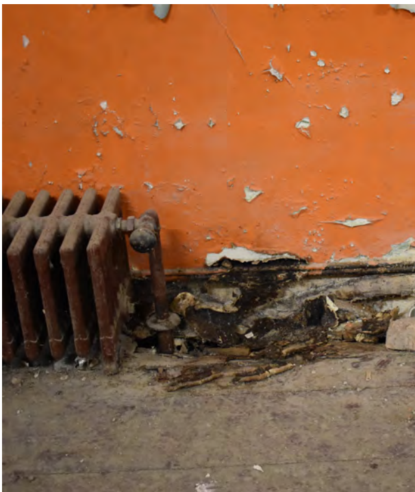
Cast iron radiator. Extensive damage to floorboards at base of radiator.
