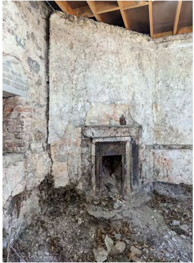
Remains of cast-iron fireplace and angled chimney breast in room 2.5. Interior plasterwork remains. Uneven ground surface consisting of rubble and loose cobbles.
