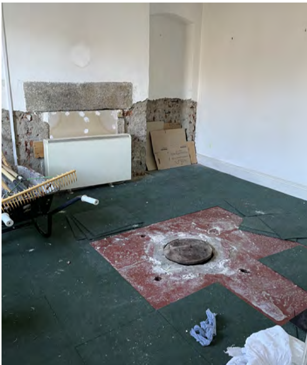
Ground floor room to the north. approx. 1m of internal plaster to the north facing external wall has been removed above finished floor level.
