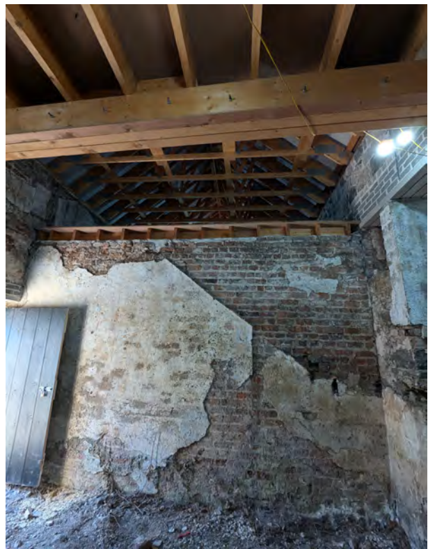
Remnants of lime plaster to wall of 2.5 indicating stairway leading to loft space.
