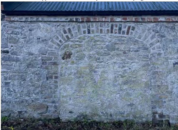
One of four blind archways which have been blocked up with random rubble stone. Partial areas of render remains.
