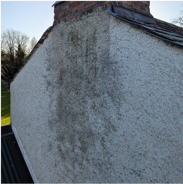
Figure 57 - Discolouration to north facing gable.
