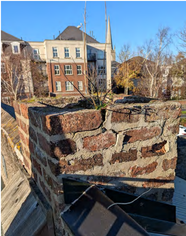
Vegetation growth has caused separation of the mortar joints causing damage to the chimney stack.
