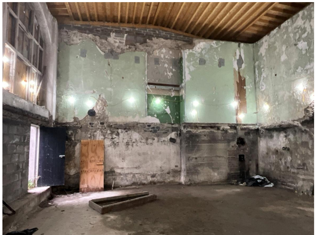
Fig 4.3.2 North wall of Cromwell's fort – note parrass plates at first floor level that tie Building B3 and plates at high level that support trussed rafter roof to B3.
