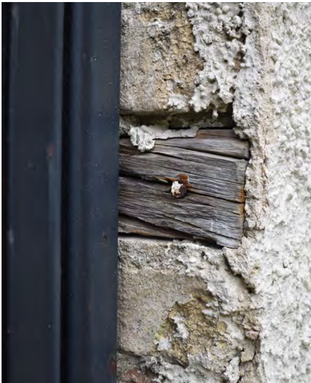
Detail of reveal to doorway in southern wall. Brick reveals with bedded timber fixings. Reveals are not rendered.
