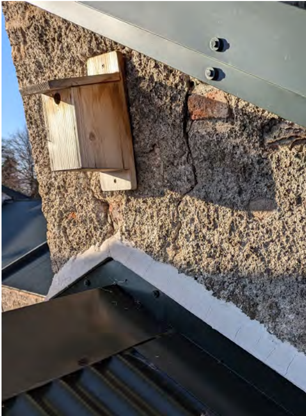
Nesting box to south wall above roof of building 5 (A). Crack visible in plasterwork to wall.
