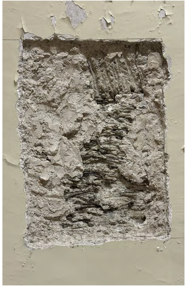
Plasterwork to ceiling exposed during 2018 site investigation works. The ceiling was made using a wicker basket frame that was subsequently plastered. The mortar was found to date from the 16th - 17th Century.
