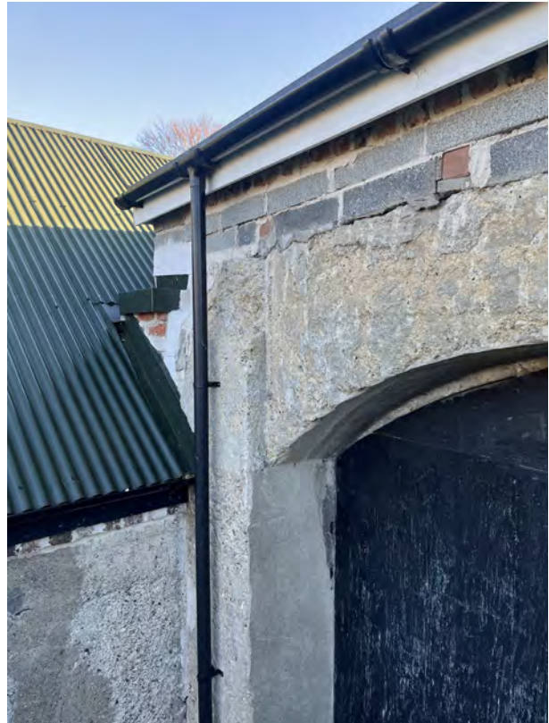
Unrendered blockwork built above existing brick & stone walls at North-West entrance.
