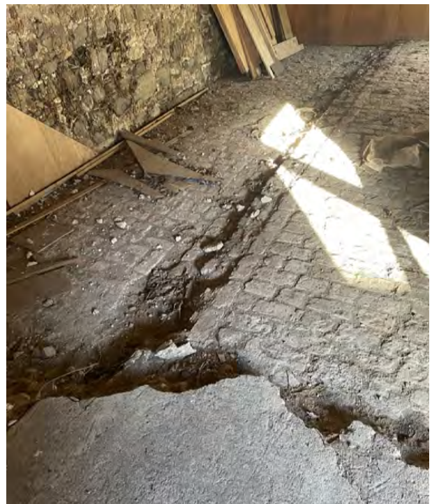
Drainage channel formed in stone setts.
