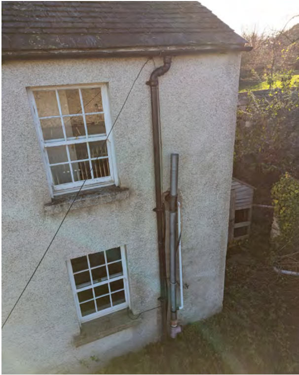
Untidy services stack and electrical wiring.
