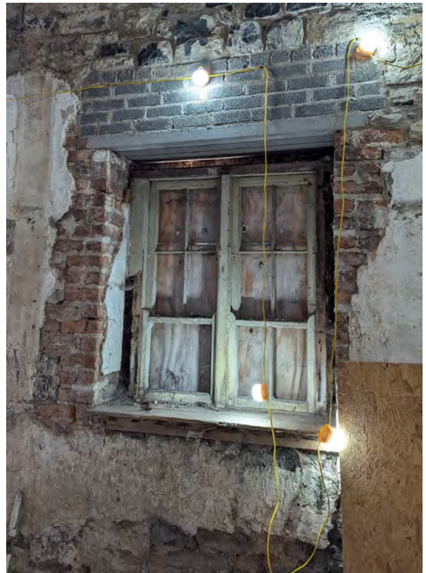
A pair of 4 over 2 format sliding sash windows with central mullion, to the right of entrance 2.1
