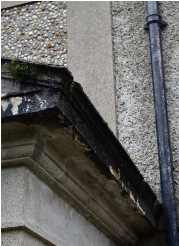
Stone work to western entrance porch. The edges of the stonework are damaged, with vegetation growth and damp staining visible
