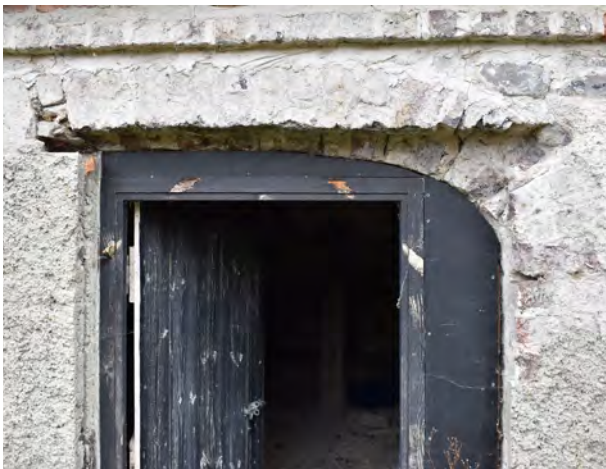
Doorway inserted into one half of the central arch in the north range.
