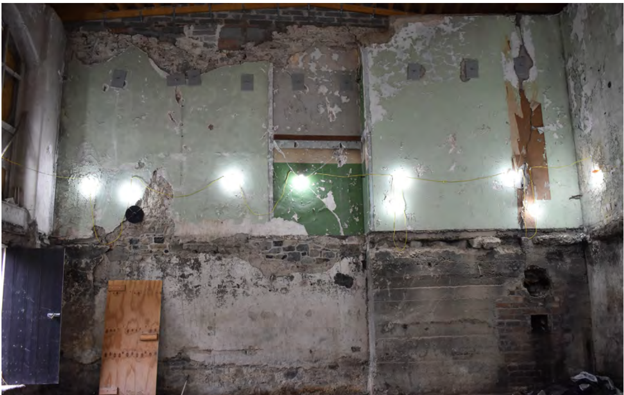
Northern wall, Room 2. Walls are in poor condition. There is damage to masonry where the first floor and services installations have been removed.
