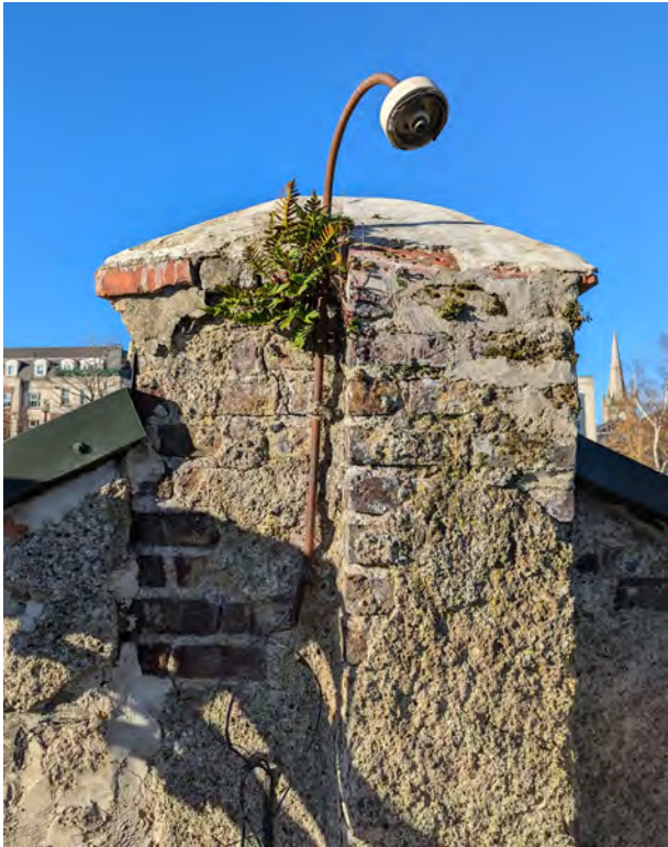
The shared wall with Building 6 forms a pier, matching that of Building 4. Vegetation growth is visible from the top of the pier, near a redundant lighting fixture. Render partially remains but is in poor condition.
