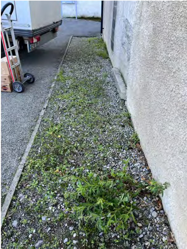
Gravel drainage channel of approx. 1m width to the base of the walls to the east facade. Vegetation growth visible.
