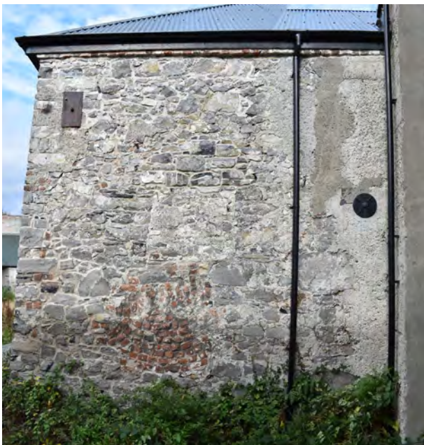
South Facade. There is an unusual brick repair in a round or circular fashion approx .5m – 1m above ground level.
