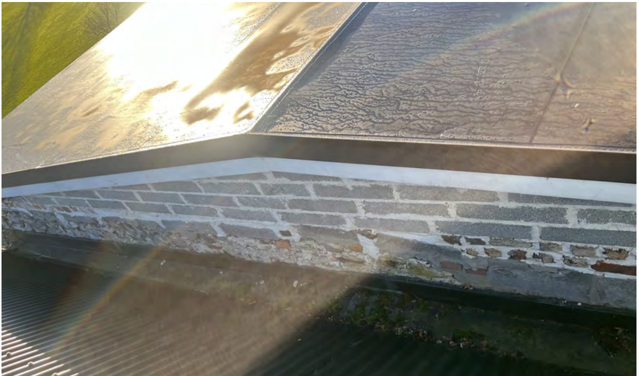
Unrendered blockwork built upon existing brick / stone wall, form gable end of pitched roof.
