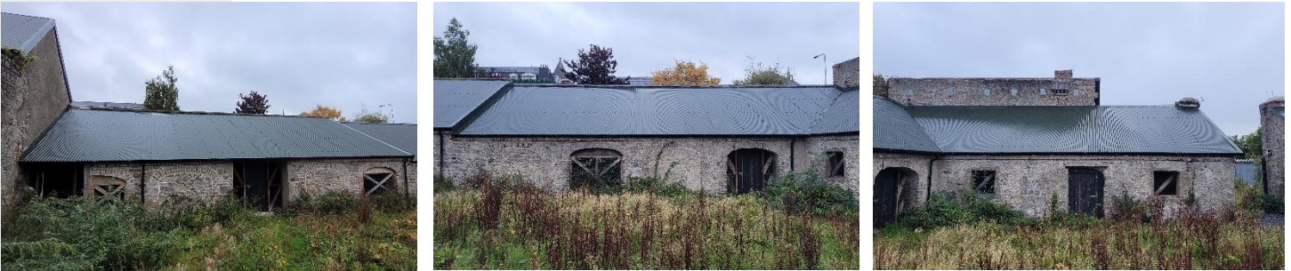
Fig 4.6.1 shallow pitched roofs and steps in roofs along elevation. There may be some capacity to raise roof to north (rhs) section against flank wall of Building 5
