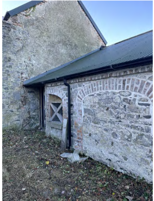
Partially demolished archway and adjacent blind archway situated to the southern end of the west range.
