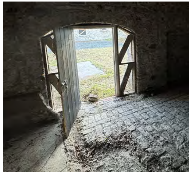
Archway fitted with timber bracing and door.
