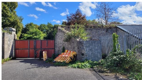
Fig 5.2.2 West side of Wall A - Vegetation control; wall top and localised repairs required.
