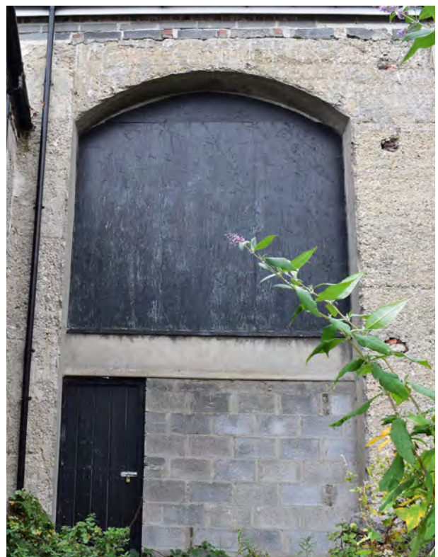
Ope 14 (A) plywood covering to ope; (B) Timber panelled door and block-work infill.
