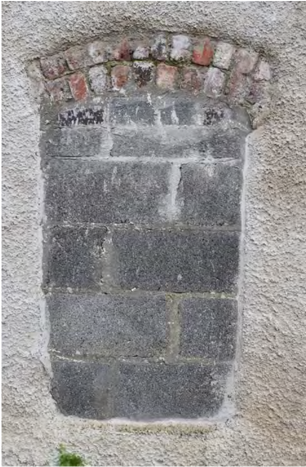
Ope 12, blockwork infill unrendered. Brick arch visible. Missing cill.
