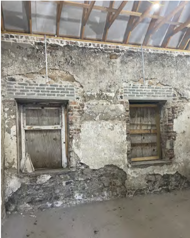
Window opes in room 2.3. New concrete lintels and blockwork have been installed above. A course of brickwork has been added to the tops of the walls to take the wallplate of the new timber structure.
