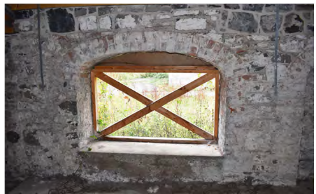
Modified archway with raised cill to create window opening. Opening braced with timber and fitted with protective mesh.
