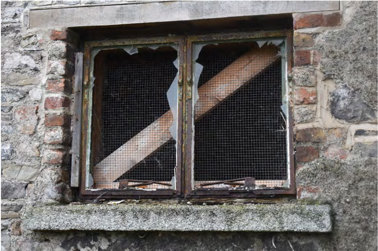
Window opening with two pivot-hinged metal casement windows and central mullion, granite cill.
