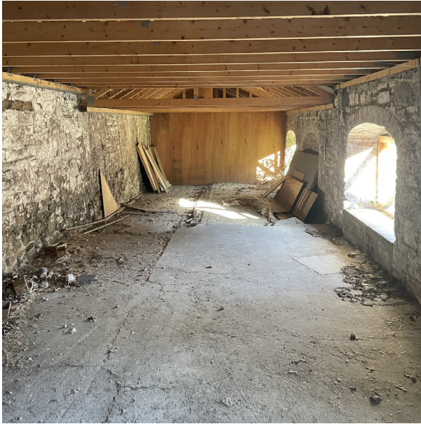
Figure 50 - Building 6, west range interior. The floor slopes significantly downwards heading north.
