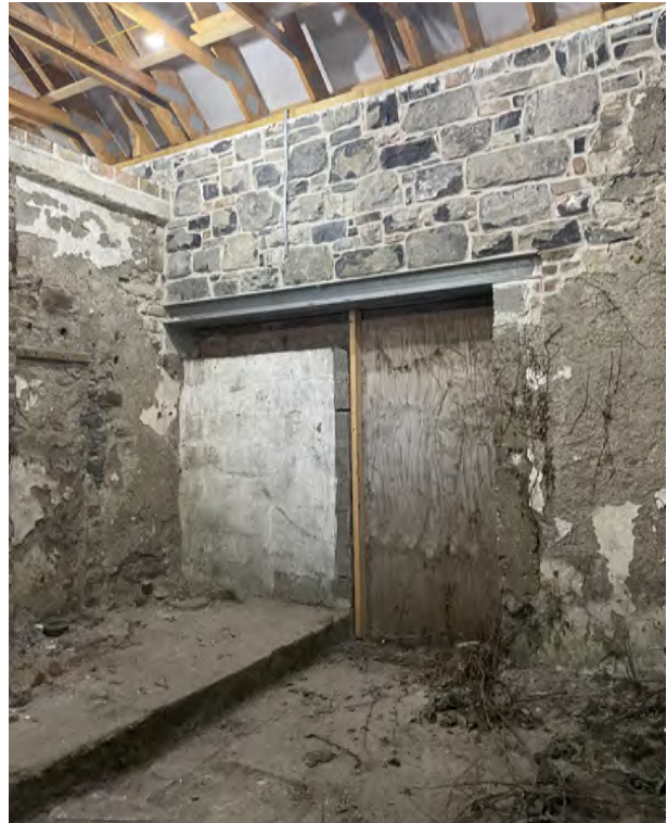
Doorway to 2.4 (leading to Rathfarnham Road). New steel lintel and calp limestone built to wall top.
