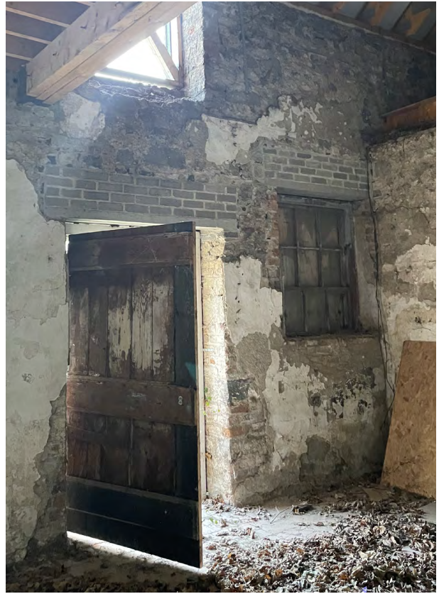
Braced and ledged door to 2.7, recently repaired. 6 over 3 timber sash window.
