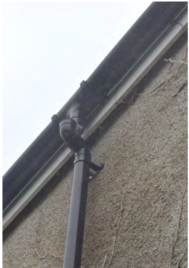
Downpipe out of alignment with gutter outlet.
