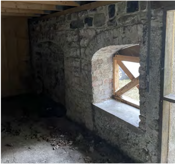
Partially demolished vaulted opening, modified cill height.
