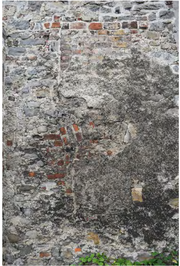
Blocked up openings visible behind remnants of plasterwork on western gable.
