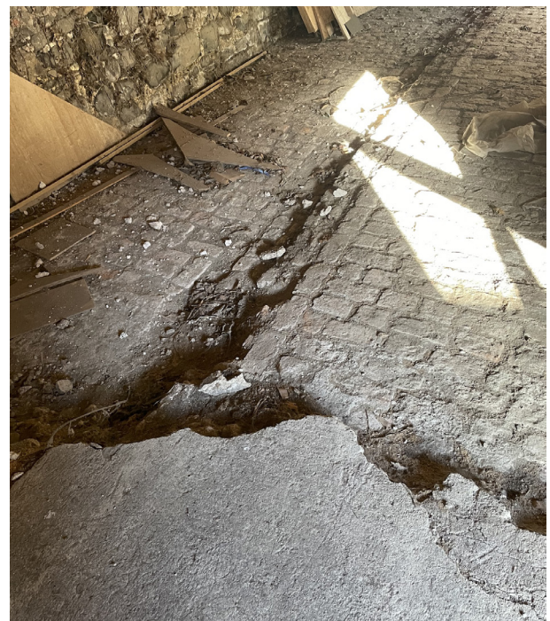
Figure 51 - Building 6, west range, drainage channel formed in stone setts.
