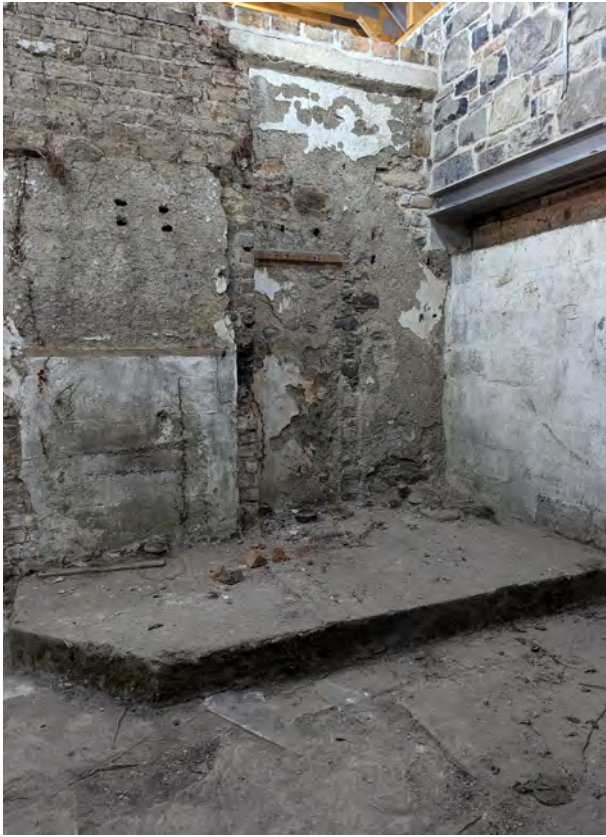
Raised concrete slab in the south-west corner of room 2.4 contains three former WC drainage pipes. These correspond to the location of a soil vent pipe externally on the West facade.
