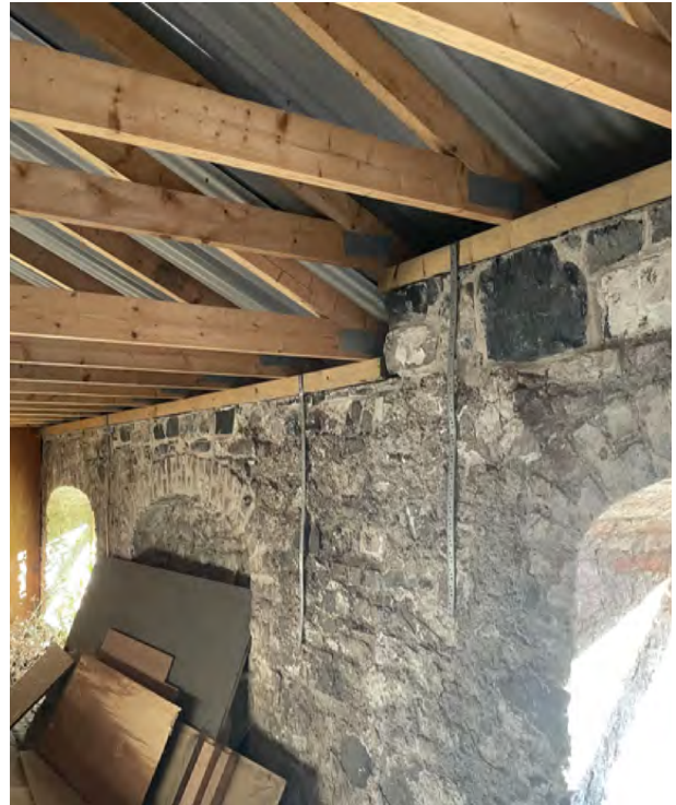
Timber roof structure and wall plate fixed to tops of masonry walls.
