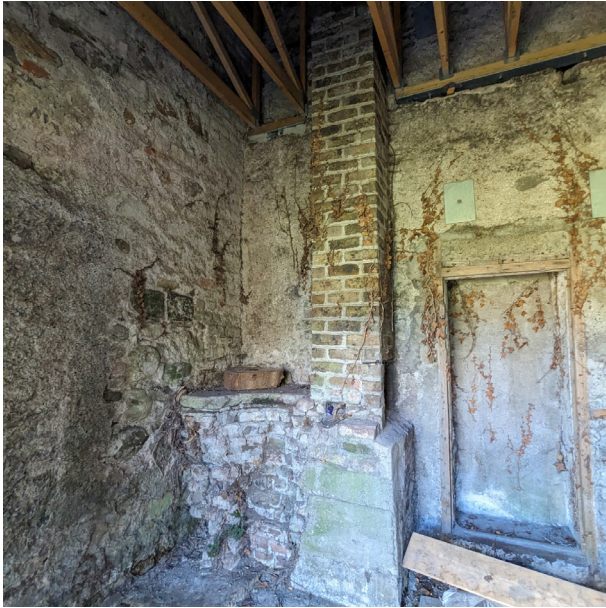
Figure 47 - Interior building 5 (A), chimney stack with widened base, resembling construction of a forge.
