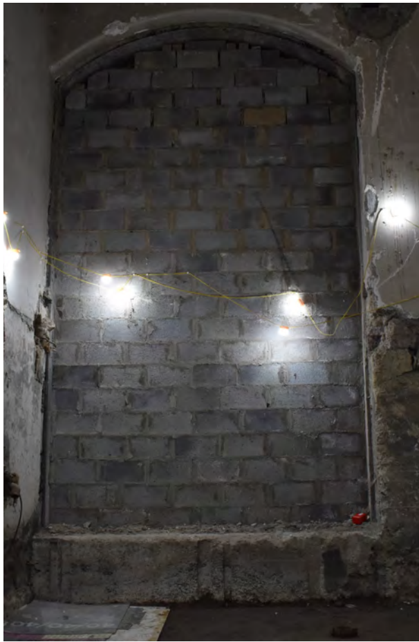
Ope 13 - 2 storey arched opening, blockwork infill.
