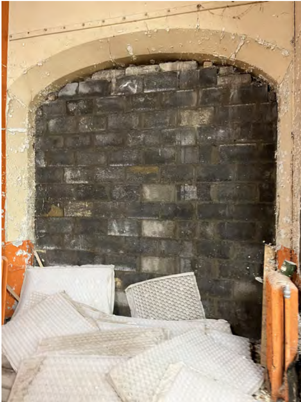
Ope 1 Exposed blockwork to former window ope in eastern wall.
