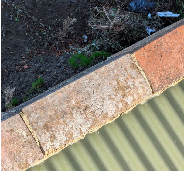
Figure 42 - Clay ridge tiles bedded on to profiled metal roof of Building 4. Maker's mark visible.
