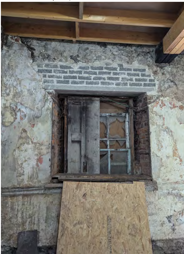
Window joinery including 6 over 3 sash window and shutters stored within the existing ope. Concrete lintol and blockwork over. Textured obscure glass remains, mostly broken.
