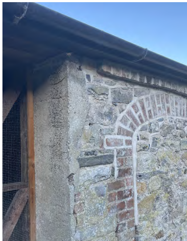
Recent repointing of mortar joints visible at brickwork and tops of walls.
