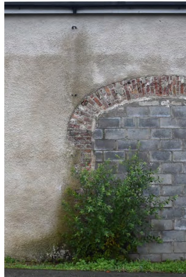
Missing downpipe resulting in staining to wall, vegetation and algae growth. Horizontal line of saturation visible on plasterwork above archway. This was visible running the length of the eastern facade.
