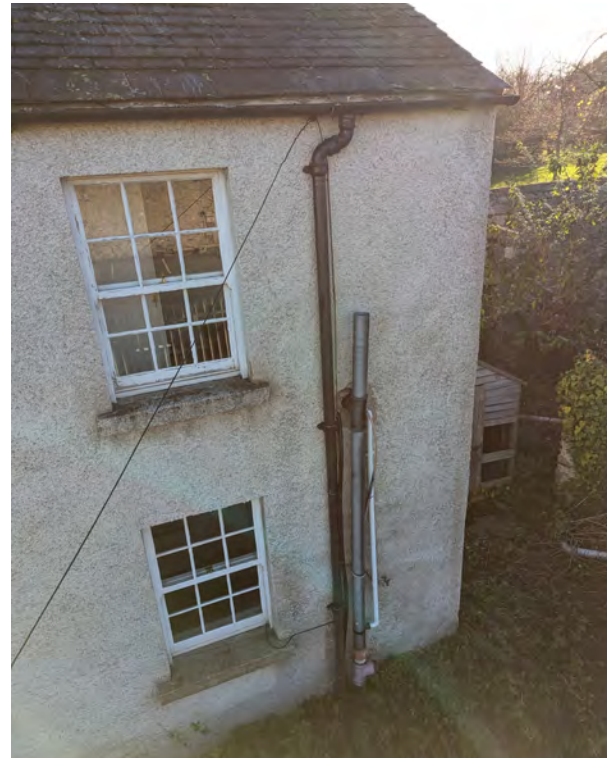
Untidy services stack and electrical wiring.
