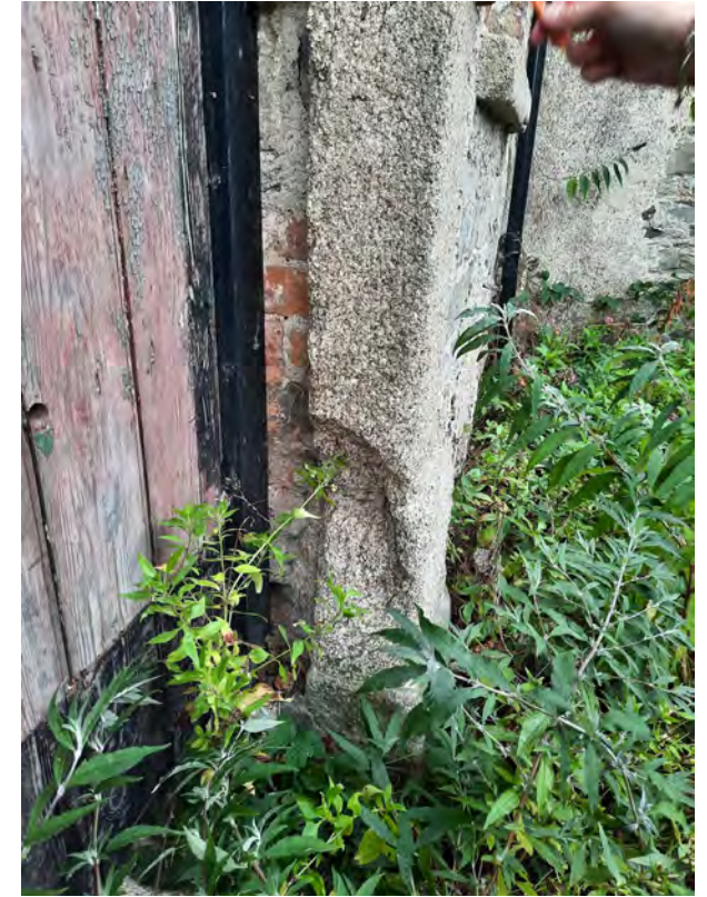
Damage to stone doorway surround at entrance to 2.7
