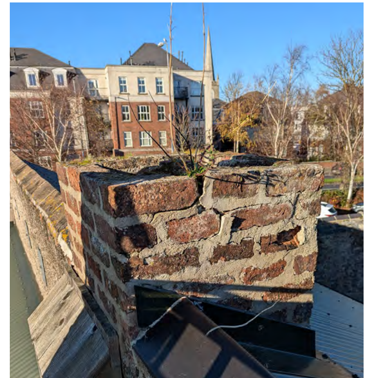
Vegetation growth has caused separation of the mortar joints causing damage to the chimney stack.
