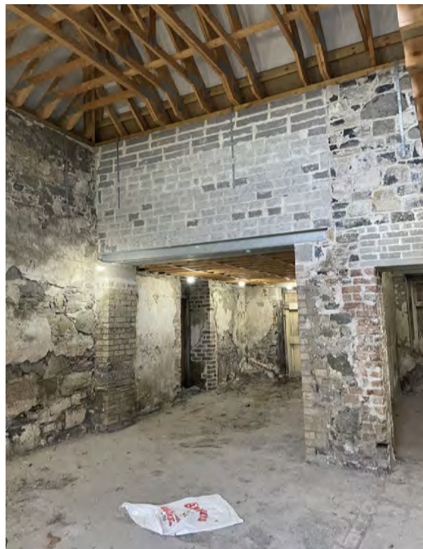
Recently installed steel lintol with concrete blockwork to wall top above opening between 2.1 and 2.2
