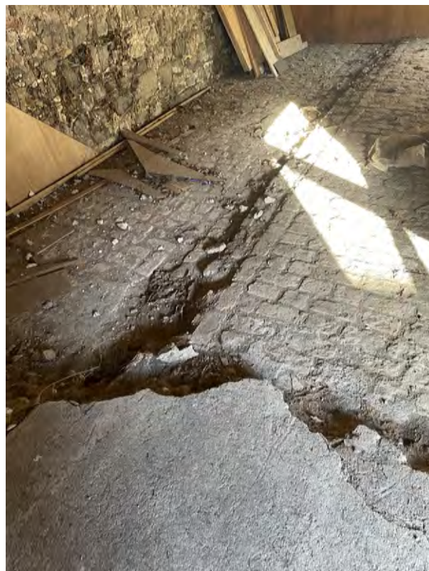
Drainage channel formed in stone setts.
