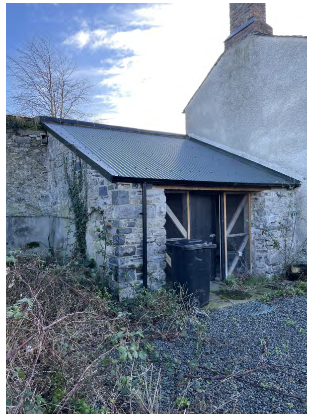
The single storey building to the north has been reroofed in a profiled metal sheeting and has pvc gutters and downpipes.
