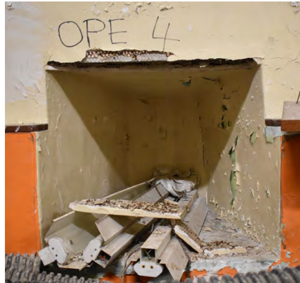
Ope 4 Former opening in eastern wall, plastered and painted. There is no corresponding opening visible externally.
