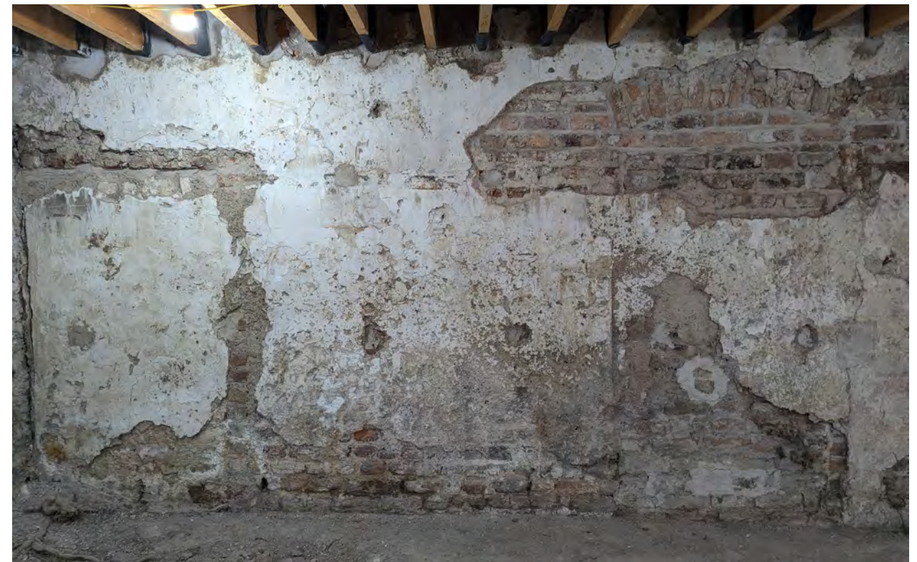
Previous openings in wall between 2.2 and 2.3 partially visible, infilled with brickwork and finished with lime plaster.
