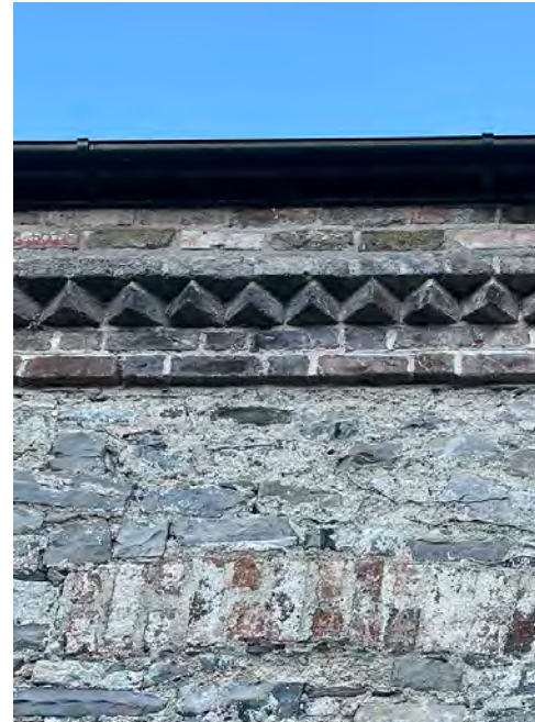
Figure 37 - Building 2, brick chevron detail
