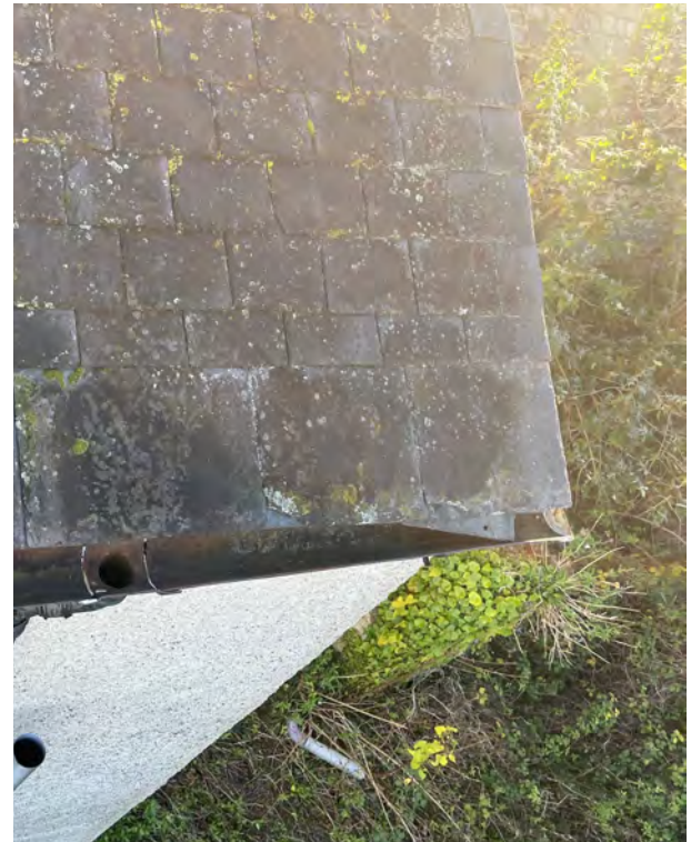
Slipped slate above gutter line. Note large format slates along the bottom course.
