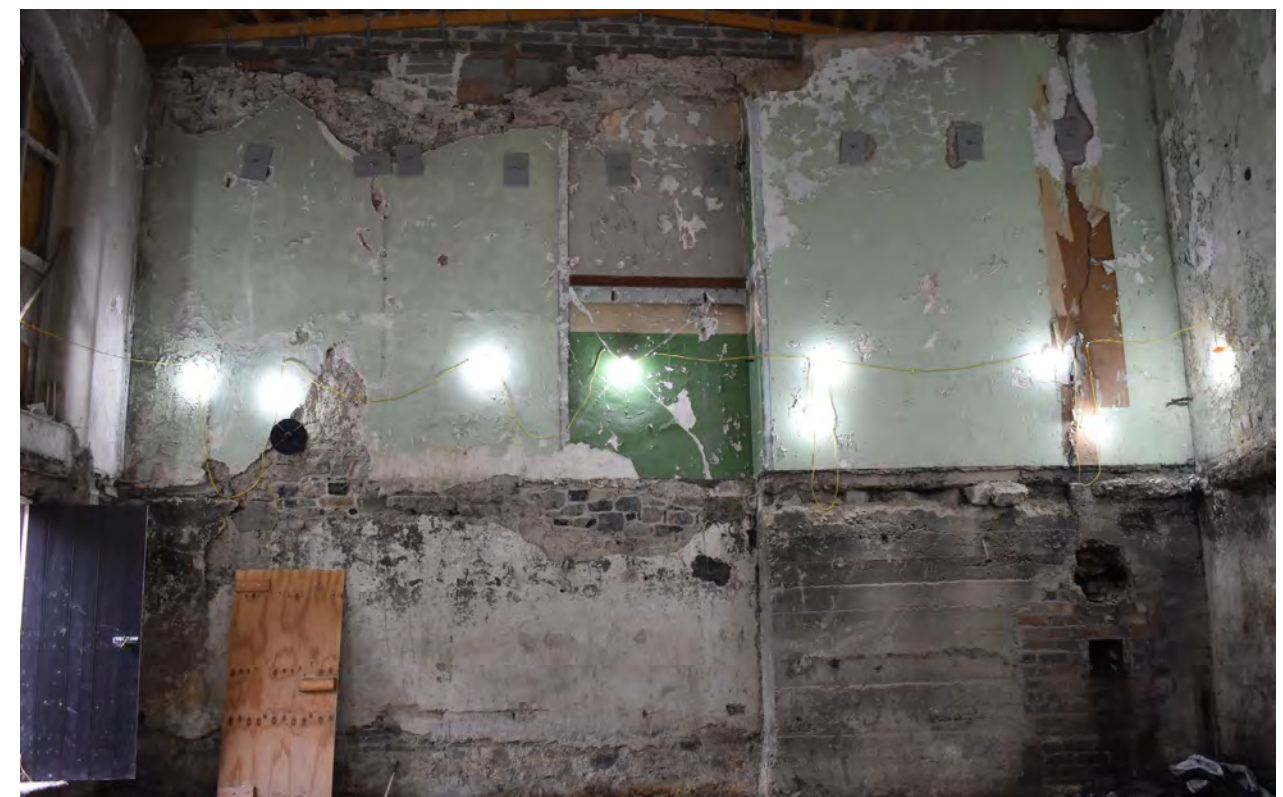
Northern wall, Room 2. Walls are in poor condition. There is damage to masonry where the first floor and services installations have been removed.
