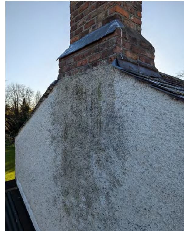
Damp staining to north facing gable.
