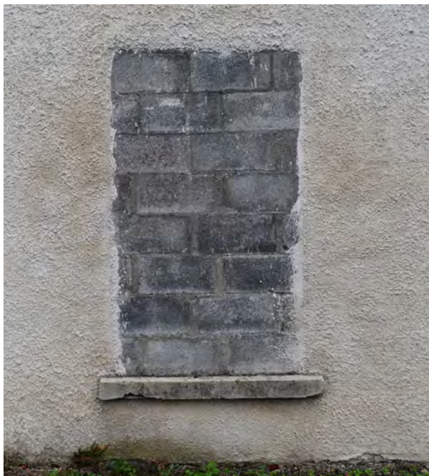
Ope 2, blockwork infill unrendered. Damage to concrete cill.
