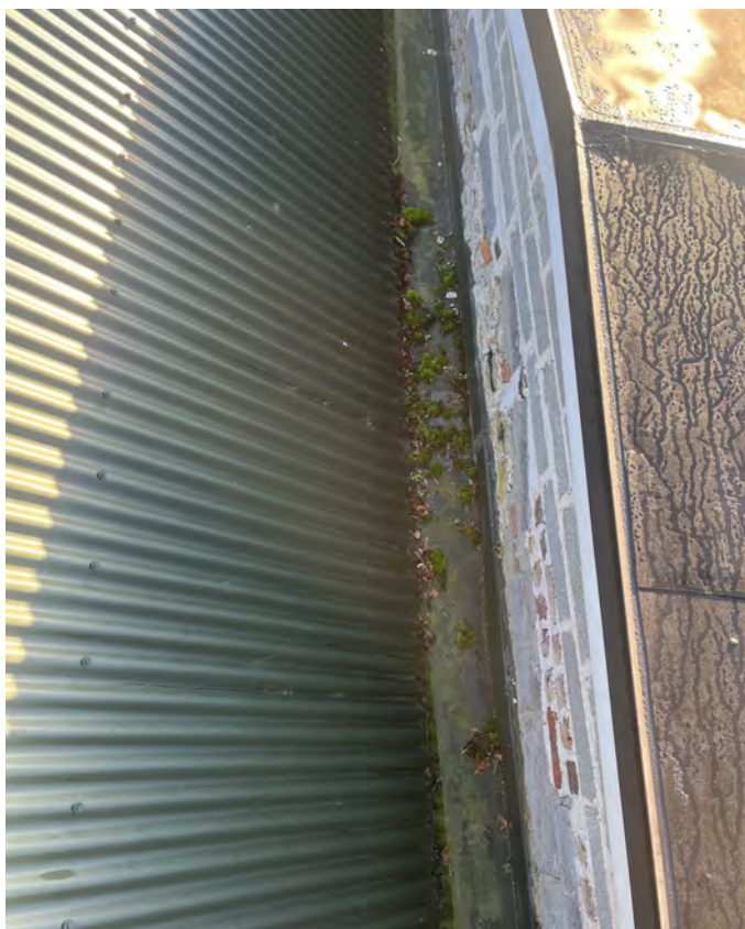
Valley gutter, areas of minor moss growth in central area.
