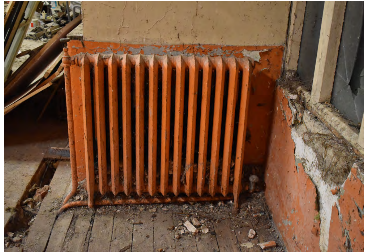
Cast iron radiators and associated pipework run along the perimeter of the external walls.
