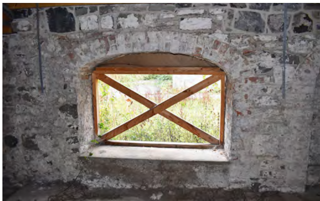
Modified archway with raised cill to create window opening. Opening braced with timber and fitted with protective mesh.
