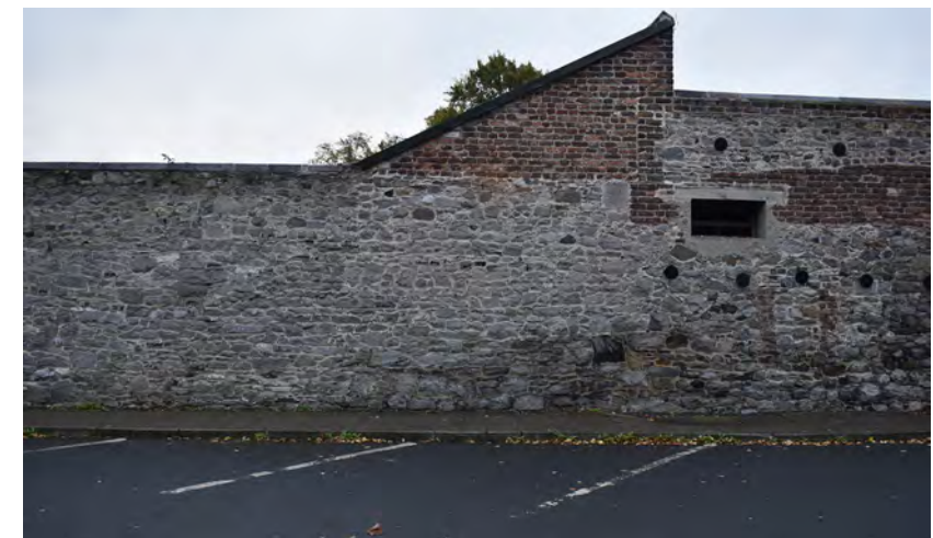
Figure 73 - Junction of Building 5 & 6, higher roof forming 'clerestory'
