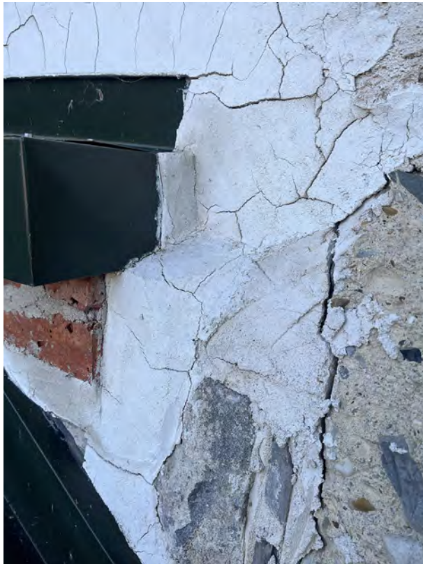
Cracks visible in plasterwork to North-West corner where edge of gully meets corner of wall.
