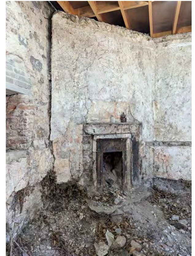
Remains of cast-iron fireplace and angled chimney breast in room 2.5. Interior plasterwork remains. Uneven ground surface consisting of rubble and loose cobbles.
