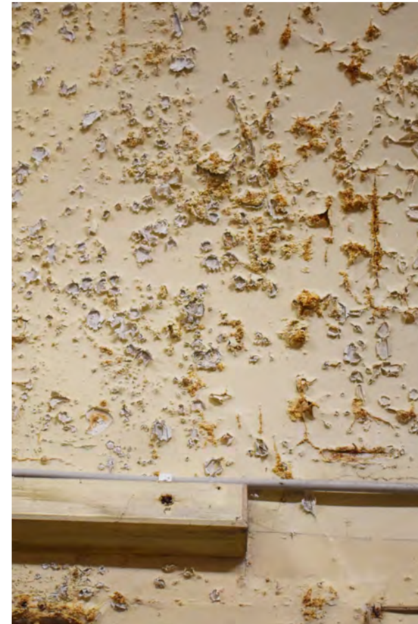
Extensive damage to paintwork throughout, including peeling and growth to walls indicating dampness internally.
