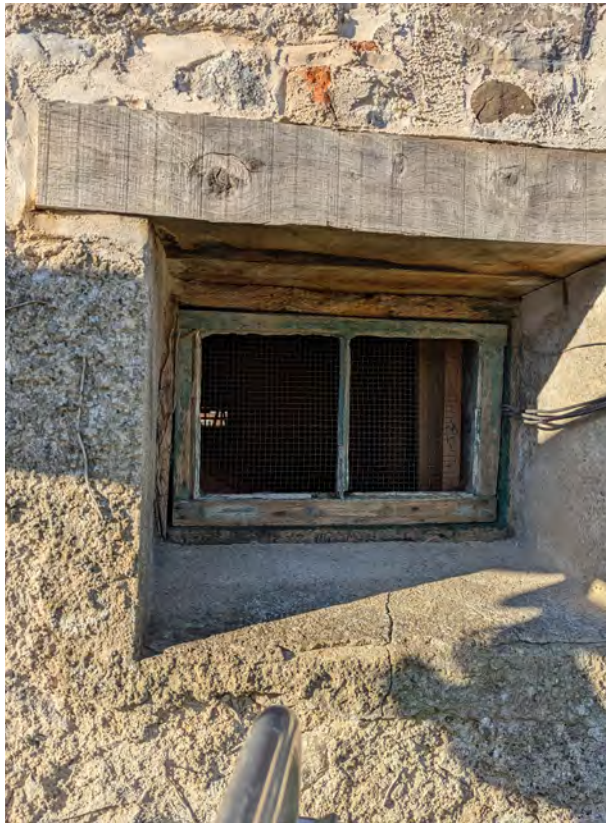
Rectangular window opening at high level within east facing gable wall, containing timber window frame with central mullion.
