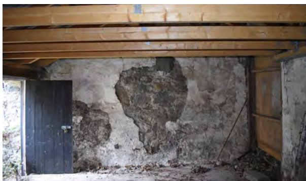
The southern interior wall is part of the gable of Building 2. Areas of whitewashed lime plaster remains. Where damaged the random rubble stone is visible. Doorway to the left of image leads to Rathfarnham Road.
