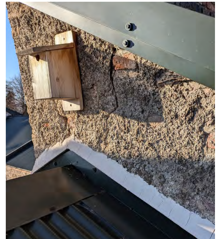
Nesting box to south wall above roof of building 5 (A). Crack visible in plasterwork to wall.
