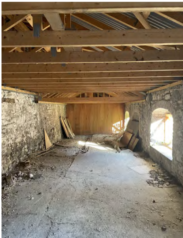
Interior of the west range. The floor is covered in approx. 150mm concrete within most of the southern portion of the west range, and slopes significantly to the north.
