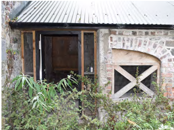
Archway partially demolished to the south of Building 6. A braced and ledge door has been fitted to one half, and a square window opening inserted into the other half.
