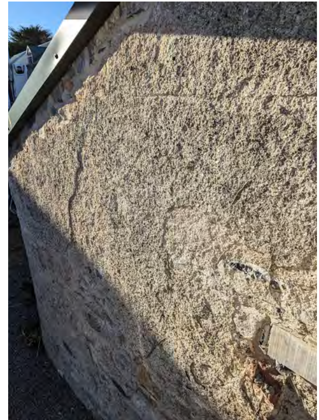
Lime render partially remains on the east facing gable, but shows signs of spalling and crumbles to touch.
