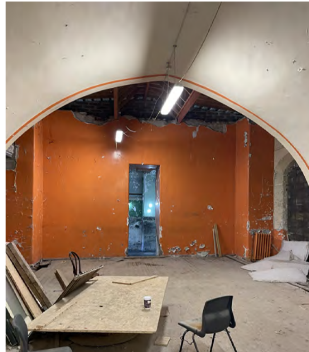
Barrel vaulted ceiling to interior of Cromwell's Fort, looking north.
