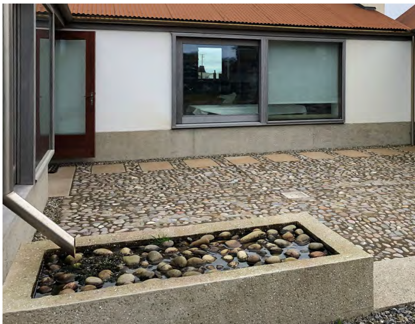
Figure 84 - Stone filled rainwater 'trough' detail by Donaghy Dimond Architects
