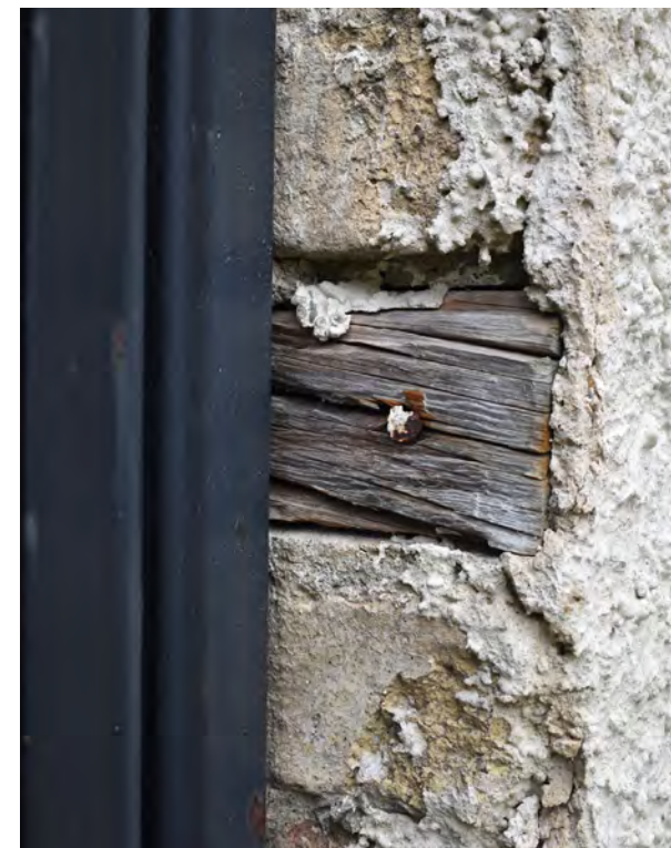
Detail of reveal to doorway in southern wall. Brick reveals with bedded timber fixings. Reveals are not rendered.
