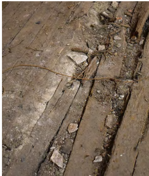
Damage to floorboards in north-west corner of Room 1 above likely services route to nearby radiators.
