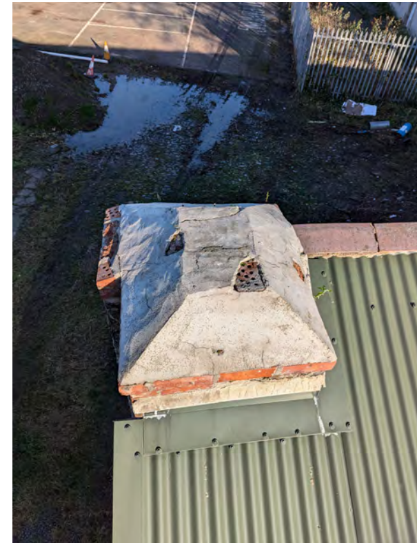
Rendered brick capping to projecting pier at west gable wall.
