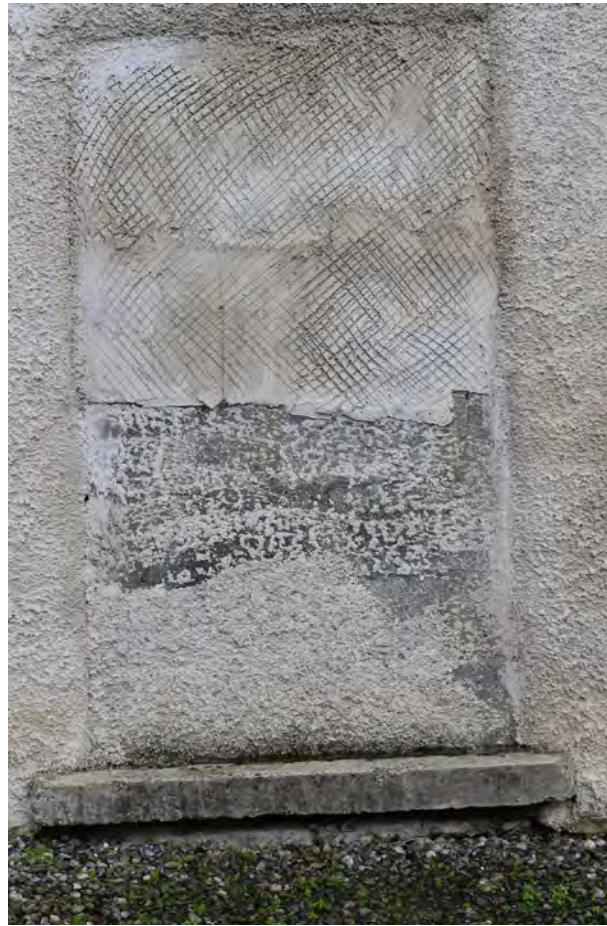
Ope 12, blockwork infil, partially rendered. Concrete cill.
