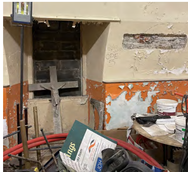
Ope 5: Exposed blockwork to former window ope in eastern wall.
