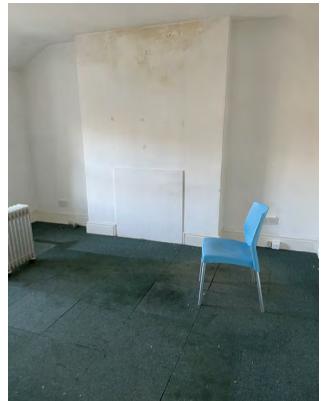
Discolouration to top of chimney breast, first floor, north room.
