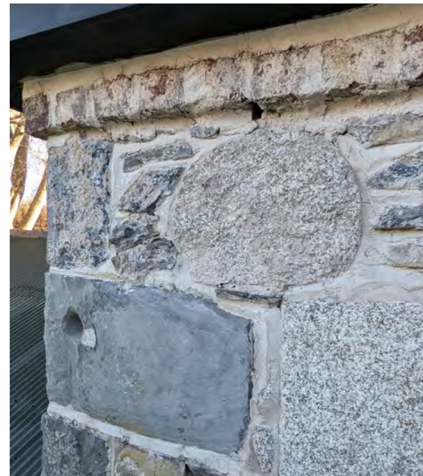
Rounded granite stone visible in western elevation. Recent repairs to mortar visible.
