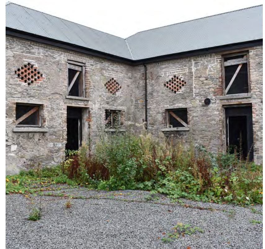
Figure 42 - Building 3, Diamond shaped brick in a perforated checker-board pattern
