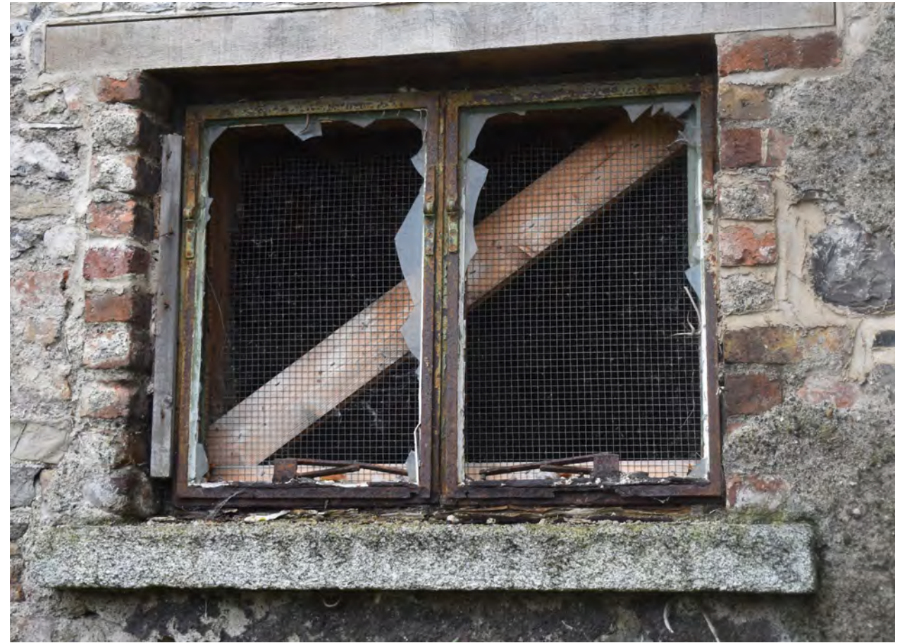
Window opening with two pivot-hinged metal casement windows and central mullion, granite cill.
