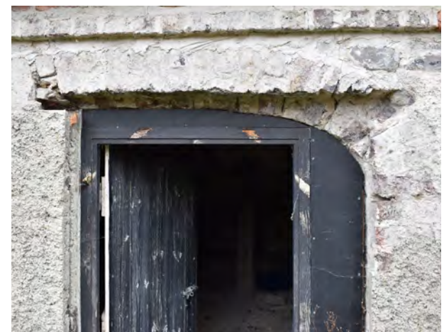
Doorway inserted into one half of the central arch in the north range.
