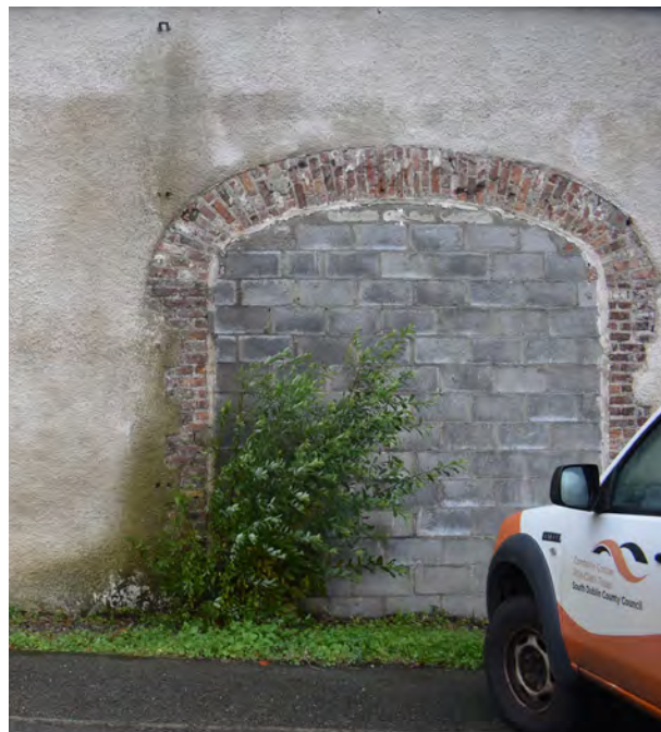
Ope 1, blockwork infill to brick carriageway arch.
