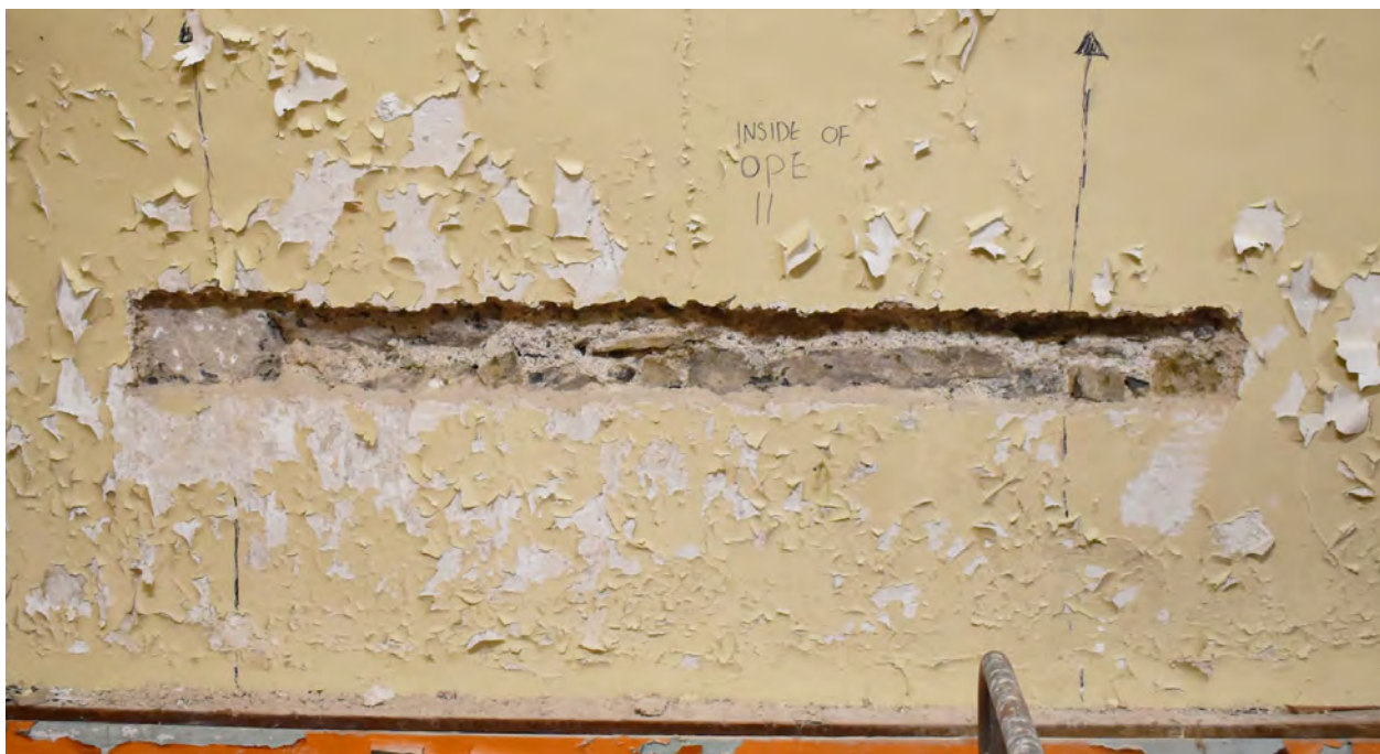
Previous investigations adjacent to Ope 6. Location corresponding with blind ope visible externally (Ope 11). The location of a corresponding internal ope was found to be inconclusive.
