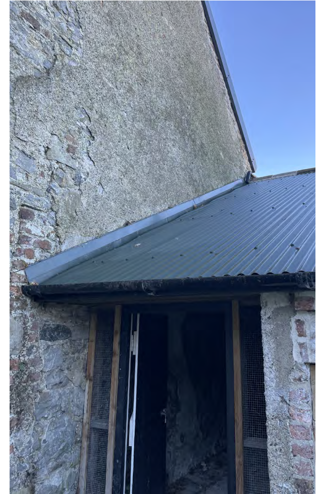
Roof abutment at junction with Building 2, pressed metal flashings.
