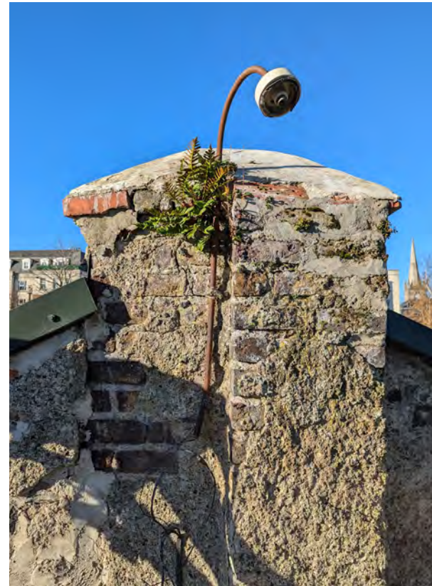
The shared wall with Building 6 forms a pier, matching that of Building 4. Vegetation growth is visible from the top of the pier, near a redundant lighting fixture. Render partially remains but is in poor condition.
