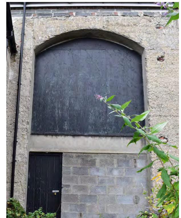
Ope 14 (A) plywood covering to ope; (B) Timber panelled door and blockwork infill.
