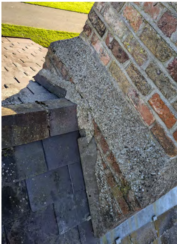
The render to the base of the southern chimney appears loose
