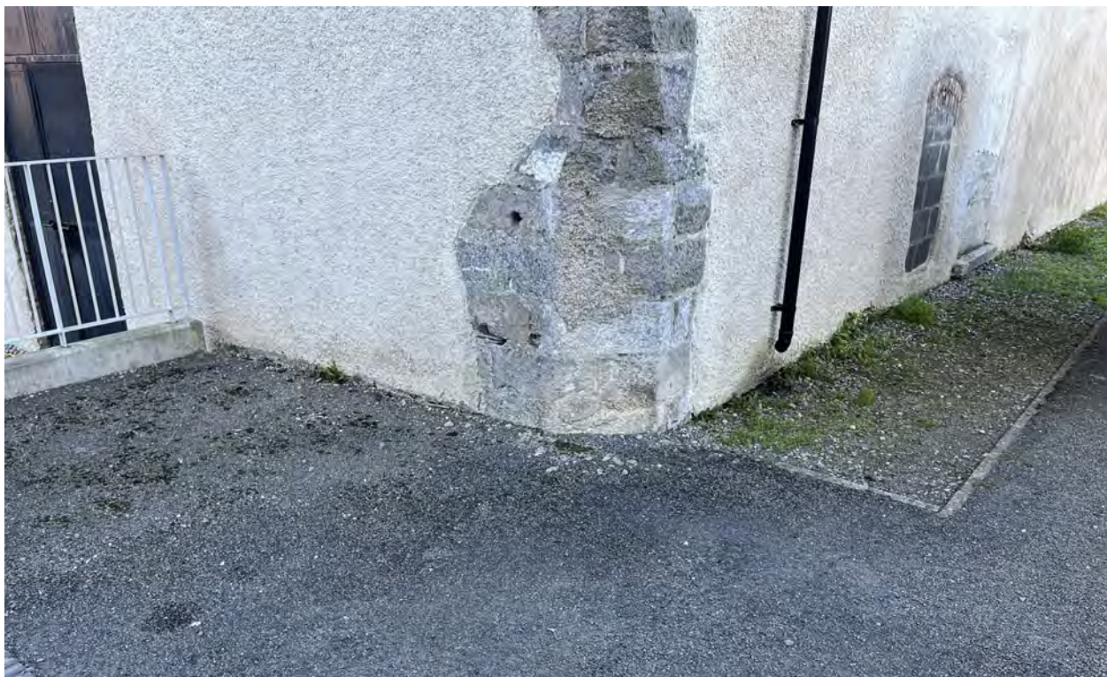
South-East corner of Cromwell's Fort. Gravel drainage channel of approx. 1m width to the base of the eastern wall. The asphalt road surface has been built up against the base of the southern wall. There is a change in level where the ground has been built up by approx 600mm at the base of the wall.
