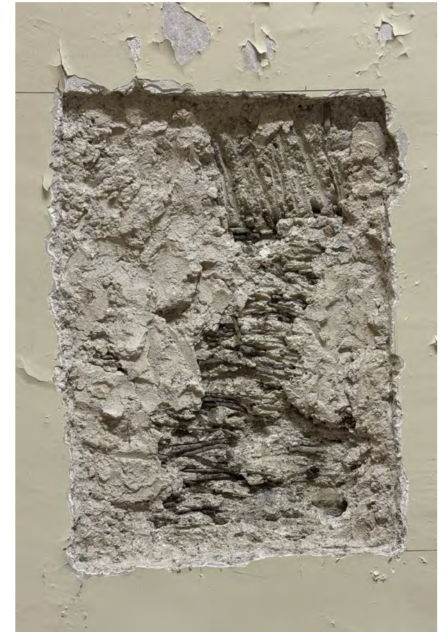
Plasterwork to ceiling exposed during 2018 site investigation works. The ceiling was made using a wicker basket frame that was subsequently plastered. The mortar was found to date from the 16th - 17th Century.
