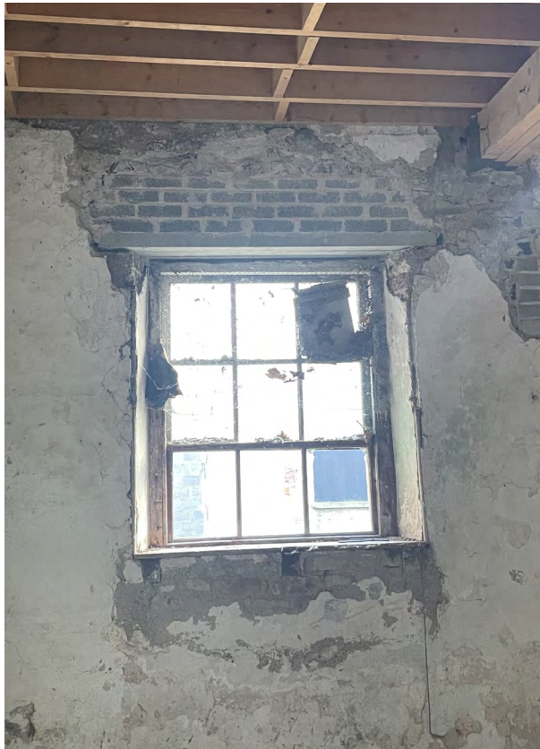
6 over 3 timber sash window in room 2.7. Records from 2018 works report this window to be fitted with a hinge allowing the sash to pivot open.
