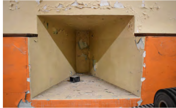
Ope 3 Former opening in eastern wall, plastered and painted. There is no corresponding opening visible externally.
