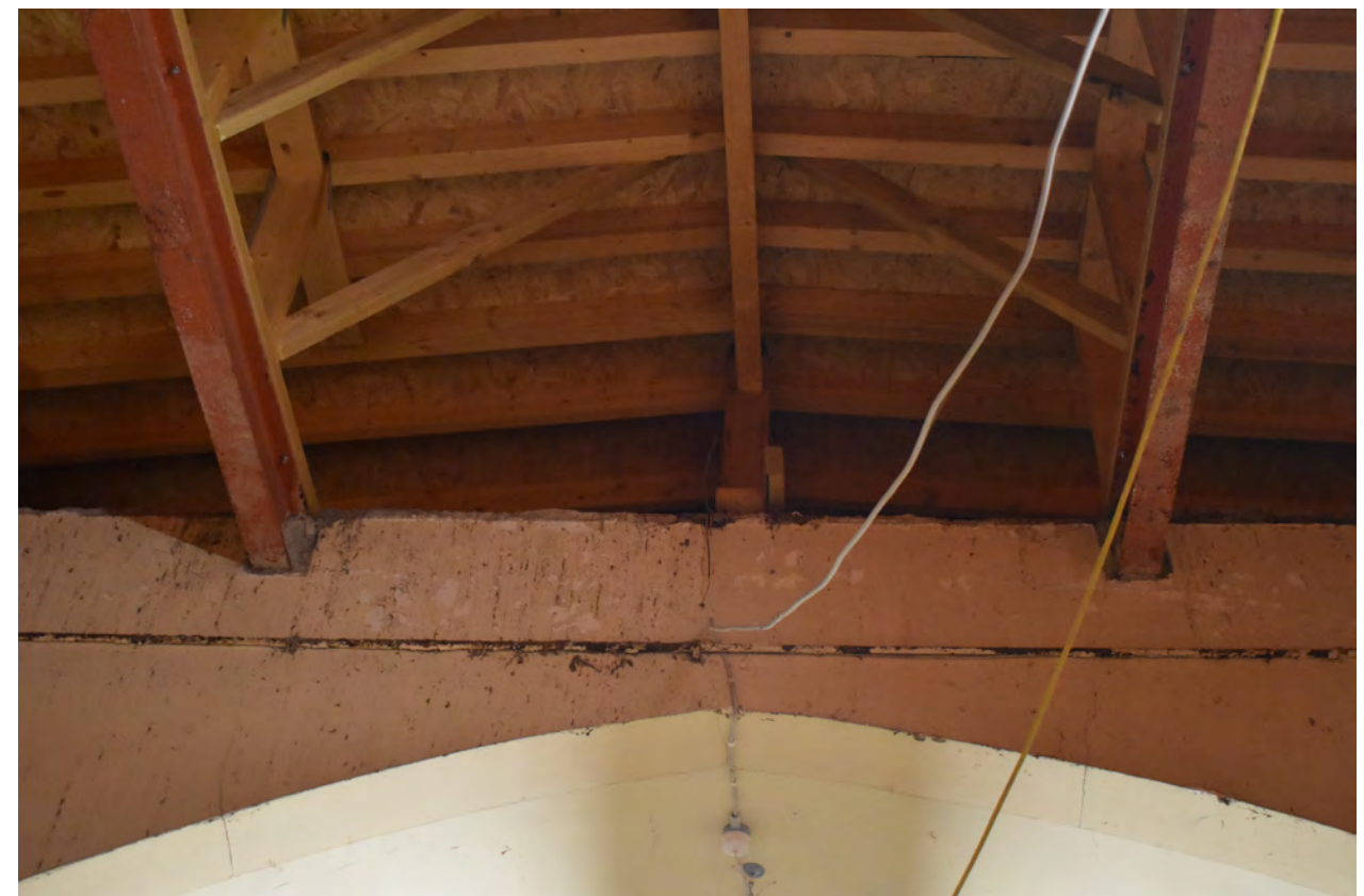
Timber roof structure supported by steel beams. Continues above the vaulted structure.
