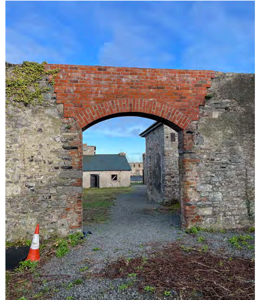
Figure 111 - Arch between Courtyard 1 & 2 rebuilt as part of 2018 works
