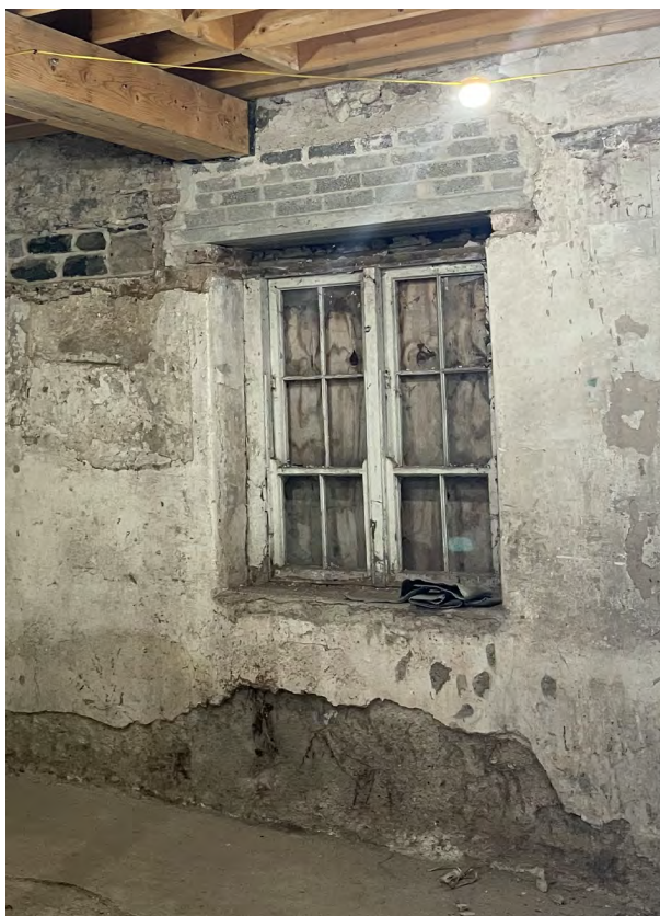
A pair of 4 over 2 format sliding sash windows with central mullion, to the left of entrance 2.1
