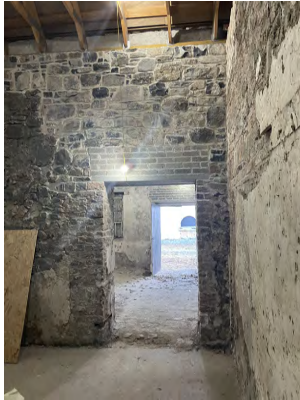
Recently installed concrete lintol, concrete blockwork and stonework to opening between 2.1 and 2.3.
