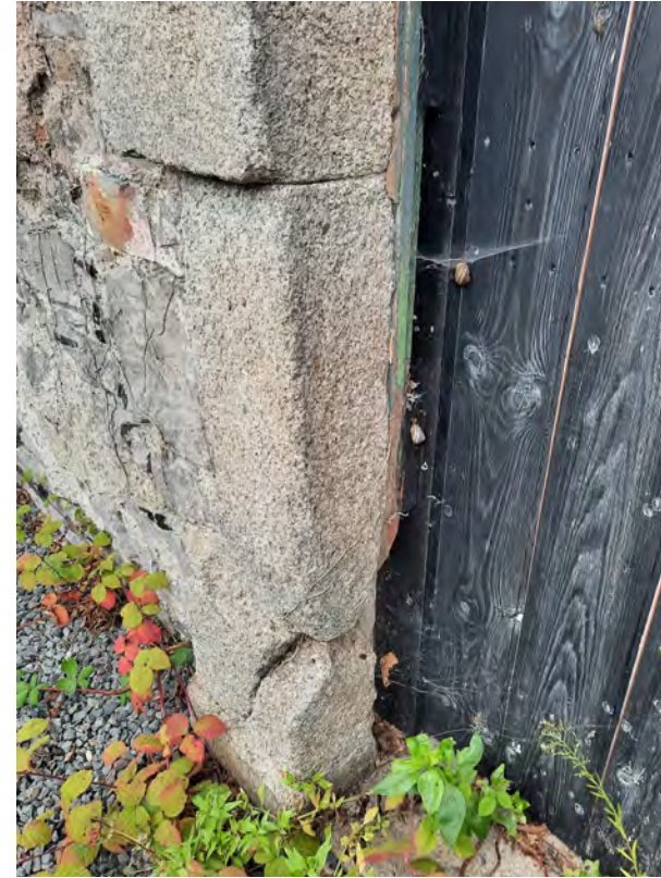
Damage to stone doorway surround at entrance to 2.6
