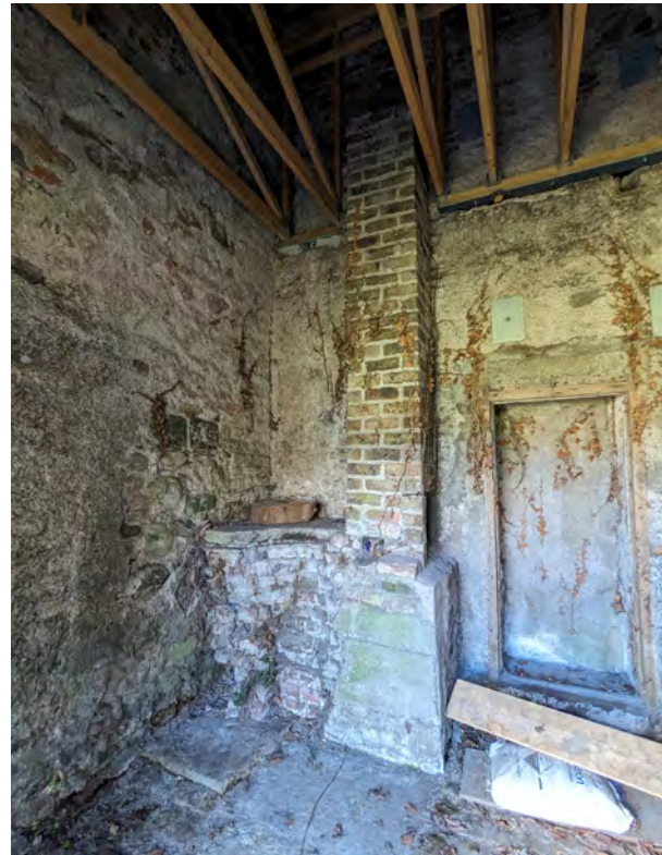
Chimney Stack with widened base, resembling construction of a forge.
