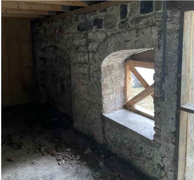
Partially demolished vaulted opening, modified cill height.
