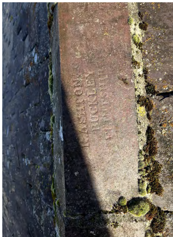
Clay ridge tiles marked with the makers mark 'R. ASHTON & Co BUCKLEY FLINTSHIRE'
