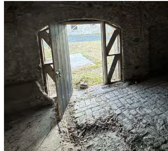
Archway fitted with timber bracing and door.
