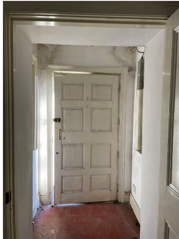
Porch leading to entrance hallway. Damp staining visible above doorway at north and south corners of the western wall.
