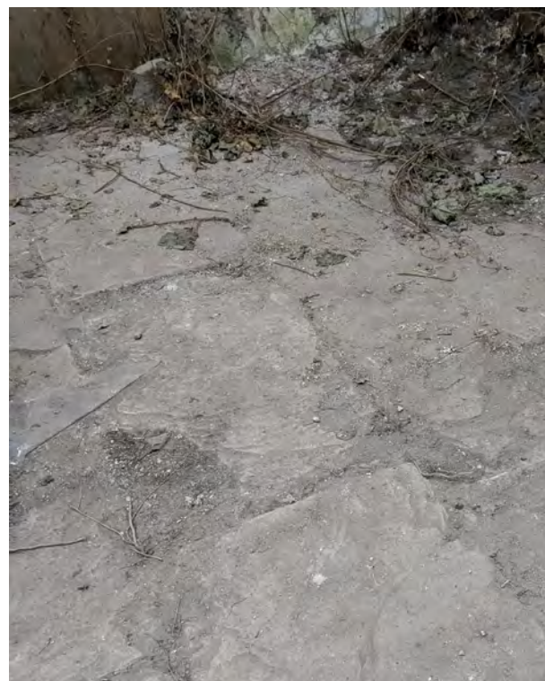
Limestone flag floor to room 2.4. Flags are uneven and damaged in places.
