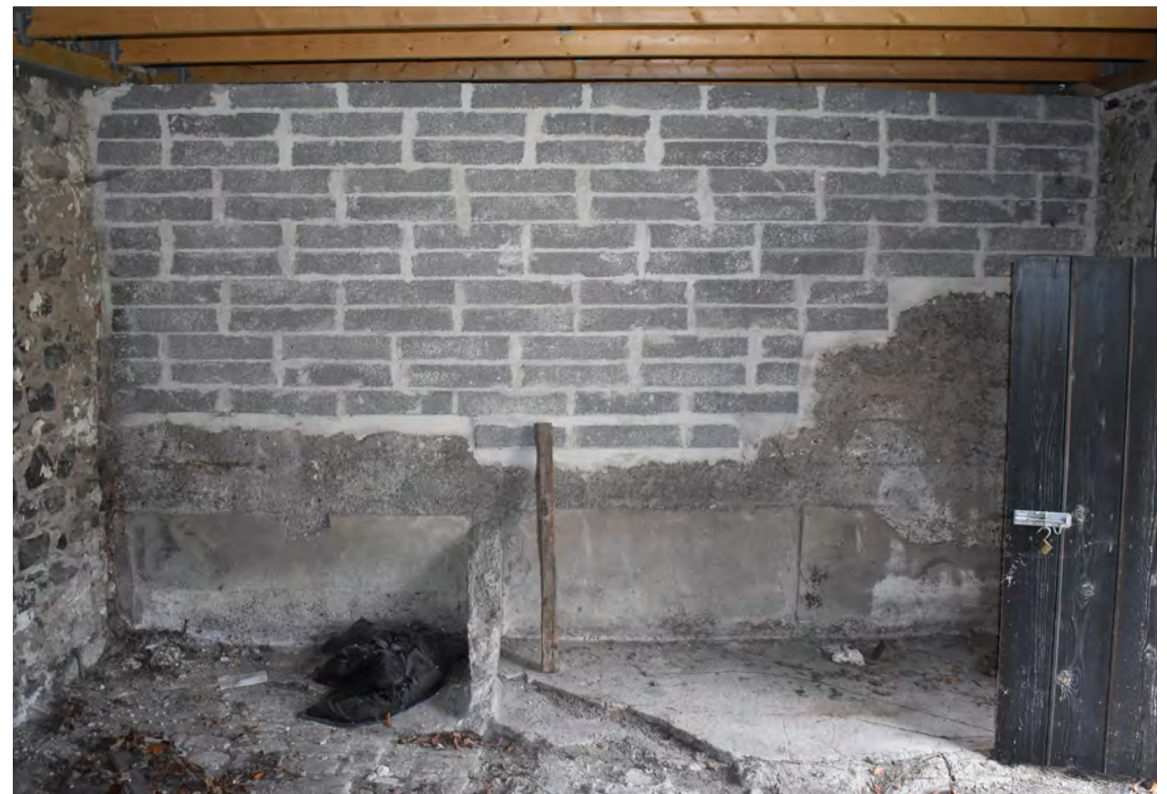
Dividing wall between west and north ranges. Remains of cattle stalls visible at base of the wall which has been built up to the base of the timber roof structure using concrete blocks.
