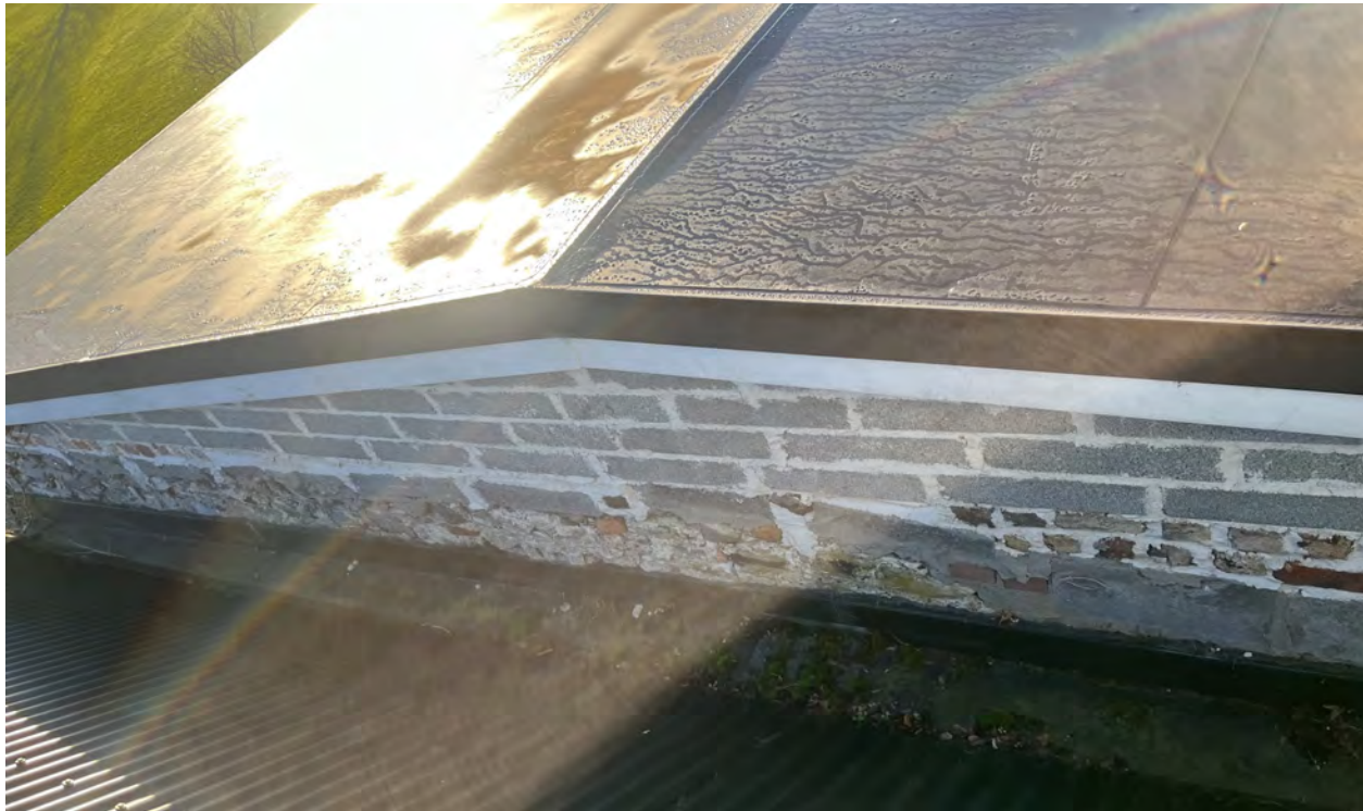
Unrendered blockwork built upon existing brick / stone wall, form gable end of pitched roof.
