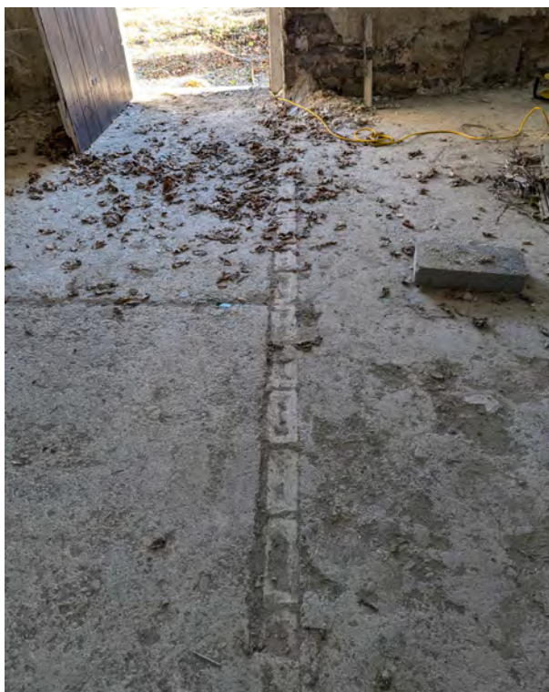
Concrete floor with brick channel detail (Room 2.1)
