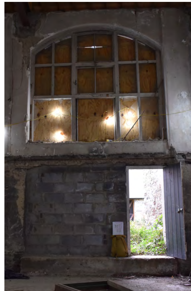
Ope 14 - (A) Multi-pane timber casement window, pivot-hinged opening sections. Some broken opaque glass remains. (B) Timber panelled door & frame provides access. Remaining ope infilled with blockwork.
