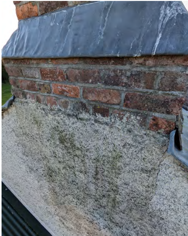
Plasterwork of the northern gable wall discoloured due to damp staining beneath the chimney stack.
