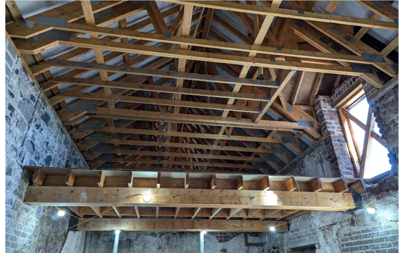
Recently installed timber Mezzanine / Loft floor construction and timber trussed rafters to roof. Recently rebuilt and repointed brickwork to top of dormer window.
