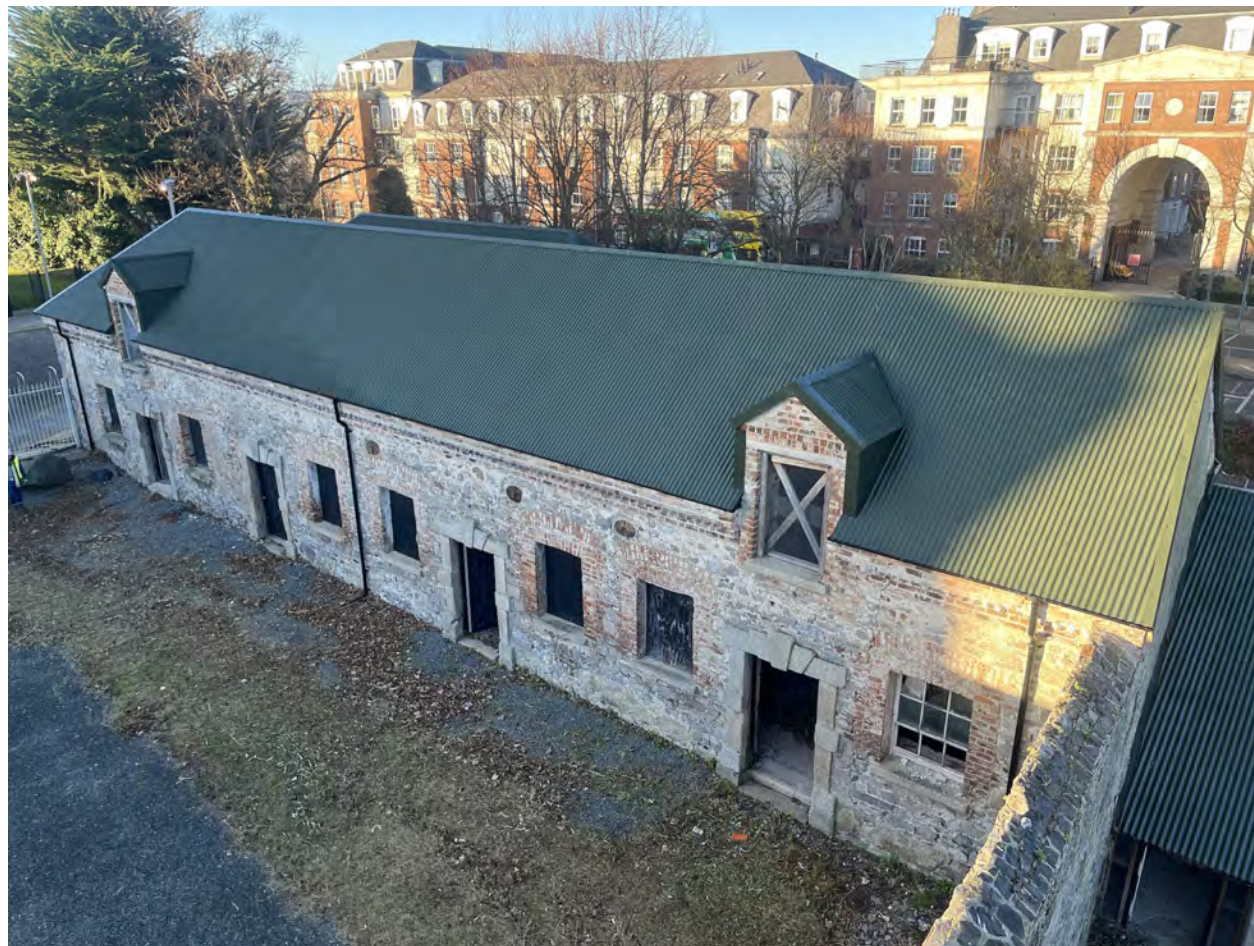
East Facade of Building 2, as seen from above, calp stone construction and brick detailing. The building has one of the more
