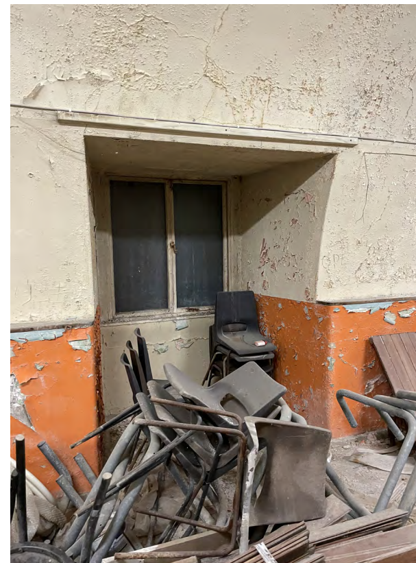
Ope 8: Timber framed window, opaque glass.
