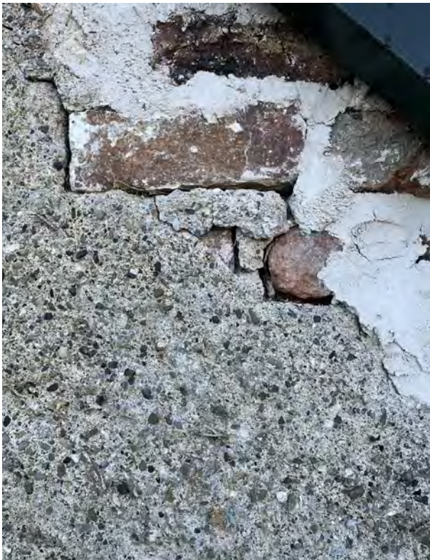
Loose bonding of brickwork to top of gable wall (north).
