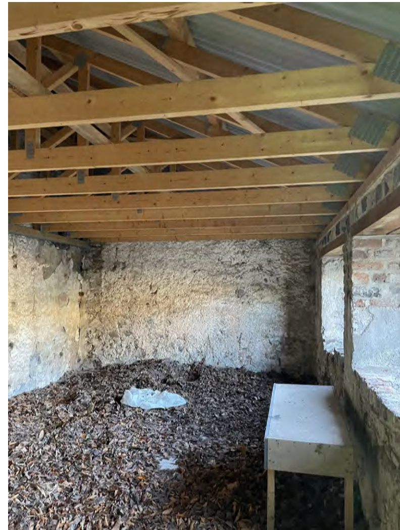
Interior, Room 4.1. Leaf fall has built up internally entering through open doorway.
