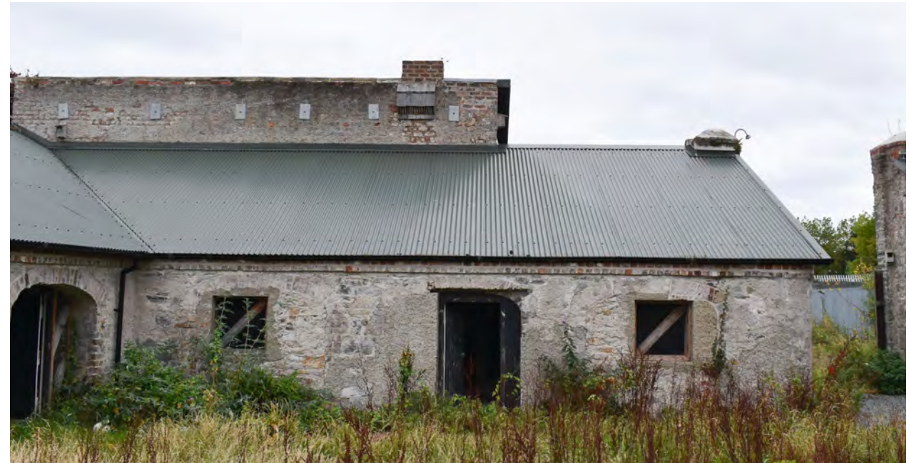
North range. The three archways have been modified, with a doorway inserted into one half of the central archway flanked by rectangular windows.
