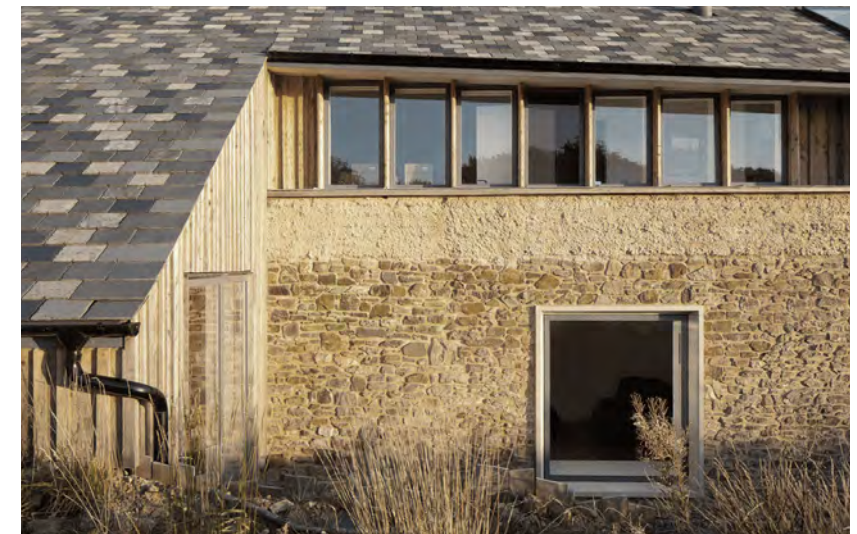
Figure 77 - Rough cast render finish to new build elements over existing wall with long window and new punched openings, Bude Barn by Fielden Fowles Architects
