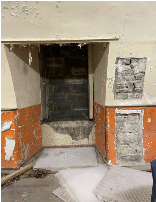
Ope 2 Exposed blockwork to former window ope in eastern wall.
