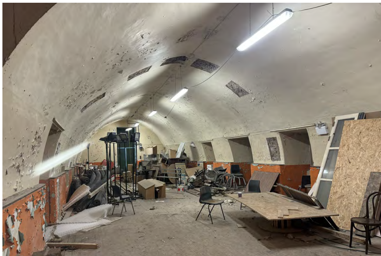
Barrel vaulted ceiling to interior of Cromwell's Fort, looking south.
