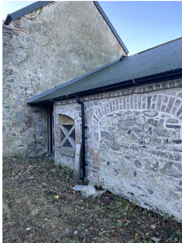
Partially demolished archway and adjacent blind archway situated to the southern end of the west range.
