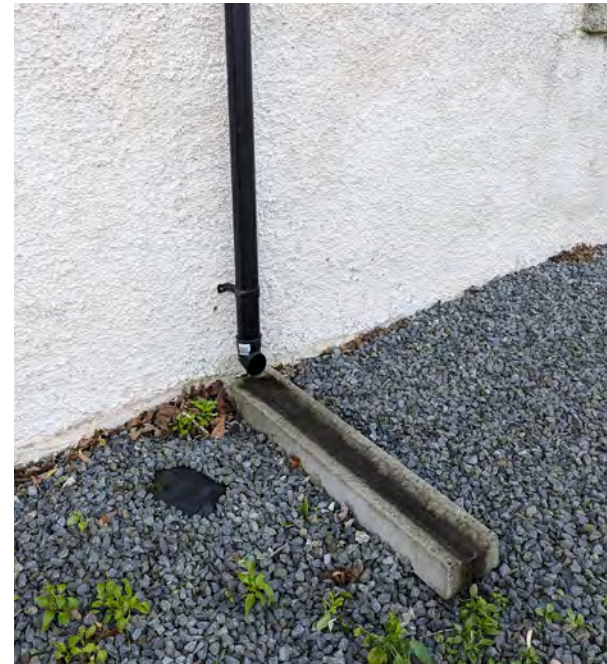
Downpipe discharging directly on to concrete channel piece perpendicular to wall.
