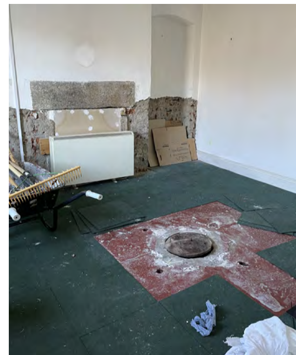
Ground floor room to the north. approx. 1m of internal plaster to the north facing external wall has been removed above finished floor level.
