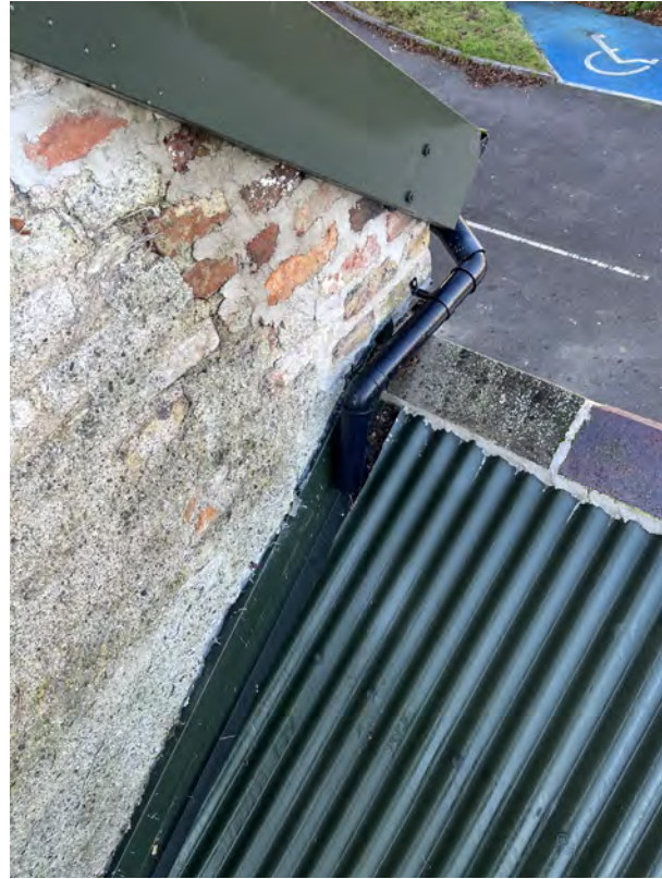
Downpipe discharging from Building 2 on to roof of Building 6
