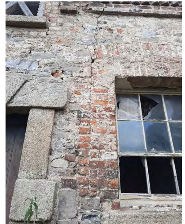
Crack in east facade between door and window at the north end of the facade. Damage to brick cornice.
