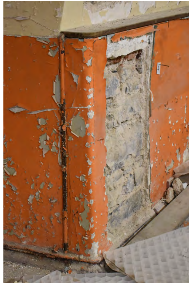
Wall projection approx 1m high at base of eastern and western walls.
