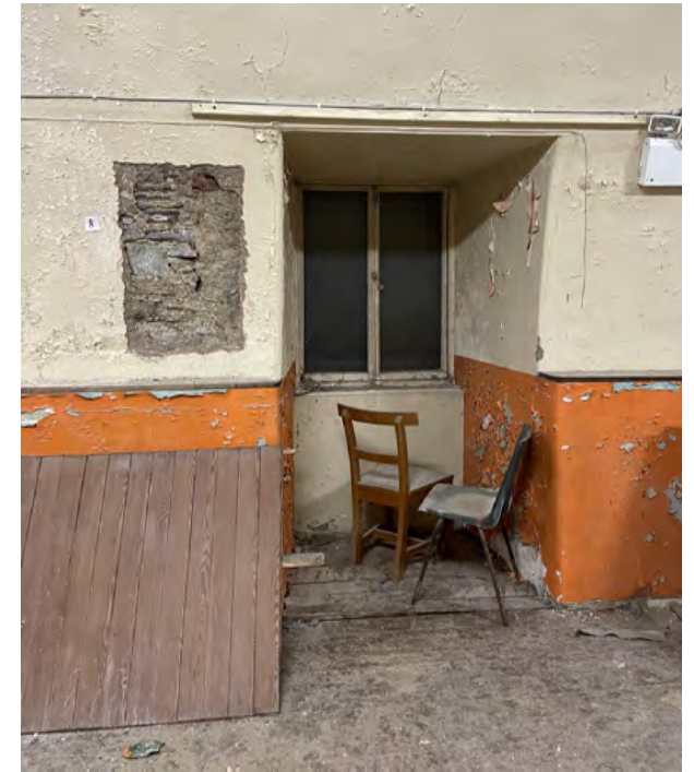
Ope 9: Timber framed window, opaque glass.
