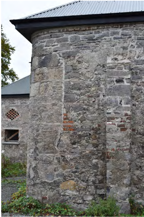
Western gable wall, rounded corner and remains of buttress.
