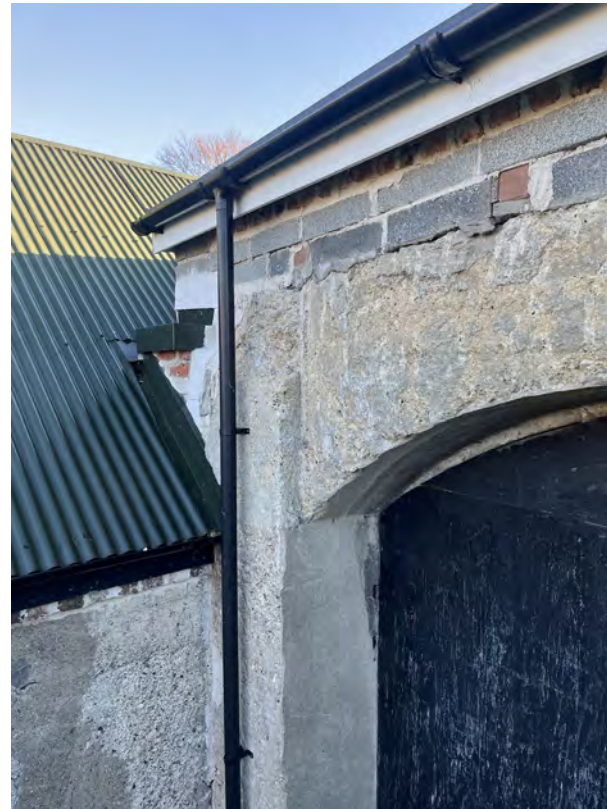
Unrendered blockwork built above existing brick & stone walls at North-West entrance.
