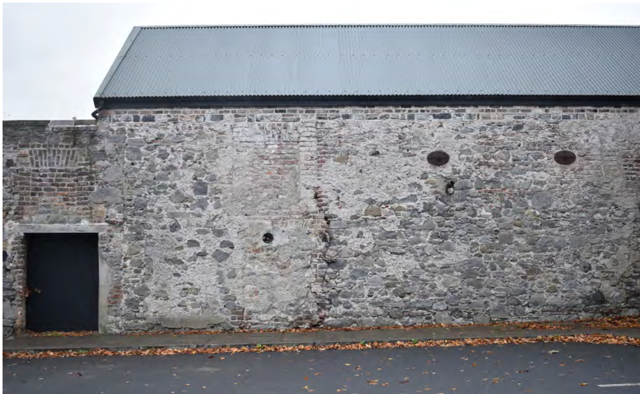
East Range, West Elevation, View from Rathfarnham Road Car Park. Remnants of lime plaster visible. Former window openings infilled with brickwork are visible where plaster has decayed.
