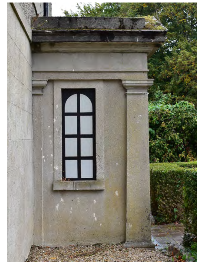
Window opening to the south facing side wall of the porch. Both windows to the north and south have been covered with a painted timber panel.
