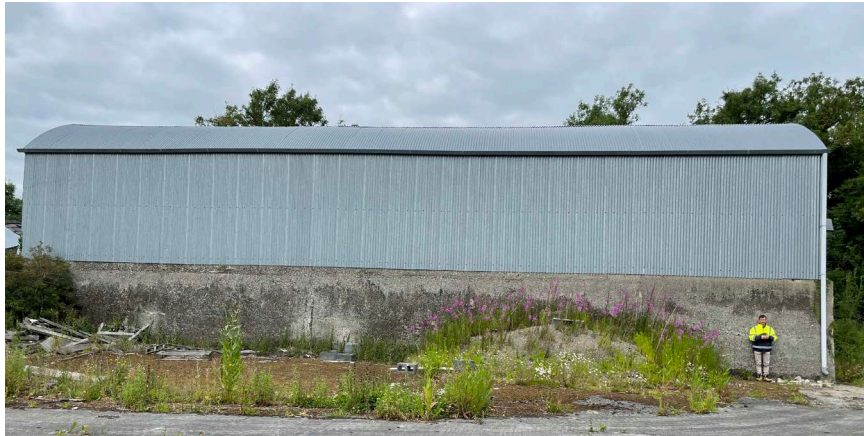
C6 Metal Shed - Current state photos
