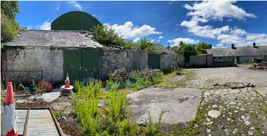
C7 Grange Cottage Outbuilding 04 - Current state photos
