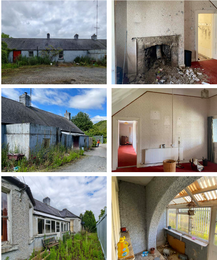
C1 Grange Cottage - Current state photos
