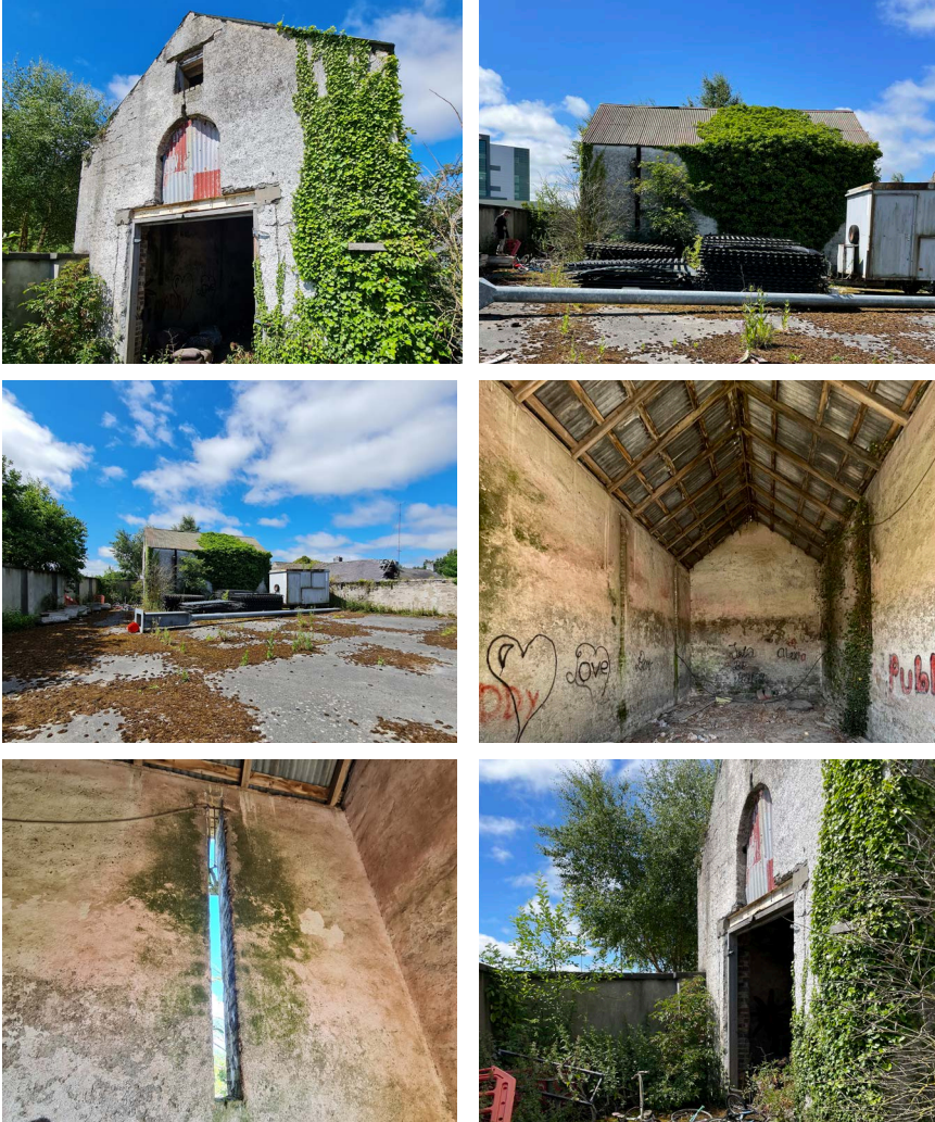
C5 Concrete Barn - Current state photos
