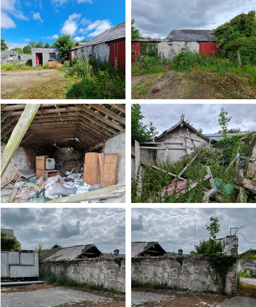
C2 Grange Cottage Outbuilding 01- Current state photos
