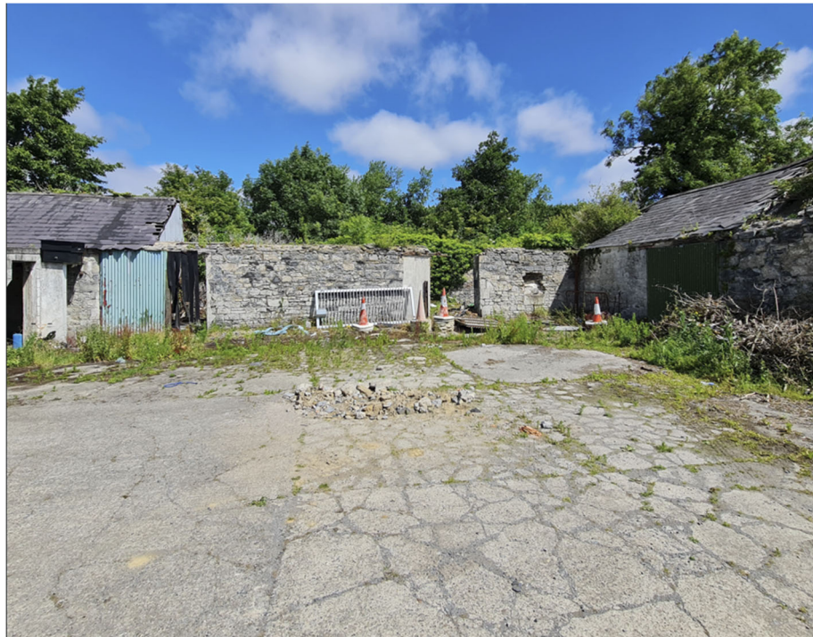
Existing Outbuildings (C4&C7)
