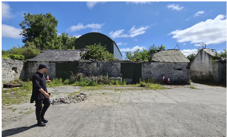
Existing View of Main Courtyard
