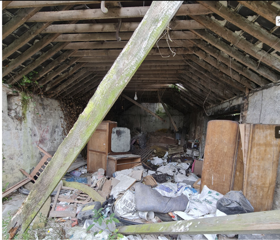
Existing Outbuilding (C2)
