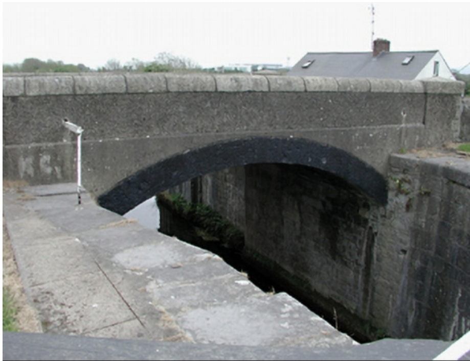
Fig. 2: Image of existing masonry bridge. Source: National Inventory of Architectural Heritage.
