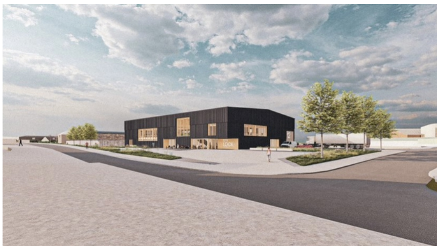
Fig. 13: Computer generated image of the north and east elevations showing new proposals for building B03. Source: Stephen Foley Architects
