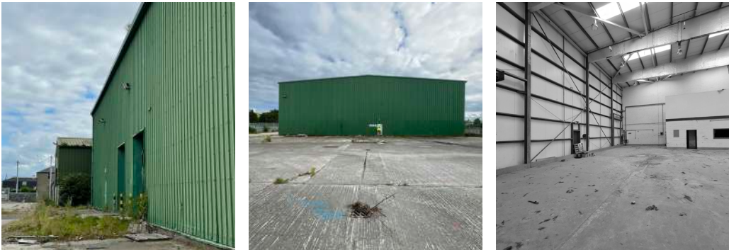
Existing Building Conditions
