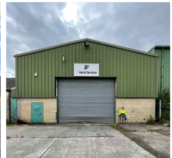
Existing industrial shed 02 to be demolished
