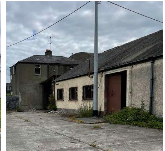
Existing industrial shed 01 to be demolished
