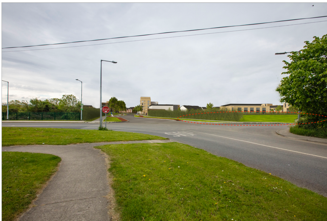
Figure 1: Extract from Proposed View 2 of the Photomontages prepared as part of ABP Ref. ABP-305267-19, as amended with subject site indicated with red dashed line (Overlay by SLA).
