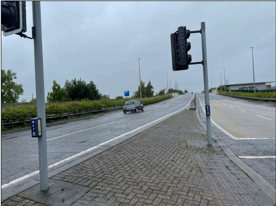
Plate 2-1 View from the south of the existing R136 carriageway with crash barriers, hazel hedgerows and fencing visible within the development site boundary.
