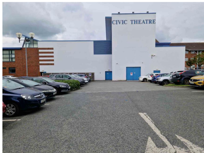
Existing site, directly adjacent to the existing Civic Theatre, looking west.
