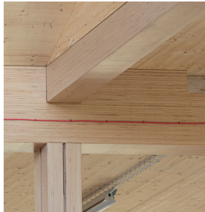
LVL exposed structure: Vistoe, Waugh Thistleton.
