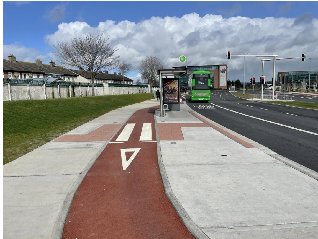
Figure 17: Example of inline bus stop island, Liffey Valley
