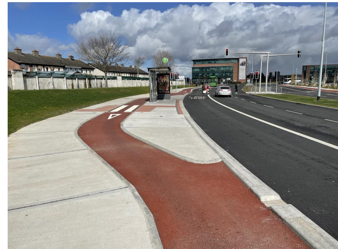
Figure 16: Example of inline bus stop island, Liffey Valley
