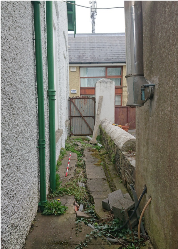
Footpath at rear of courthouse showing break with ceramic pipes and outbuilding to be demolished at right
