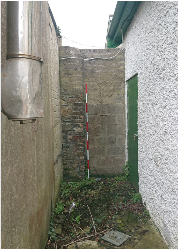
Eastern side of courtyard wall, lined in brick and extended with concrete blocks; showing also boiler house on right and outbuildings on left
