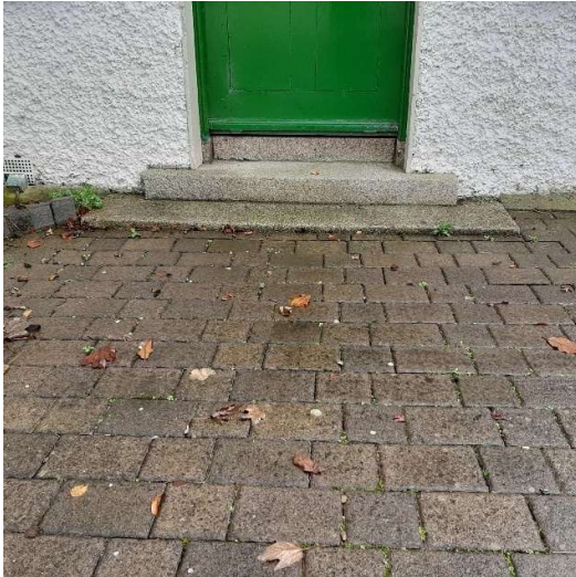
Left side: The lower granite step at the entrance to the former judge's robing room has been partly buried beneath the modern pavement. Right side: A view of the former judge's robing room.
