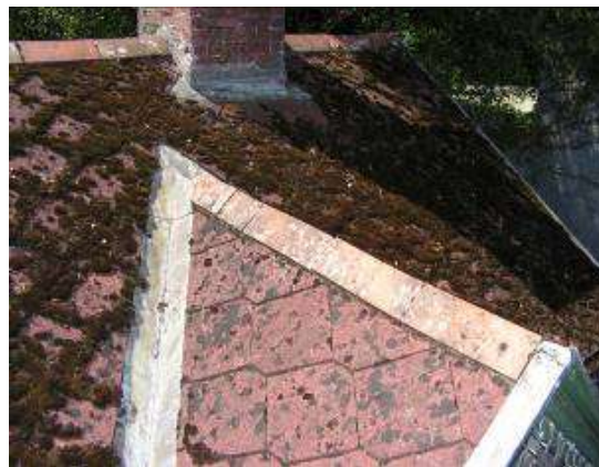
Left side: The chimney above the robing room and part of the southern roof pitch of the smaller roof. Note the eroded mortar joints in the bricks and under the ridge tiles. Right side: The northern pitch of
