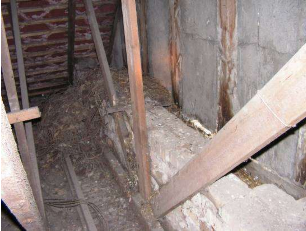
A view of the north end of the attic above the court room. Note the King Post roof truss and the inner surface of the gable to Main Street, the remains of the lime parging mortar on the undersides of the tiles, the original plaster-on-lathe of the cornice (behind the parapet wall) and the modern plasterboard of the main ceiling to the left of it. The debris in the far corner is the remains of a bird's nest
