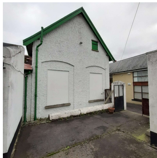
Left side: A blocked and overflowing rainwater gully. Right side: The two former window openings in the rere façade which were blocked up.
