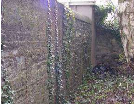
Left side: A part of the old western calp limestone boundary which is being colonised by ivy. Right side: The same wall viewed from the yard side where it has been rendered with sand and cement.
