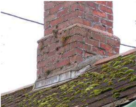
Left side: The chimney above the robing room and part of the southern roof pitch of the smaller roof. Note the eroded mortar joints in the bricks and under the ridge tiles. Right side: The northern pitch of
