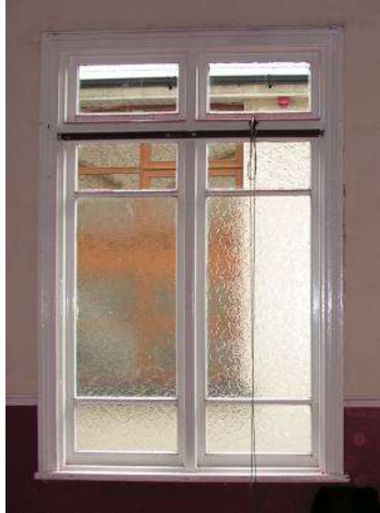
Left side: The casement window in the north-west part of the courtroom. Right side: The inside of the window in the south-east part of the courtroom. Note the cord which operated the upper vent lights
