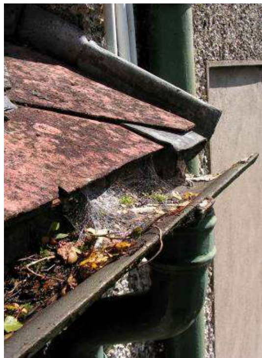
Left side: The cast iron fireplace in the former judge's robing room. Right side: A close up view of one of the asbestos cement tiles and debris-filled cast iron gutters.
