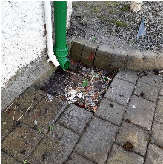
Left side: A blocked and overflowing rainwater gully. Right side: The two former window openings in the rere façade which were blocked up.
