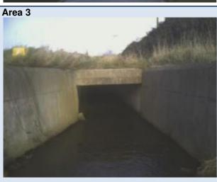
The culvert leaving Mount Argos Park at Kimmage Road Lower has been identified as at risk of blocking and causing significant increased flood risk. Debris has been found in the watercourse upstream of Mount Argos Park at Mount Argos Way which potentially may contribute to the culvert blockage risk/
