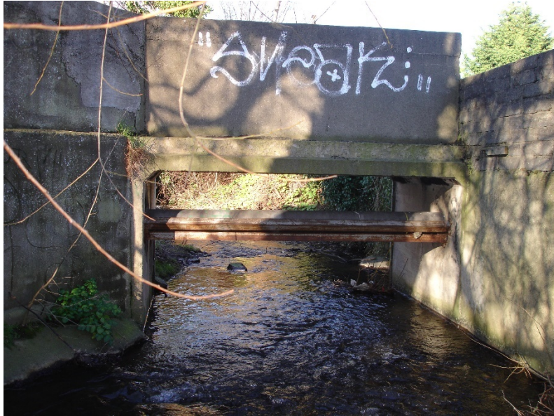
Figure 3-6: 225mm diameter Concrete Stormwater Pipe under the Foot Bridge
