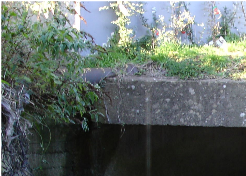
Figure 3-17: 14" dia. Cast-Iron above Twin Culvert Inlet
