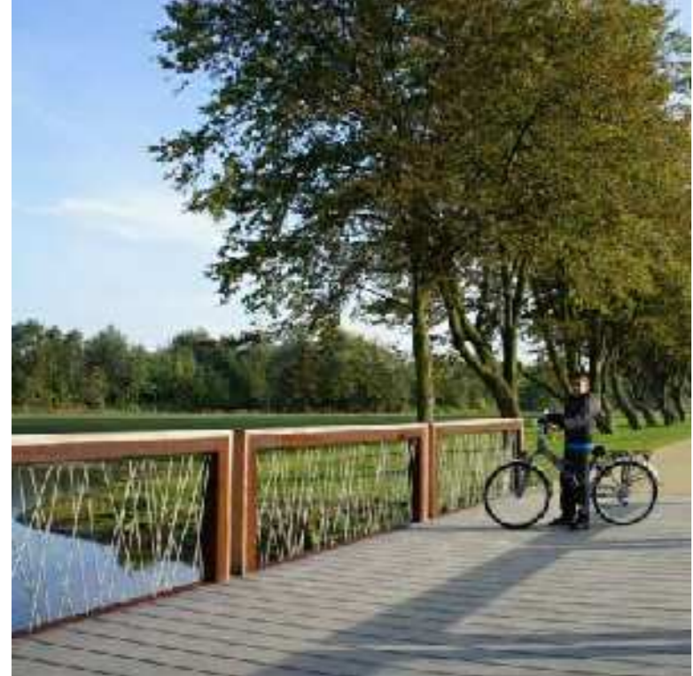
Pedestrian Bridge in Corten Steel & Composite Decking
