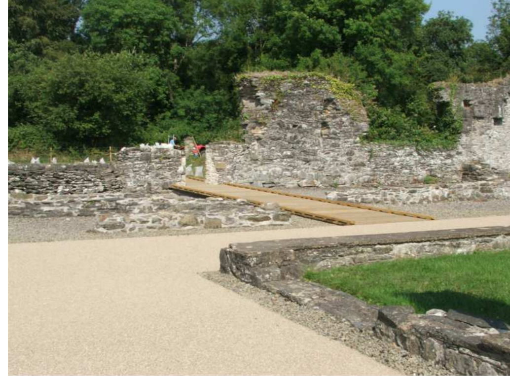
Resin Bonded Gravel
