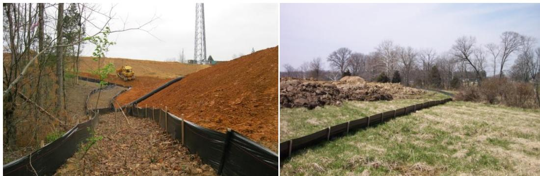
**Plates 1 & 2: Typical Silt Fence Usage**
