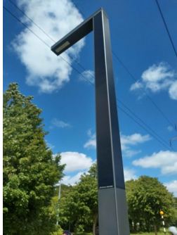
Image of Solar powered street light
