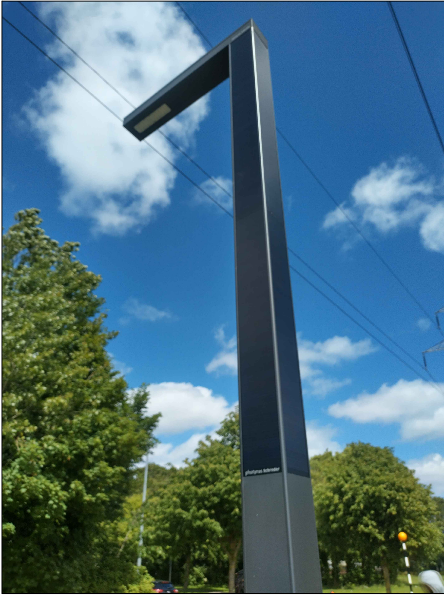
Solar powered street light Shreider Verticalis
