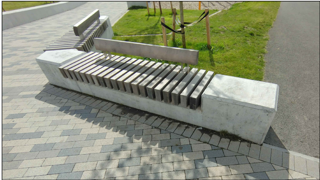
Cast in situ concrete with Streetlife timber seating
