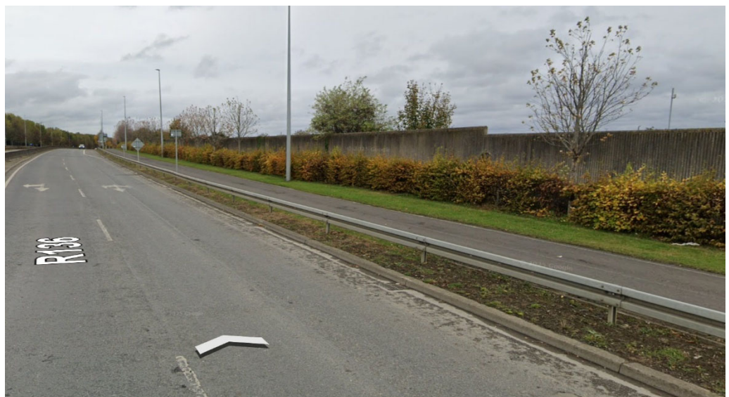
View of the west of the site looking North. Wall and screen to Grange castle Road /R136 can be seen to the right. Proposed location of new entrance road (Image courtesy of Google Maps)
