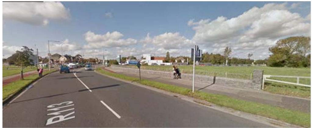
Entrance to site / Killinenny Road
