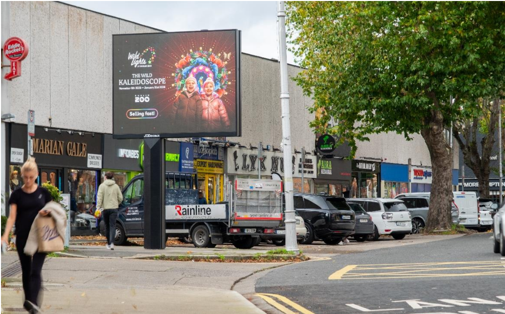
Figure 5 Image of Digipole installed in Donnybrook, Dublin 4
