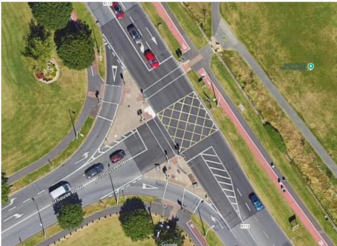
Figure 3: Aerial view of Firhouse Road West Junction
