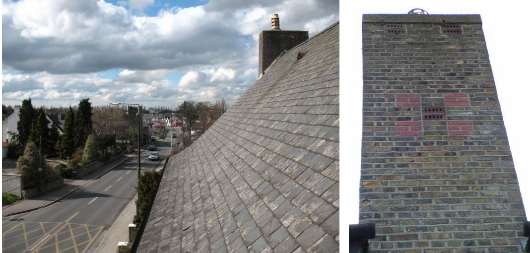
A view of the roof & northern chimney. Note the decorative pattern and the bright coloured patches of recently spalled brickwork.
