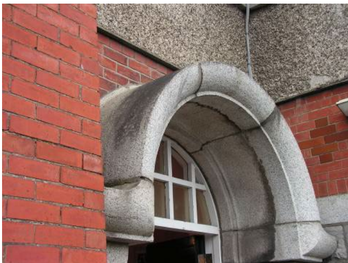
The granite hood over the entrance. Note the different texture, colour and finishing profile of the OPC binder mortar in the joints between the bricks in this area and the lime bonder mortar elsewhere. the fire exit.
