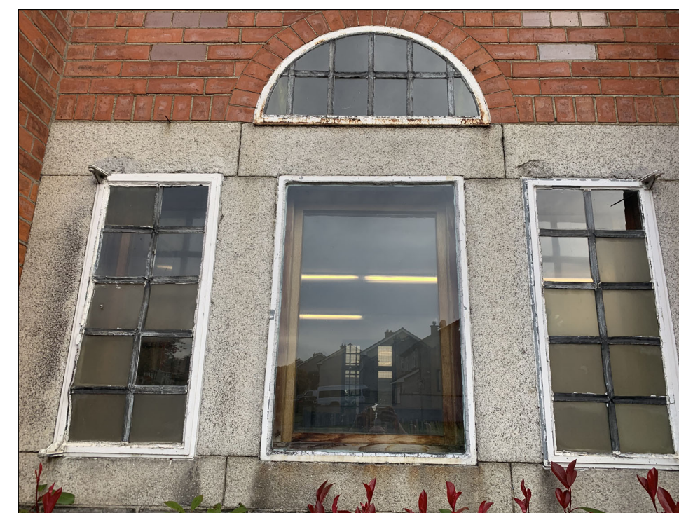
EXISTING GROUND FLOOR WINDOWS (with perspex outerframe)
