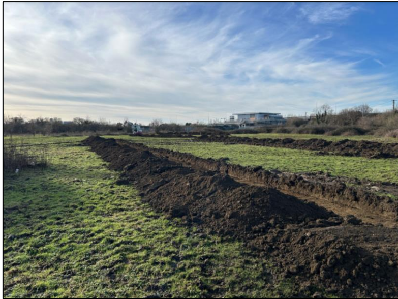
Plate 1: Looking southwest at the site during testing
