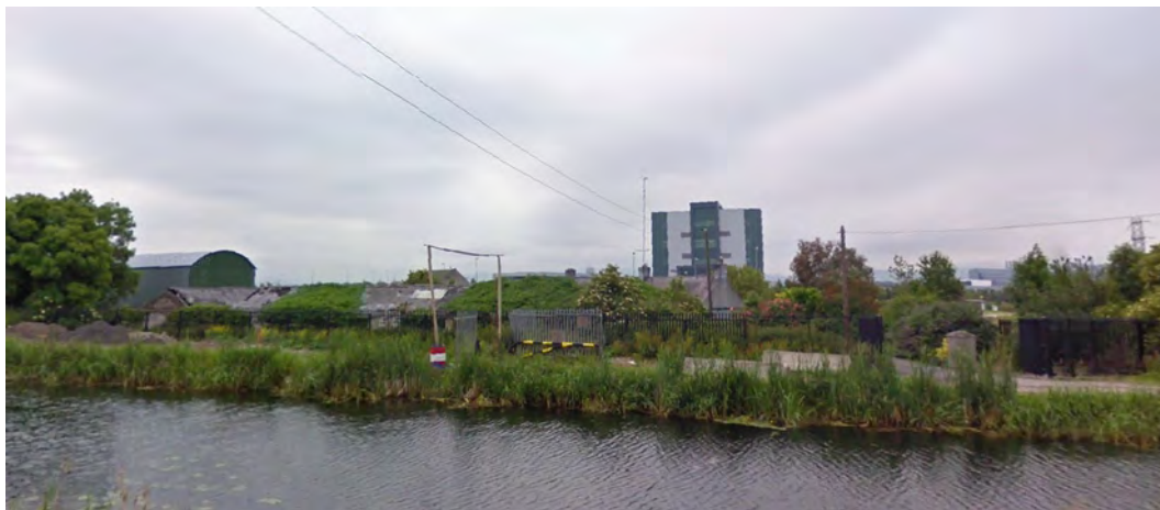
Plate 16: Clockwise from Top left: General views of existing site arrangements - East entrance gates, boundary wall at outbuilding C5, Grange Cottage courtyard, northern boundary arrangement and canal path, and existing east courtyard arrangement.
