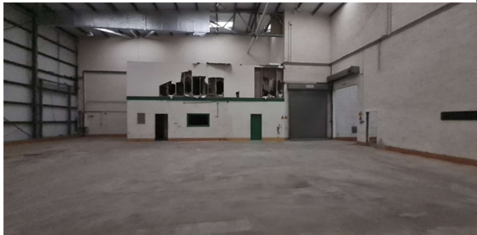
Interior of Existing Industrial Unit 03 to be retained and modified.
