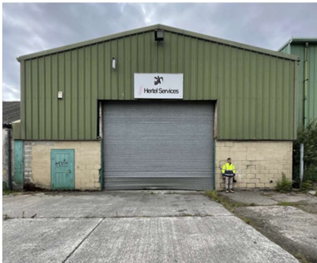
Existing Industrial Building (02) to be removed.
