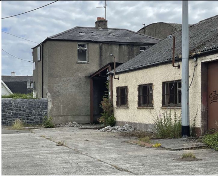
Existing Industrial Building (01) to be removed.
