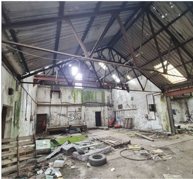
Interior of existing Industrial Building (01) to be removed.
