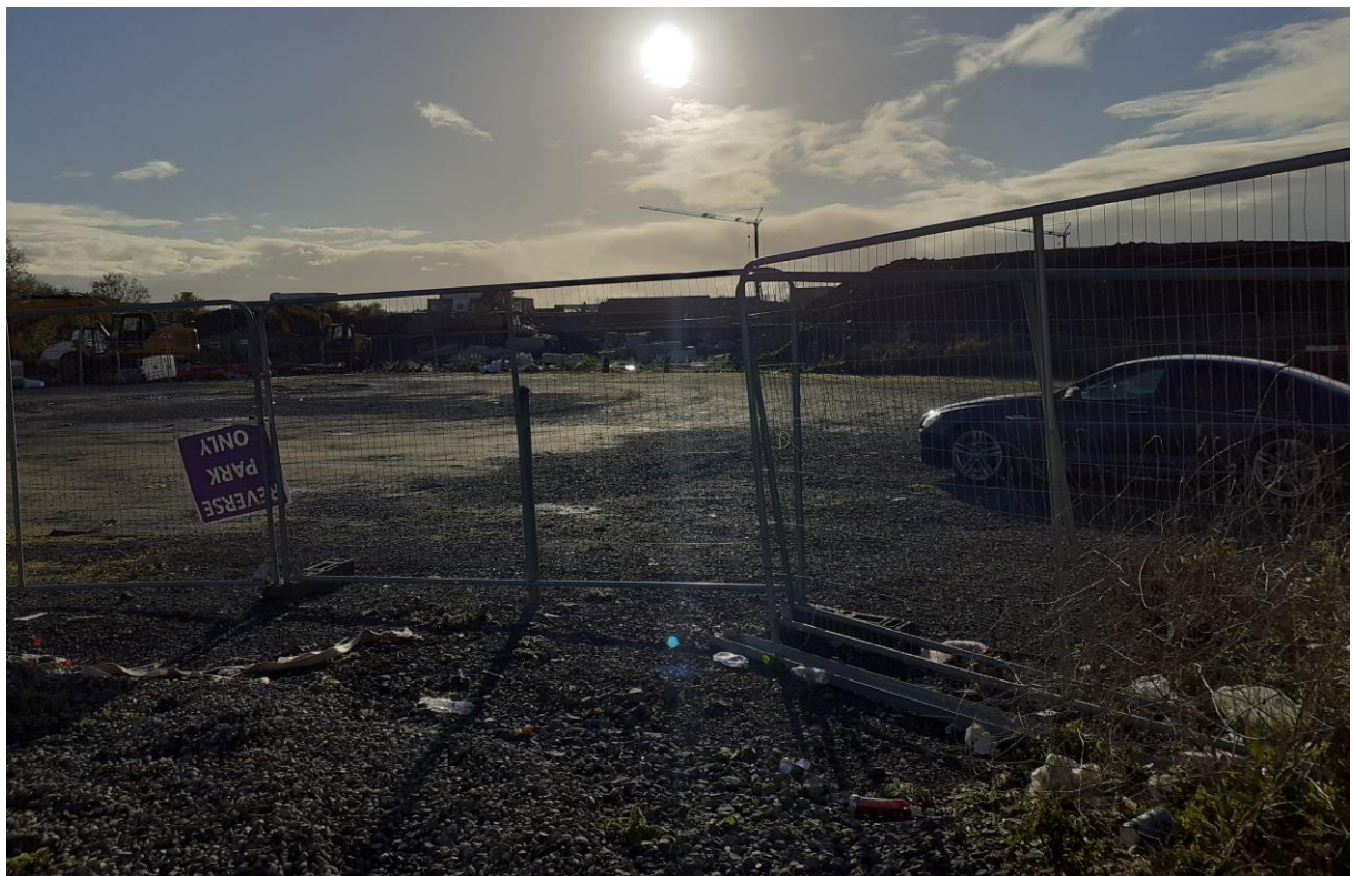
Figure 4-6: The construction area of the site, as seen from the north-east corner of the boundary
