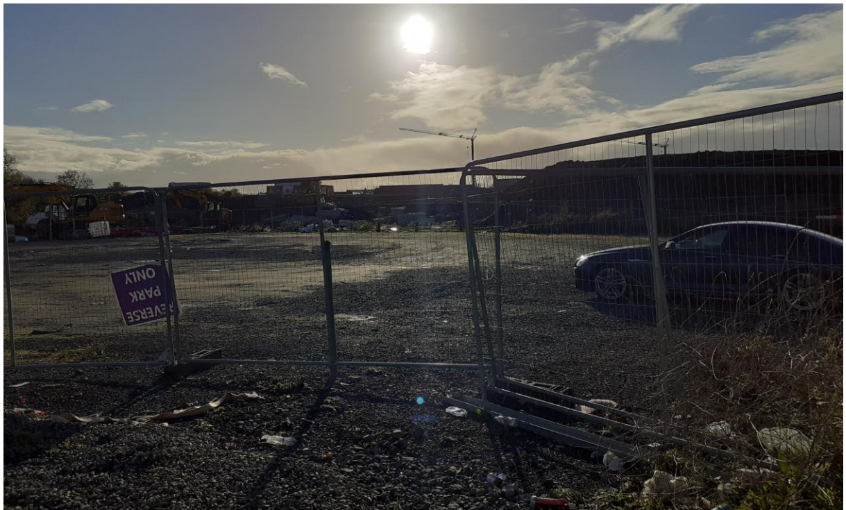
Figure 3-3: The construction area of the site, as seen from the north-east corner of the boundary.
