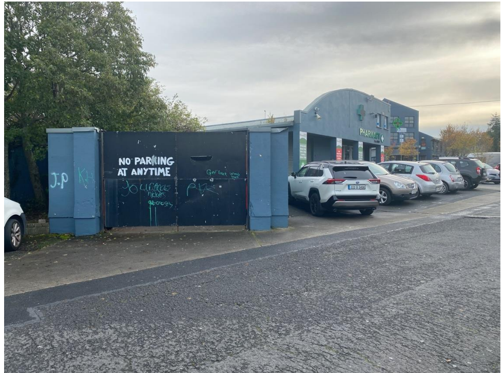
Existing Bin Store – View Towards Brookfield Enterprise Centre (PKA)
